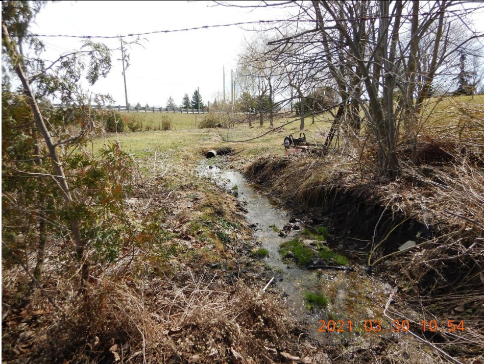
HDF 8a-2 is located on a non-participating property. Photograph taken from property line, facing downstream. Photograph for information purposes only.
