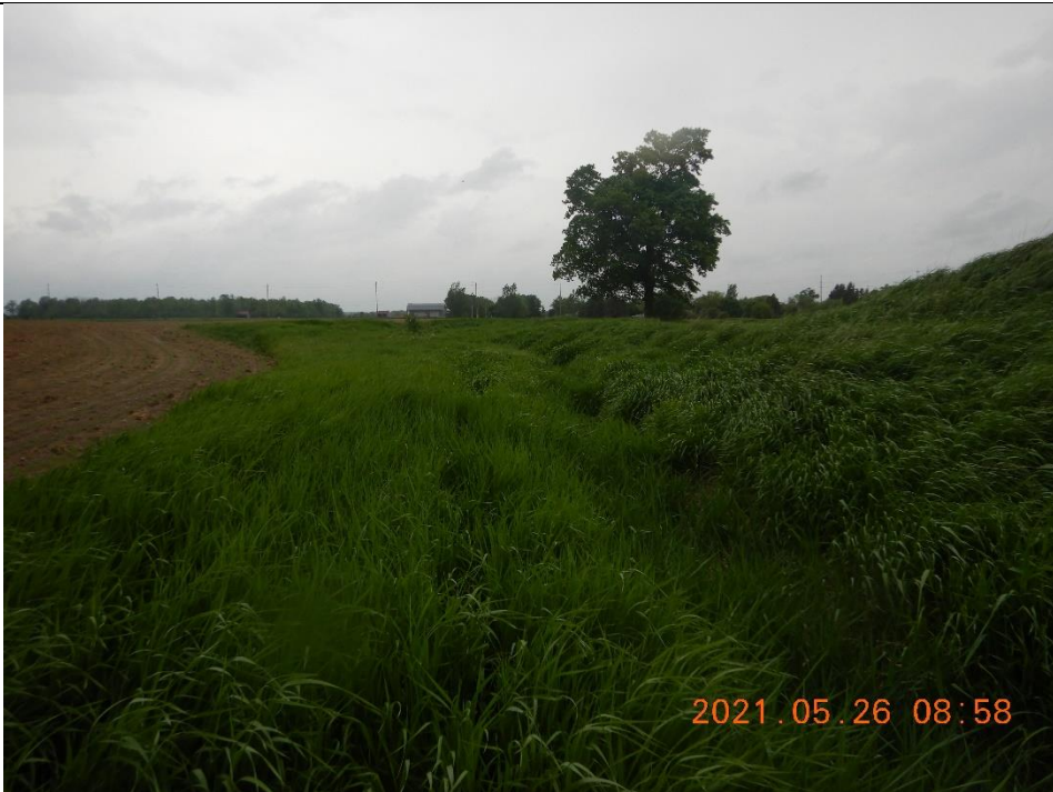
HDF 8a-4 was observed to be dry at the time of the second round of observations. Swale feature with no defined, single channel.
