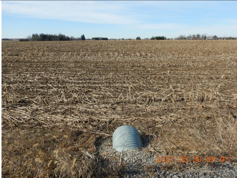
Photograph taken looking downstream, HDF 3 was not observed in situ.
