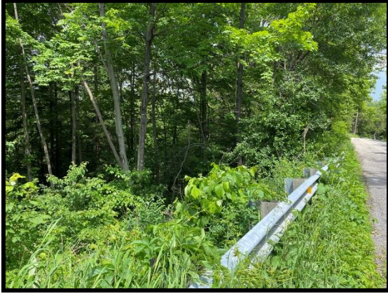
Image 11: Sloped Lands (June 16, 2022; Facing Northeast)
