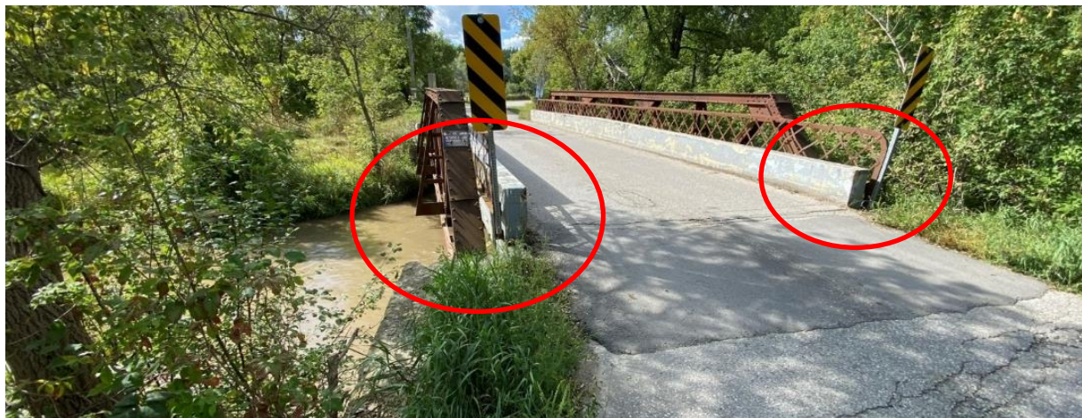
Figure 3: Transition between Roadway and Bridge
