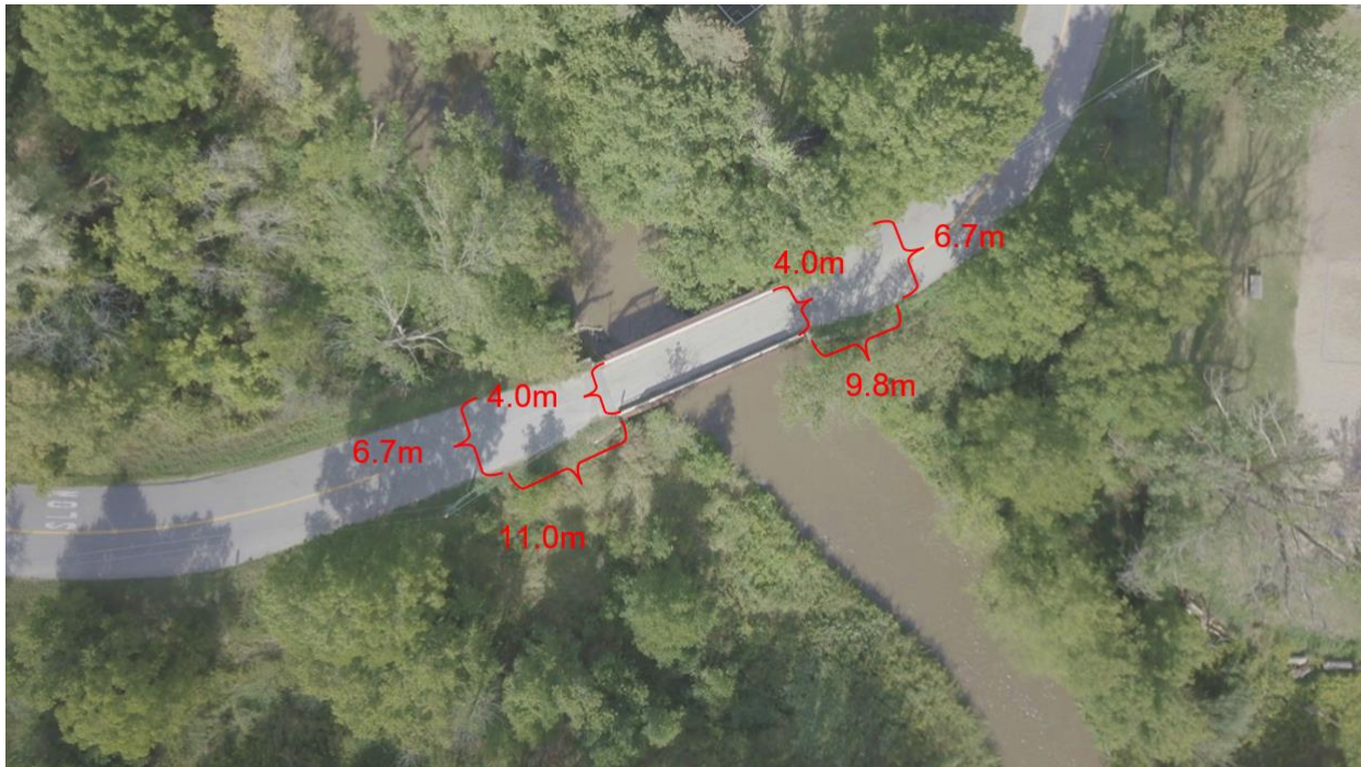
Figure 2: Pavement Width and Pavement Marking at the Bridge
