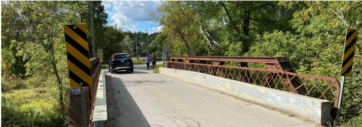
Figure 11: Pedestrians and Vehicle Sharing the Bridge
