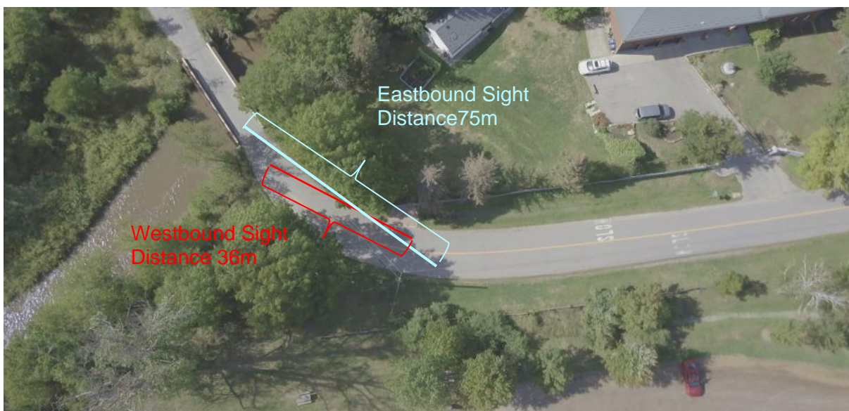
Figure 4: Sight distance at the Bridge
