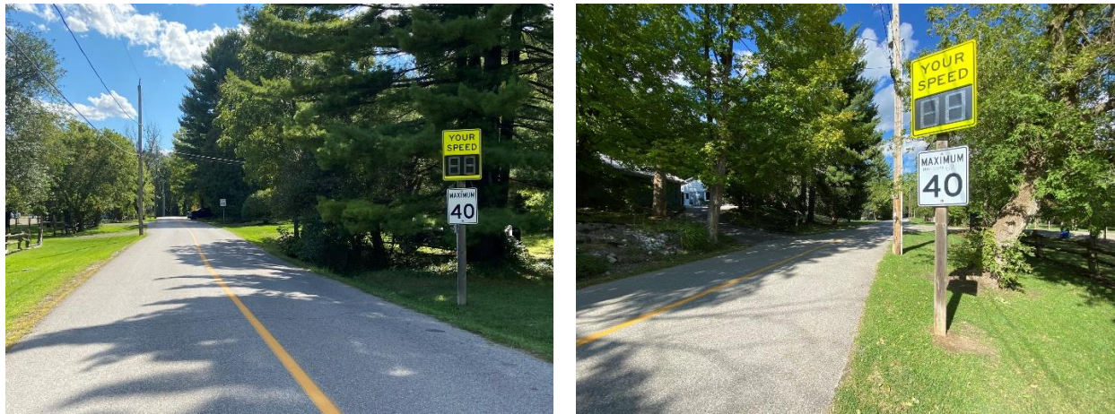
Figure 8: Digital Speed Signs Close to the Bridge
