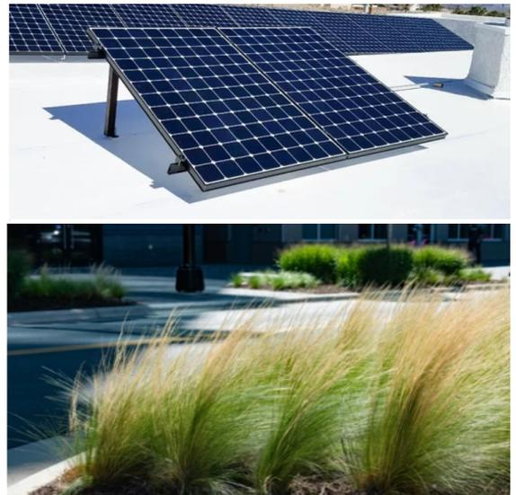
QuadReal is part of the LEED 4.1 Volume Program and is standardizing sustainable features in its developments. Roofs are designed with low-albedo white-coloured membranes. The buildings at 12668 Dixie Road are designed to be “solar ready” with roofs designed to support Photovoltaic panels and additional room in the electrical rooms to accommodate solar equipment.
