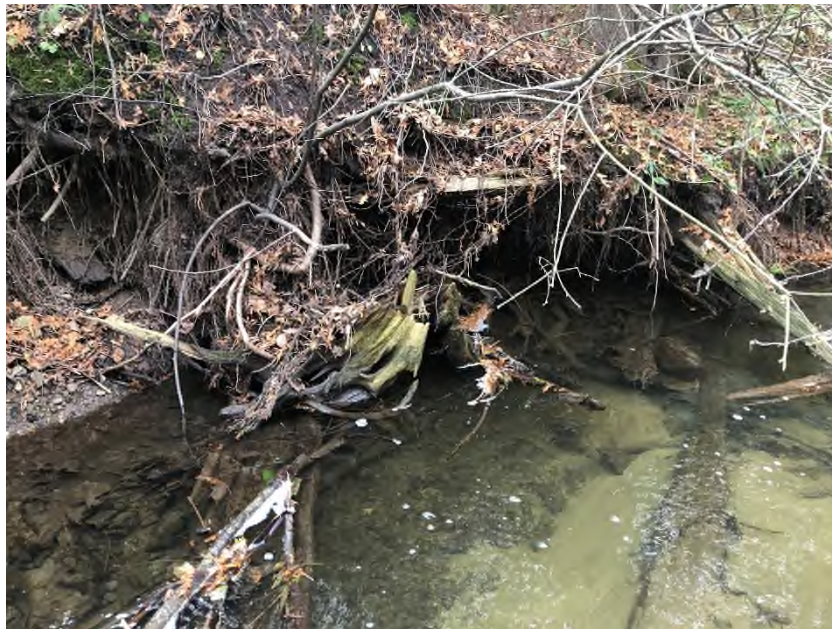
Photo 2: Facing north, an undercut section of the bank with large woody debris within it (10-30-2020).
