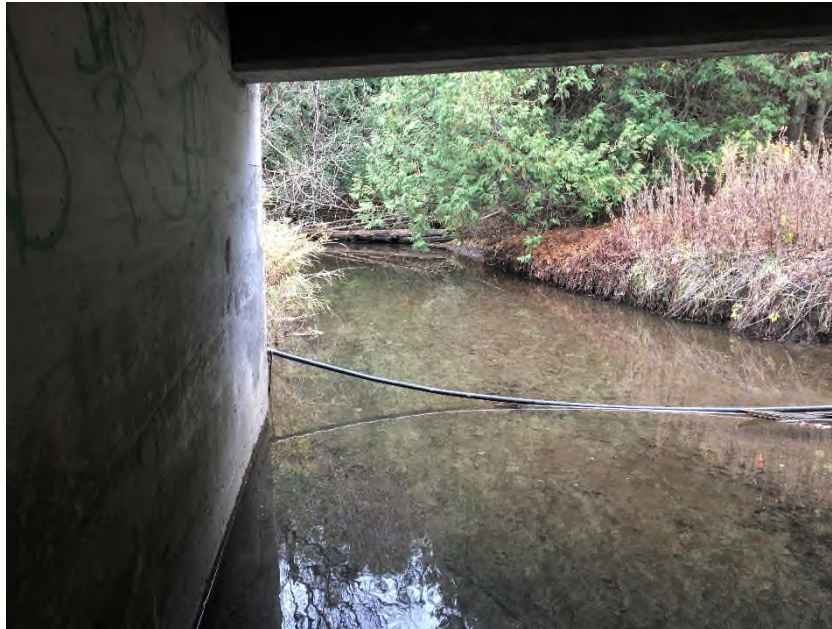
Photo 4: Facing south, the watercourse downstream of PSR-1 (10-30-2020).
