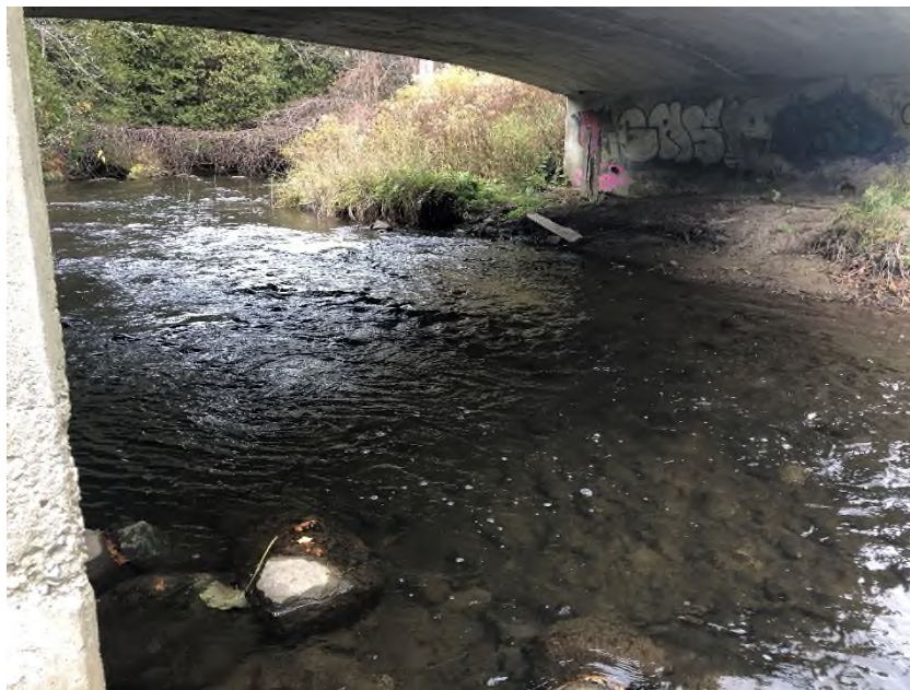
Photo 8: Facing north, the watercourse flowing through the PSR-2 bridge (10-30-2020).
