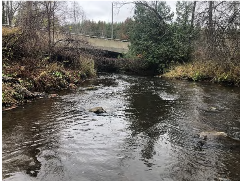
Photo 7: Facing south, the watercourse flowing toward PSR-2 (10-30-2020).
