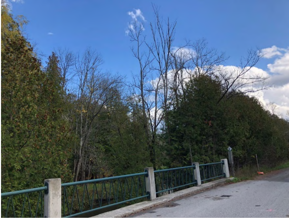
Photo 5: FOMM4-2 - As viewed from Duffy's Lane Bridge looking southeast (September 30, 2020)
