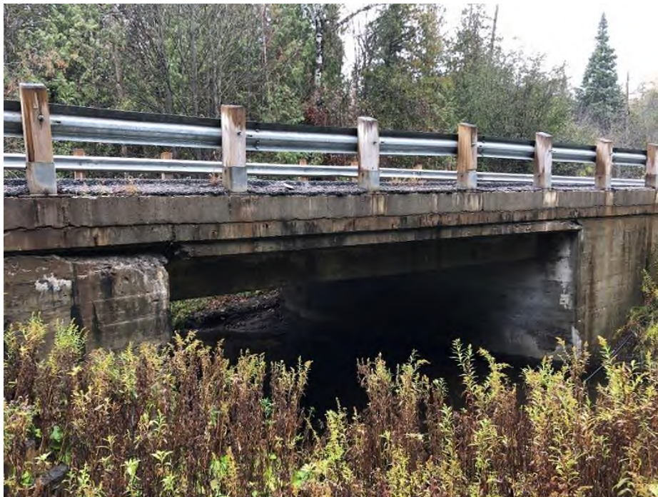
Figure 3: Patterson Side Road Bridge No. 1 (ASI 2020)
