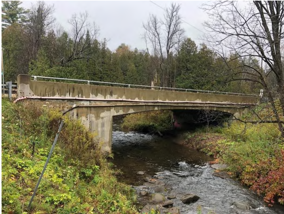
Figure 4: Patterson Side Road Bridge No. 2 (ASI 2020)
