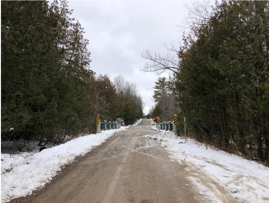
Plate 25: Southeastern approach, looking northwest towards Duffy's Lane Bridge
