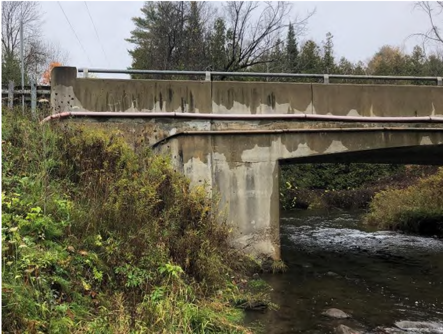
Plate 20: View west, of the southeast elevation of the south abutment.
