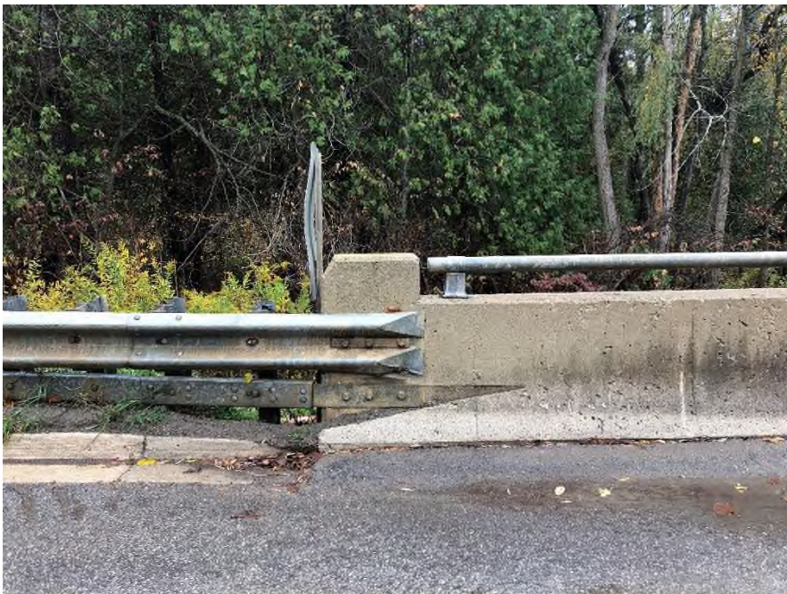
Plate 19: Detail of guard rail, as well as concrete parapet and steel rail barrier system.
