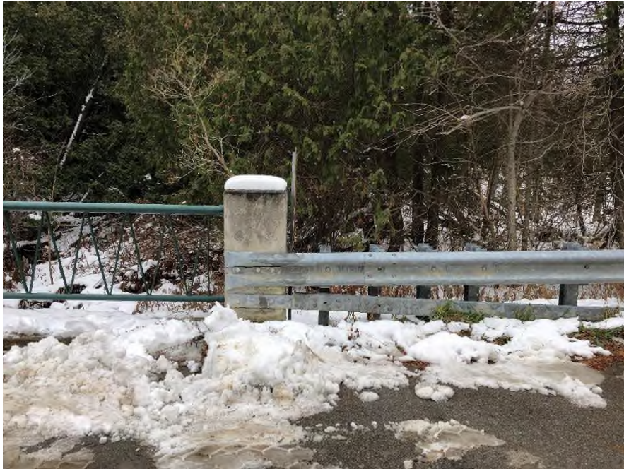
Plate 31: Detail of guard rail, as well as cement post and steel rail barrier system.
