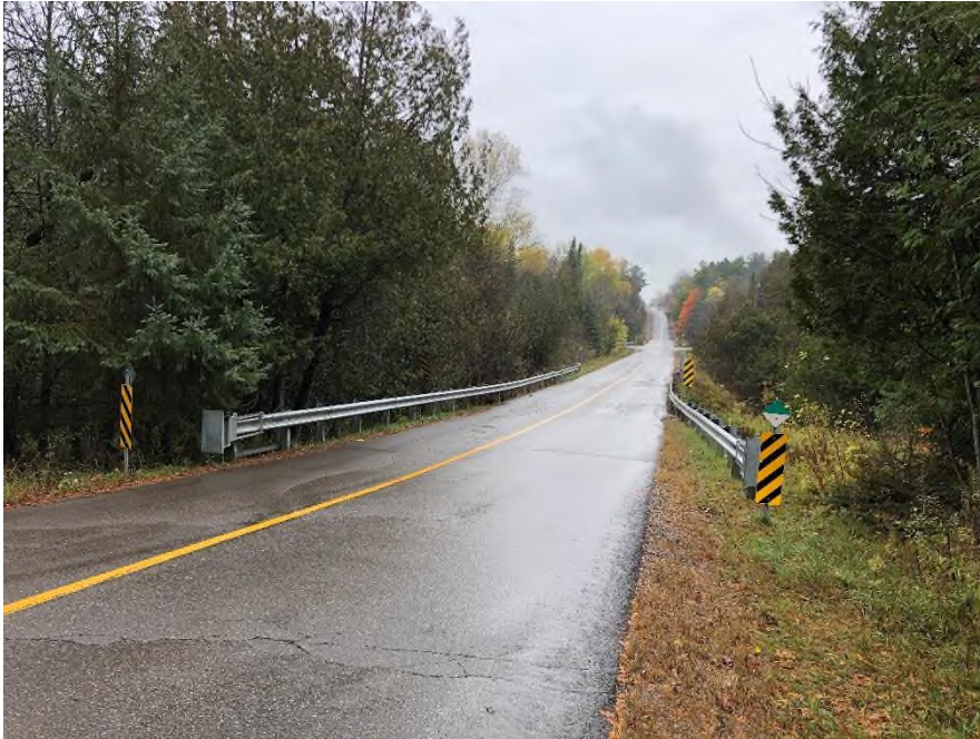
Plate 1: Southern approach towards Bridge No. 1, looking northeast along Patterson Side Road.
