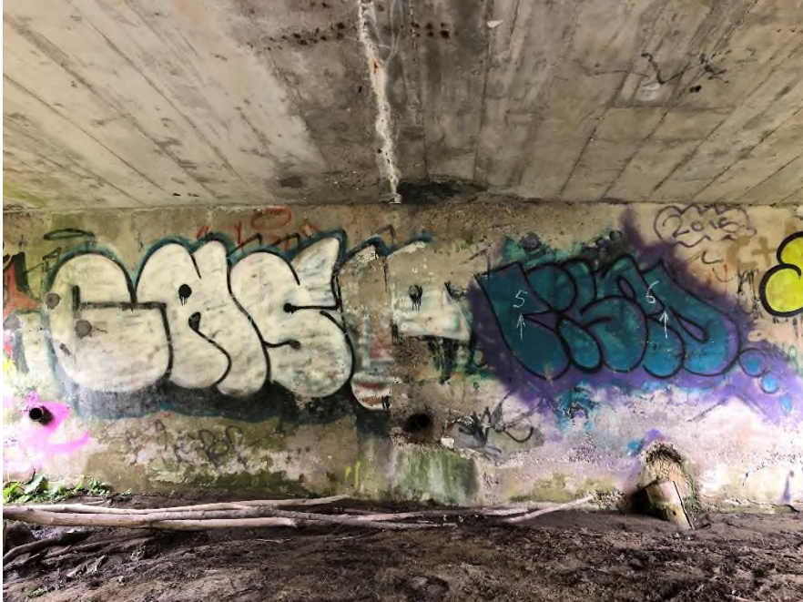
Plate 22: Underside of superstructure and north abutment
