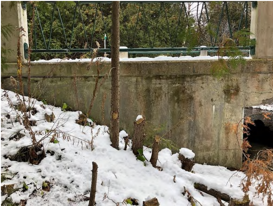
Plate 30: Northeast elevation of the east abutment of Duffy's Lane Bridge.
