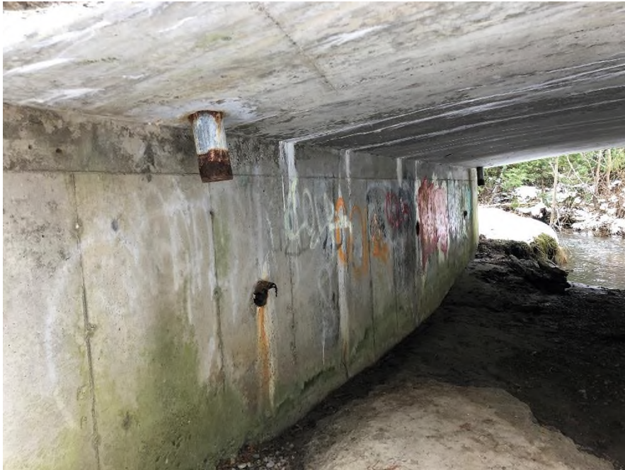
Plate 35: Underside of superstructure and west abutment
