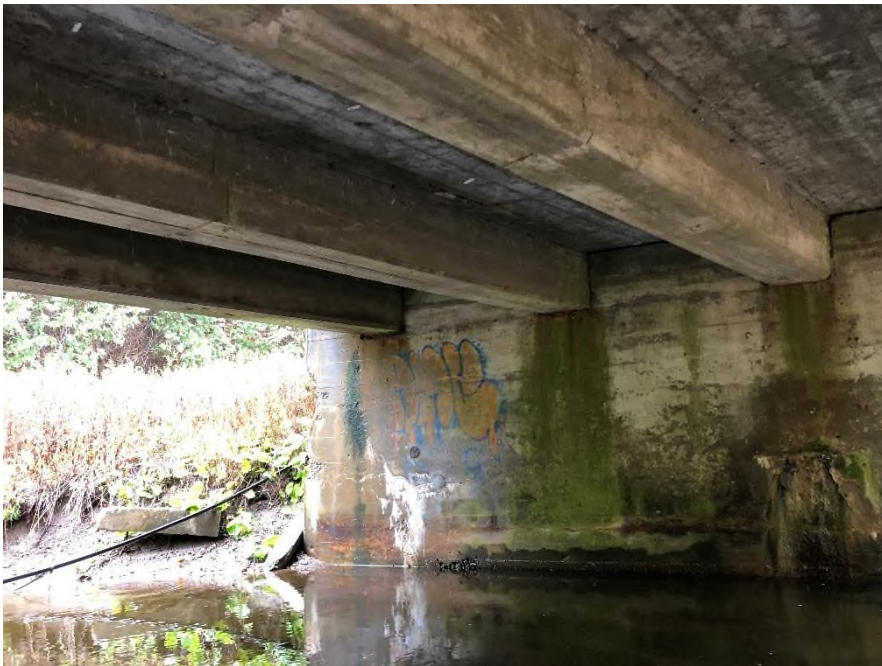
Plate 8: South abutment of Bridge No. 1 and view of concrete T-Beams
