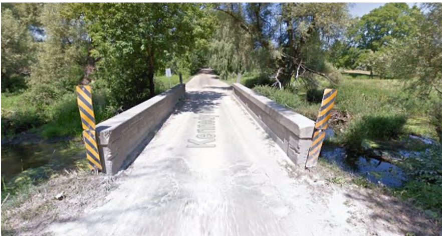
Plate 23: Kennedy Road Bridge, Town of Caledon (Google Maps, 2015)
