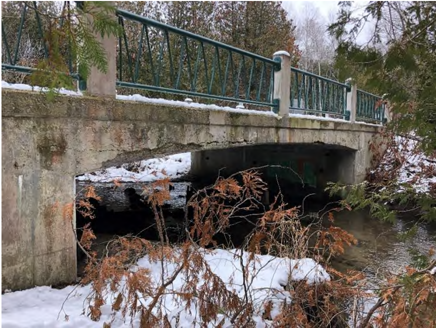
Plate 27: Oblique view of northeast elevation of Duffy's Lane Bridge.
