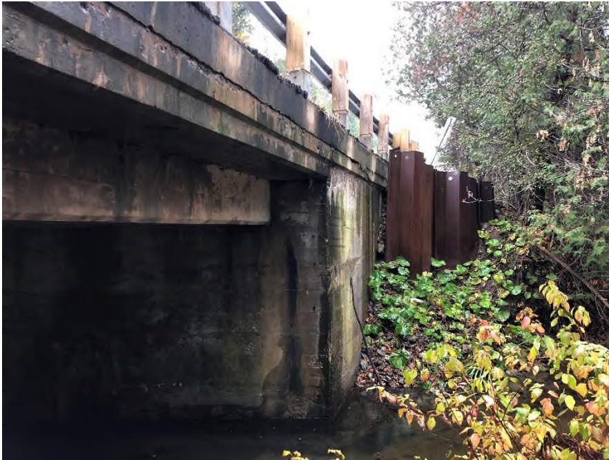
Plate 7: South abutment of Bridge No. 1.
