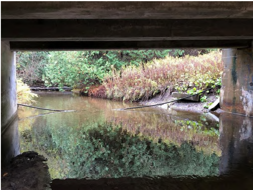
Plate 10: View southeast beneath the bridge structure, along the waterway
