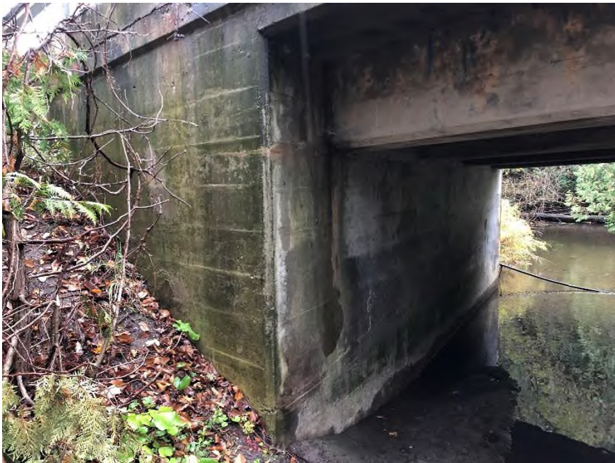
Plate 6: North abutment of Bridge No. 1.
