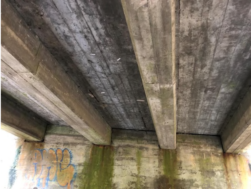
Plate 9: Cast-in-place concrete beams supporting the superstructure of Bridge No. 1.
