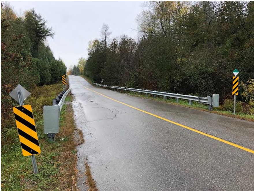
Plate 2: Northern approach towards Bridge No. 1, looking southwest.
