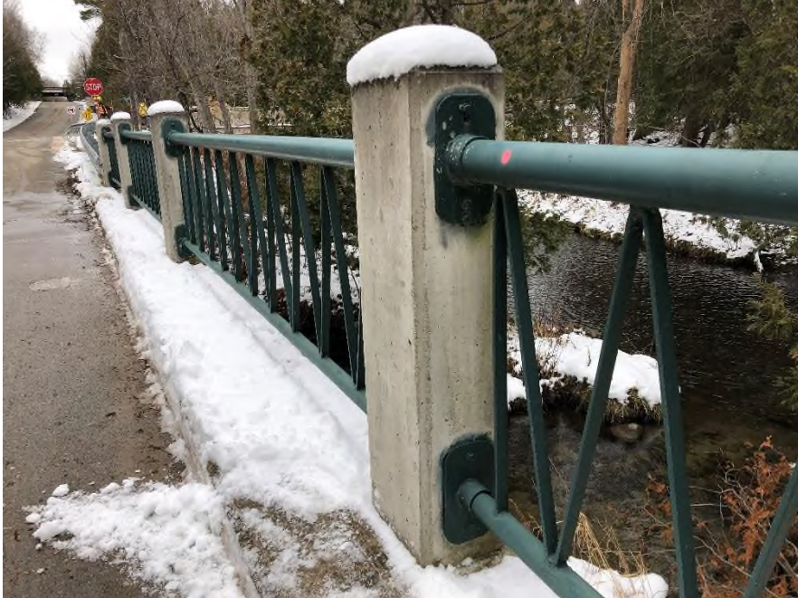
Plate 33: Oblique view of cement post and steel barrier system.
