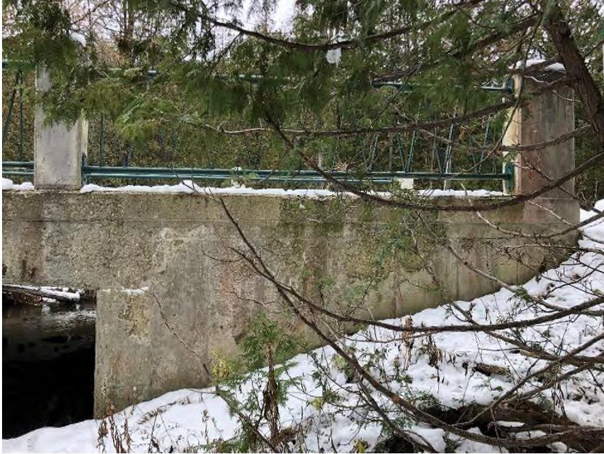
Plate 29: Southwest elevation of the east abutment of Duffy's Lane Bridge.
