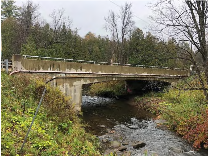
Plate 16: Southeast elevation of Bridge No. 2
