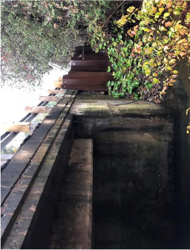
Plate 3: View of Patterson Side Road Bridge 1 over Humber River; Area is disturbed, no potential
