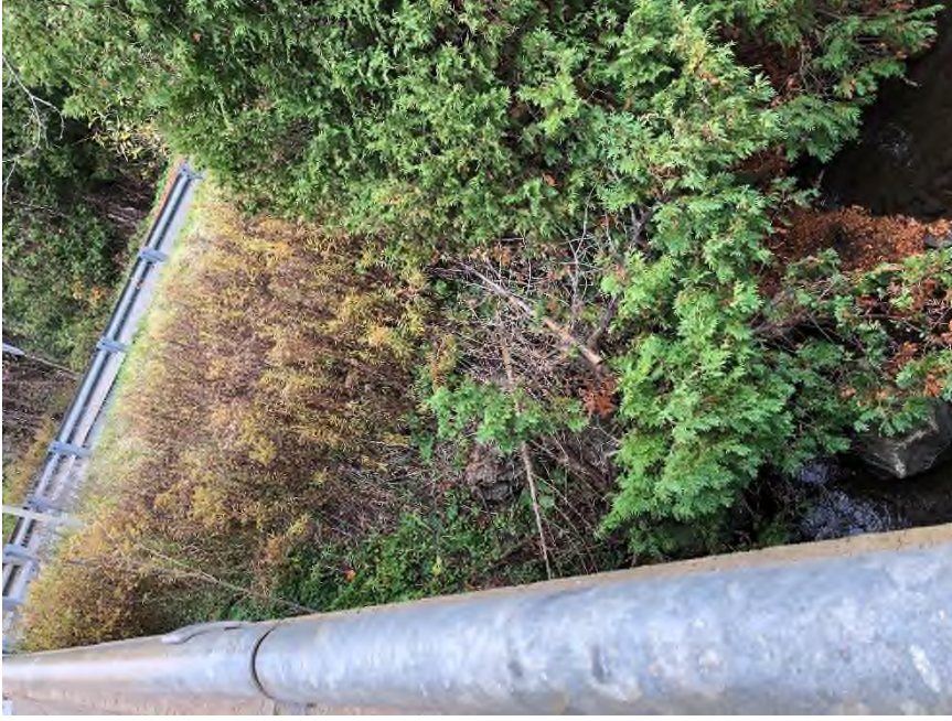
Plate 7: View from Patterson Side Road Bridge 2 over the Humber River
