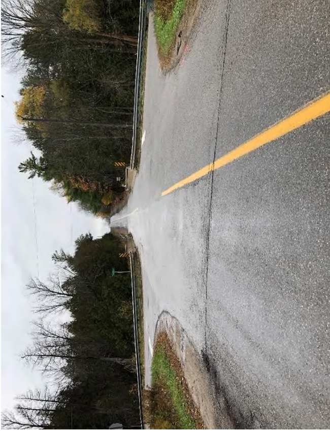
Plate 4: View of Patterson Side Road at Duffy's Lane; Road ROW is disturbed, no potential
