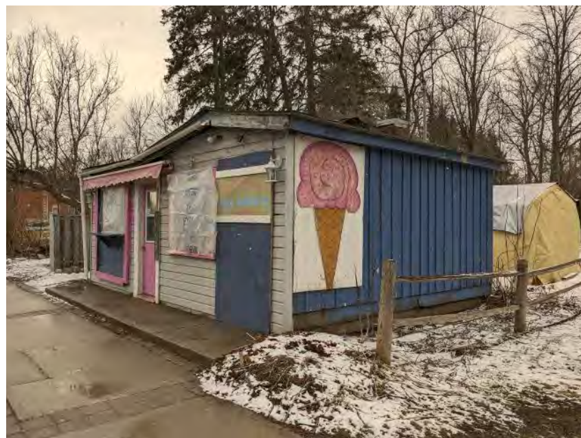
Figure 67: Northeast and northwest façades.
