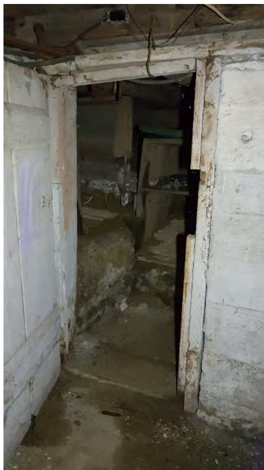
Figure 22: Entrance to crawlspace beneath the Main Block.
