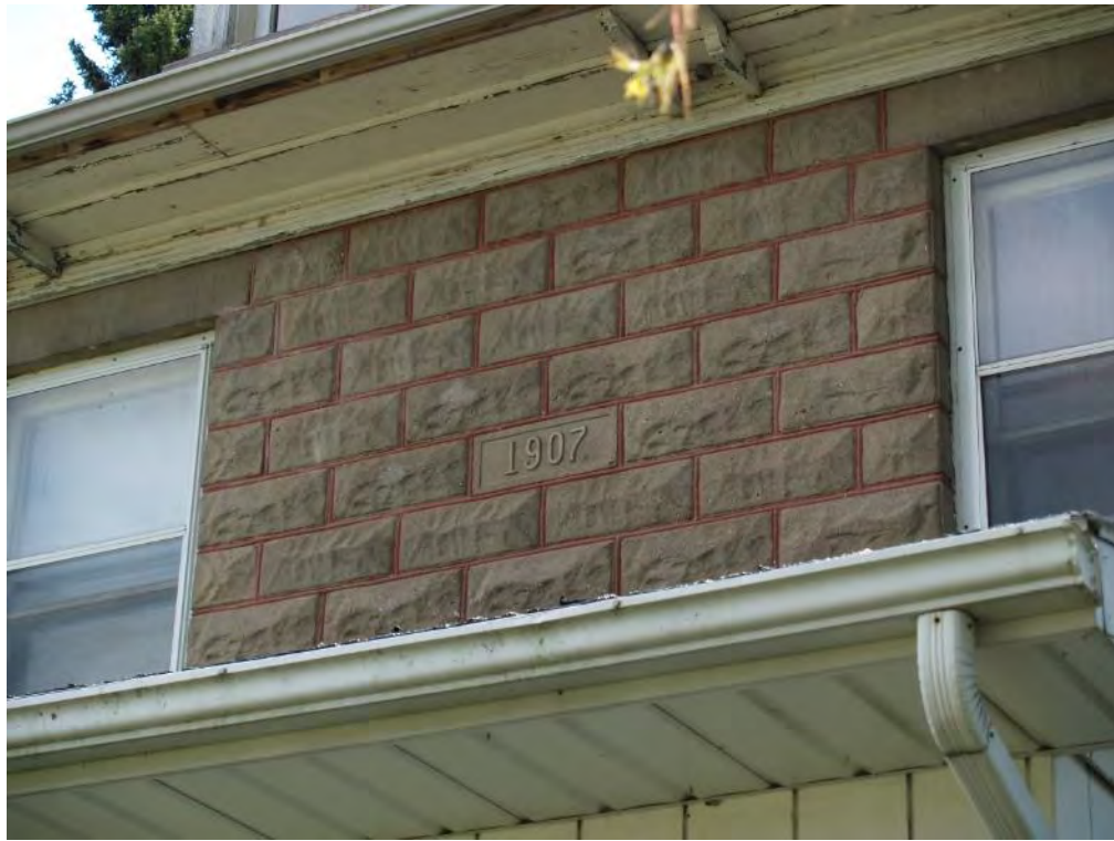
Figure 42: '1907' datestone on the northeast façade.
