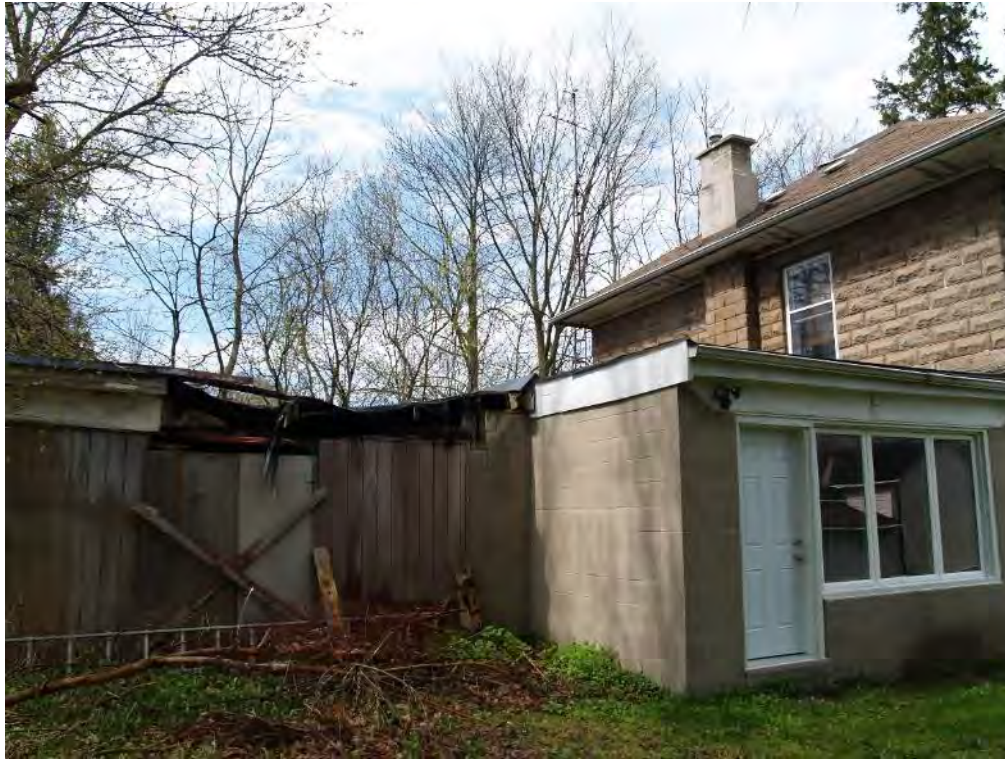
Figure 58: Southwest and southeast façades of the Southwest Addition.
