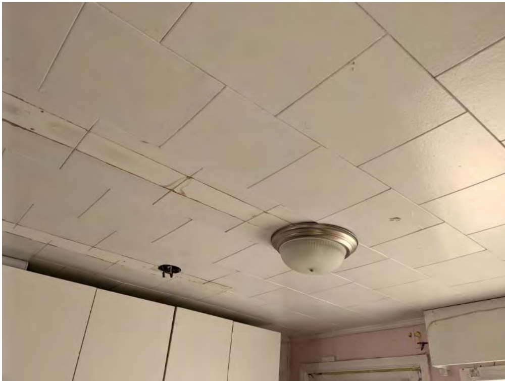
Figure 80: Drop tile ceiling in Main Block.
