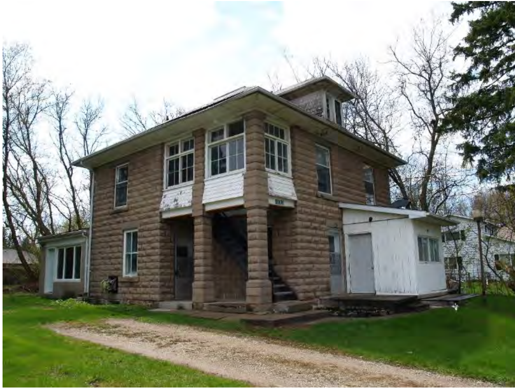
Figure 37: Northeast and southeast façades.
