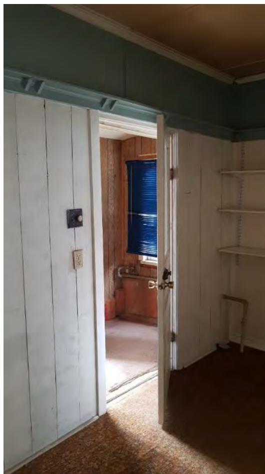
Figure 32: Southwest room, which provides access to the exterior.
