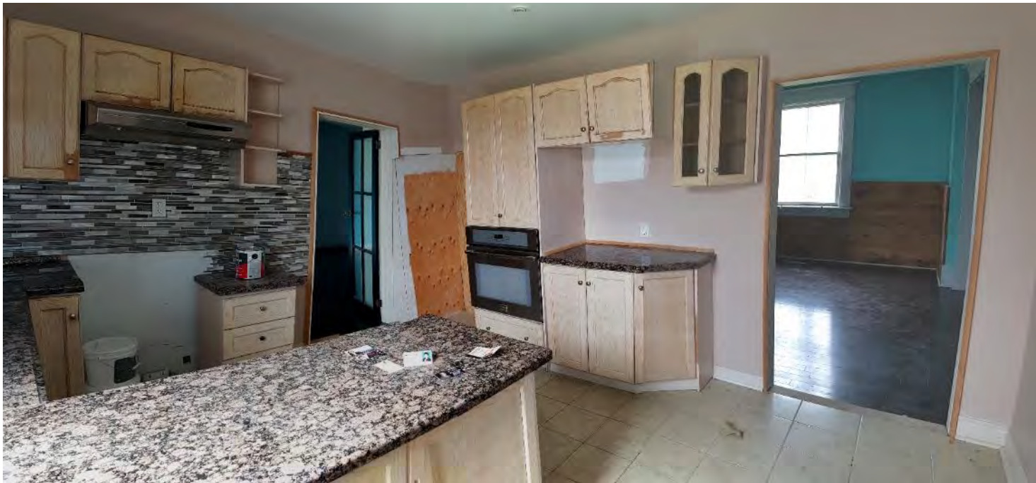
Figure 48: Kitchen showing doorway leading to the Southwest Addition and living space to the north.
