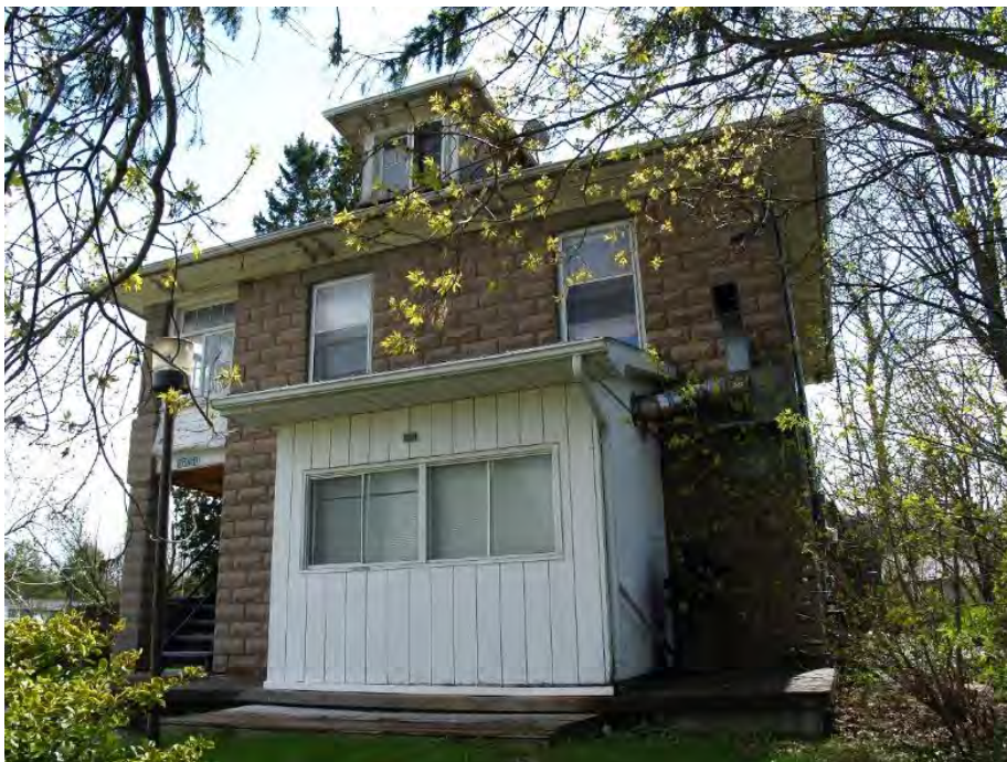
Figure 57: Northeast and northwest façades of the Northeast Extension.
