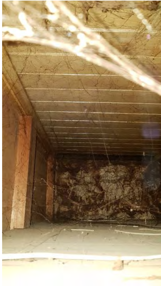
Figure 24: Interior of the attic.
