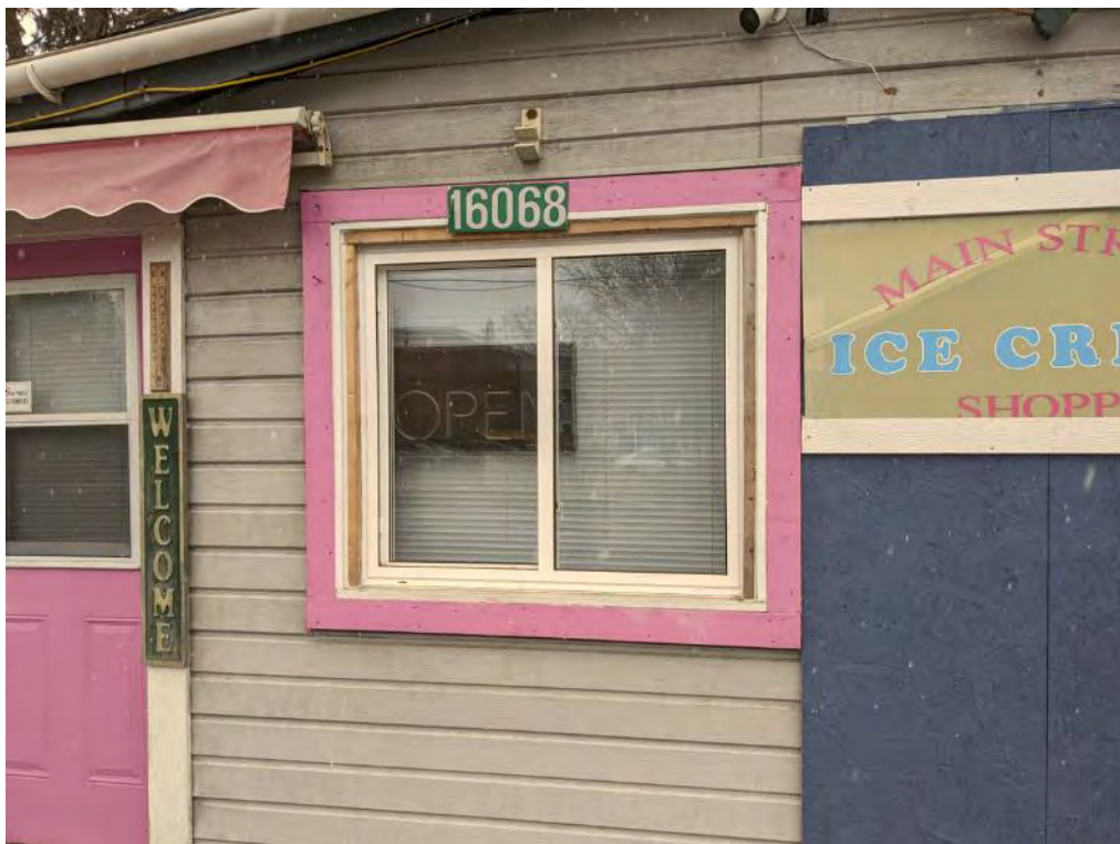
Figure 74: Upgraded horizontal sliding window on northeast façade.
