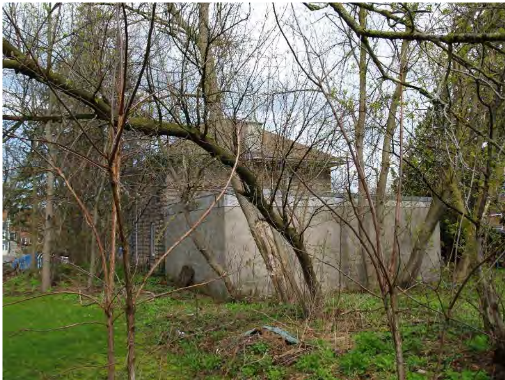
Figure 38: Northwest and southwest façades.
