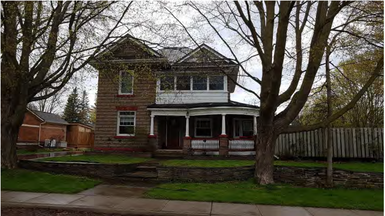
Figure 91: An example of a rockface construction with tinted raised joints at 10 Maple Street.
