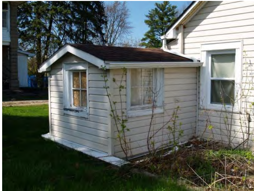
Figure 26: Southwest and southeast façades of the northwest addition.
