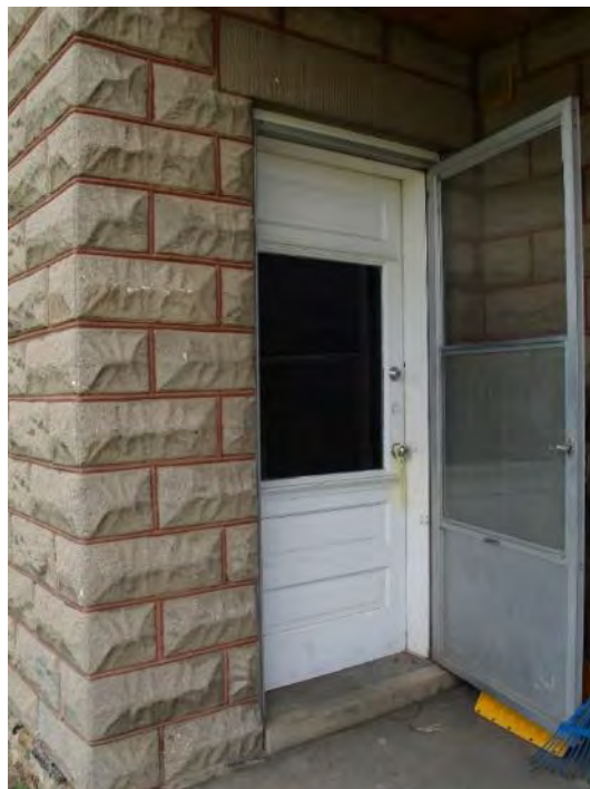
Figure 45: Three panelled off-centre door on the first level.
