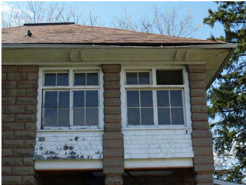
Figure 41: Scalloped wood shingles on the second level.
