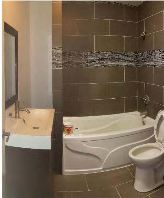
Figure 52: Bathroom at the southwest corner of the living space.
