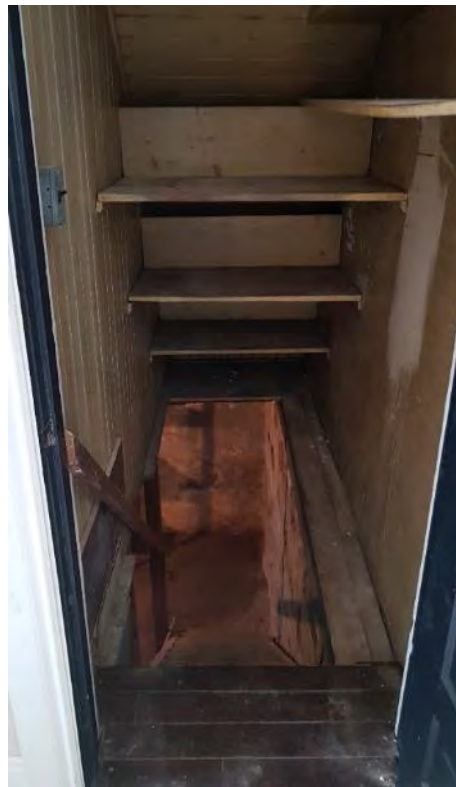
Figure 53: Stairs leading to the basement.
