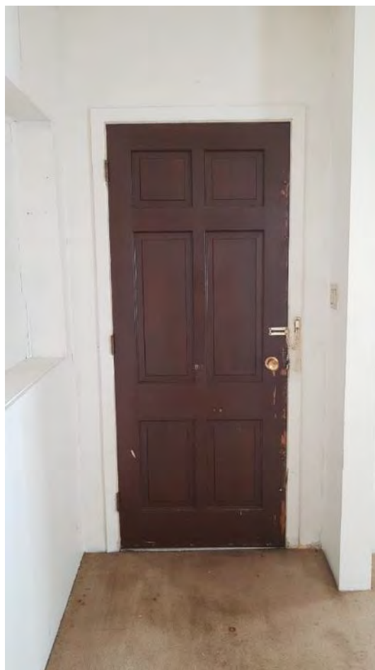
Figure 16: Interior side of the main entrance on the northeast façade.
