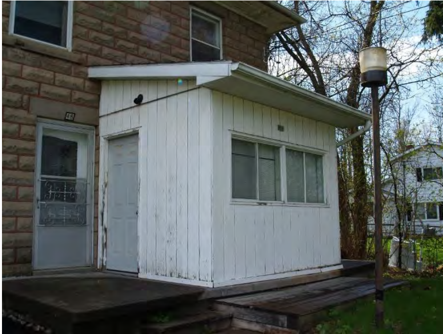
Figure 56: Northeast and southeast façades of the Northeast Extension.
