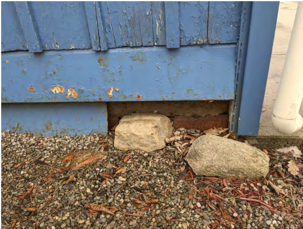
Figure 73: Poured concrete foundation intermixed with brick.
