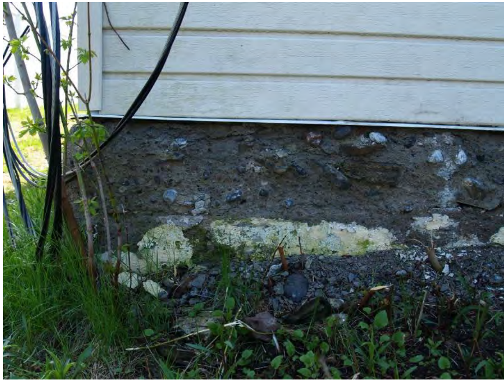
Figure 13: Poured concrete foundation with heavy aggregate base.
