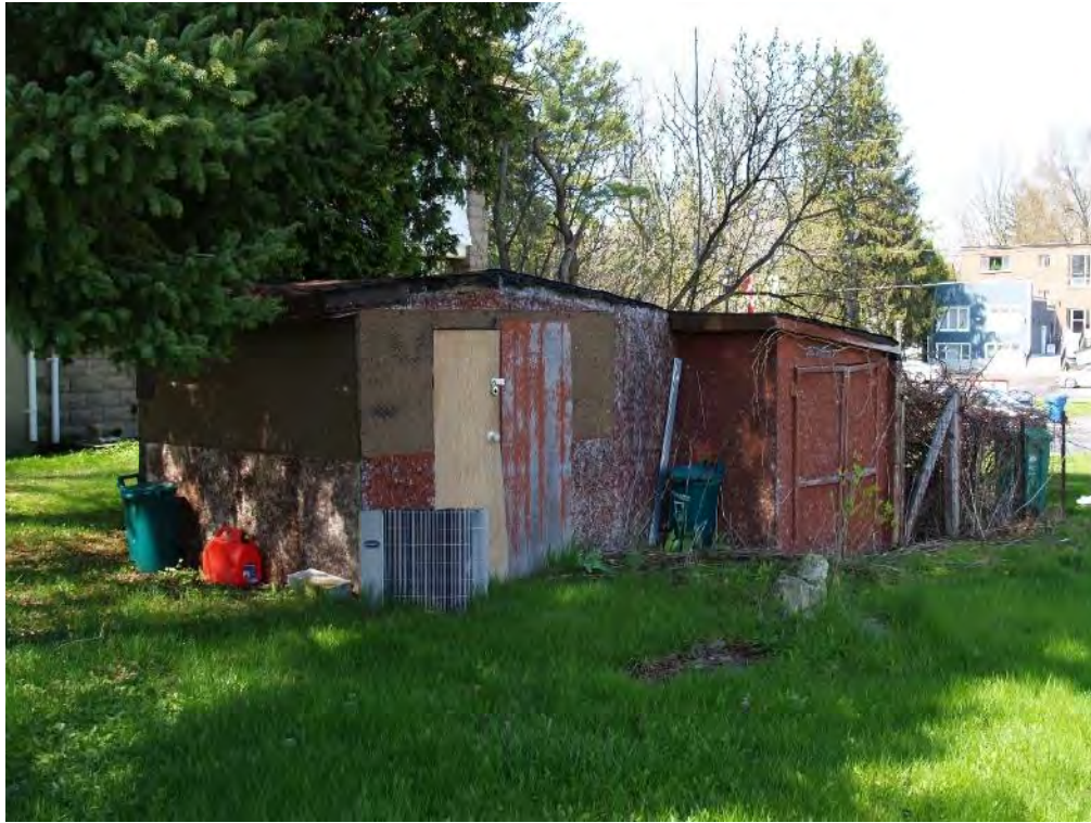
Figure 12: Wood shed to the rear of 16054 Airport Road.
