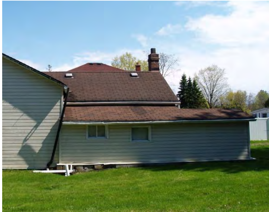
Figure 25: Northwest façade of the northwest addition.
