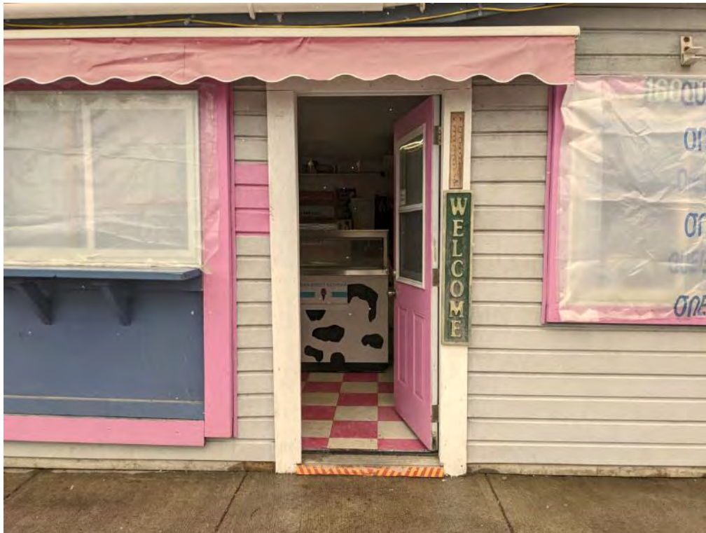
Figure 75: Upgraded single-leaf door with vertical sliding window on northeast façade.
