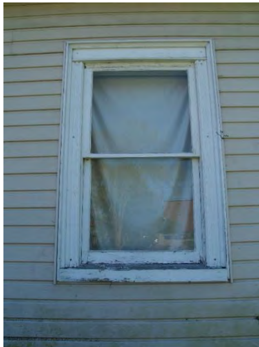
Figure 14: One-over-one double hung window.
