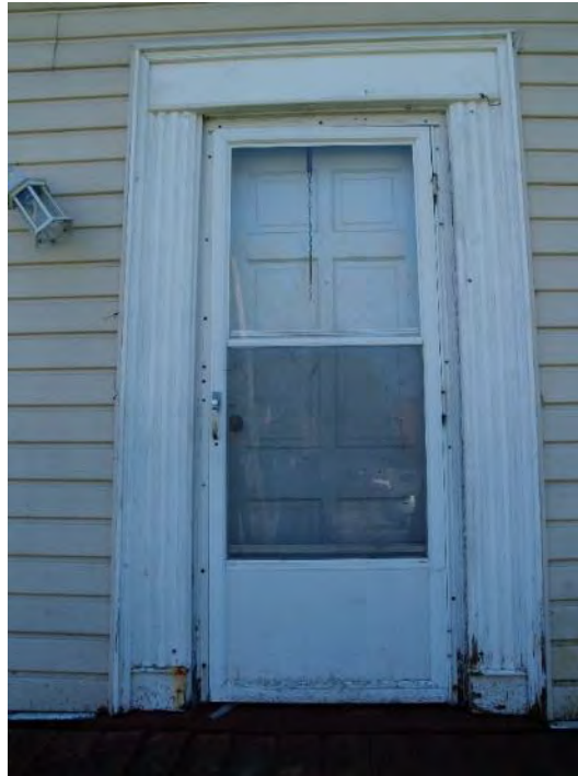
Figure 15: One leaf, six panelled main entrance on the northeast façade.
