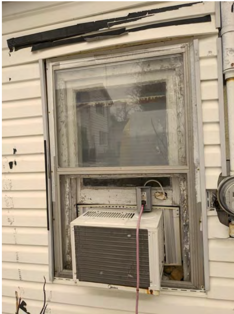
Figure 76: Wood framed one-over-one hung type window on southwest façade.
