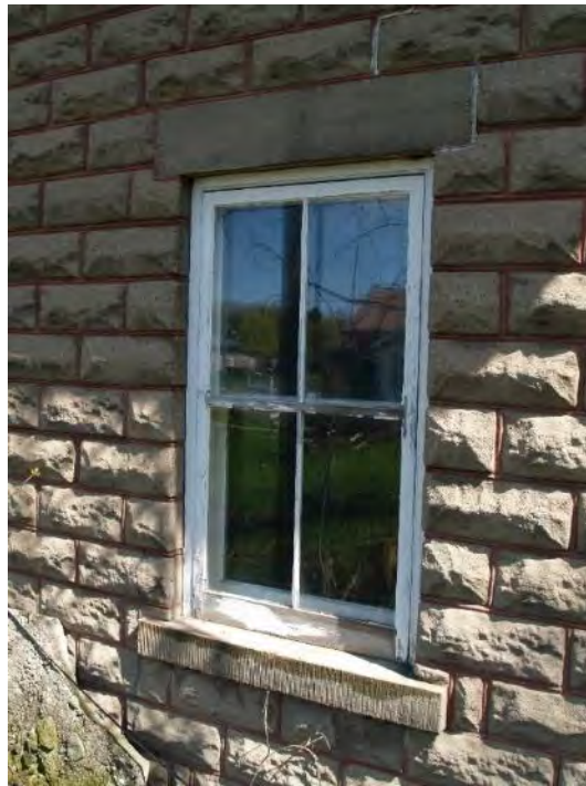
Figure 44: Two-over-two window with plain lintel and lug sill.
