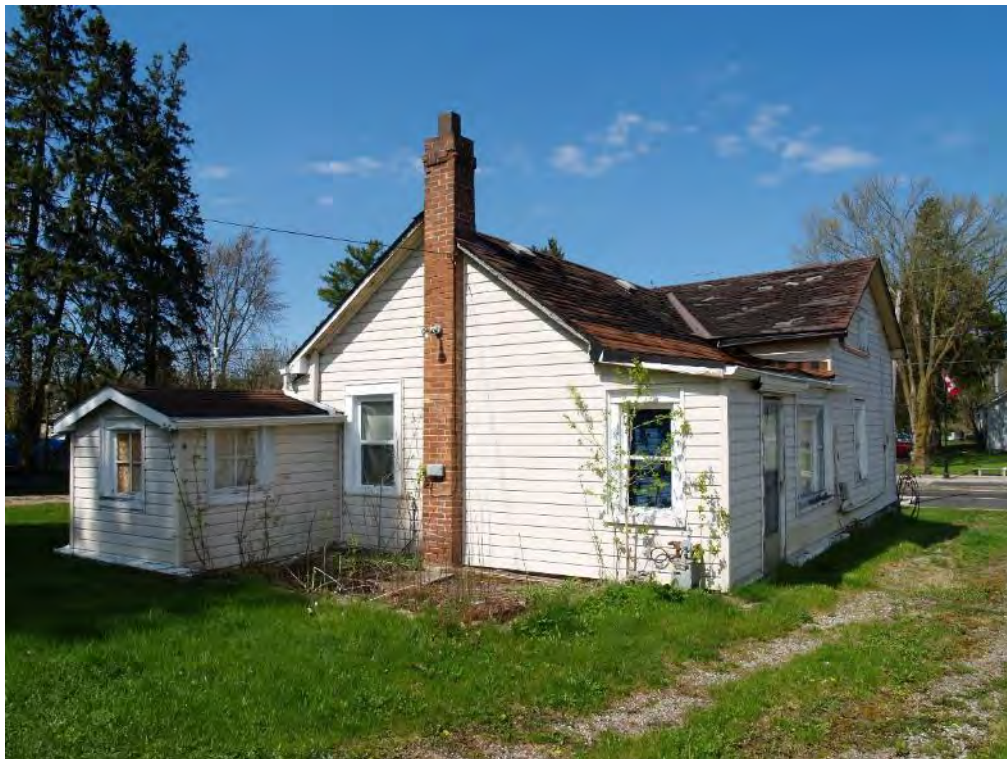
Figure 11: Southwest and southeast façades.
