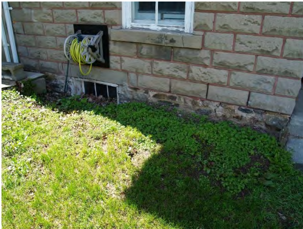
Figure 39: Split fieldstone foundation.
