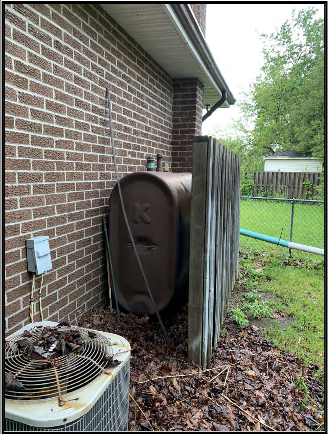
Photograph 2: The Furnace oil AST in the vicinity of APEC1
