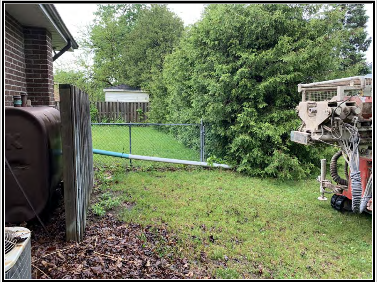
Photograph 3: Drilling BH1/MW1 in the vicinity of APEC 1 (Furnace oil AST)
