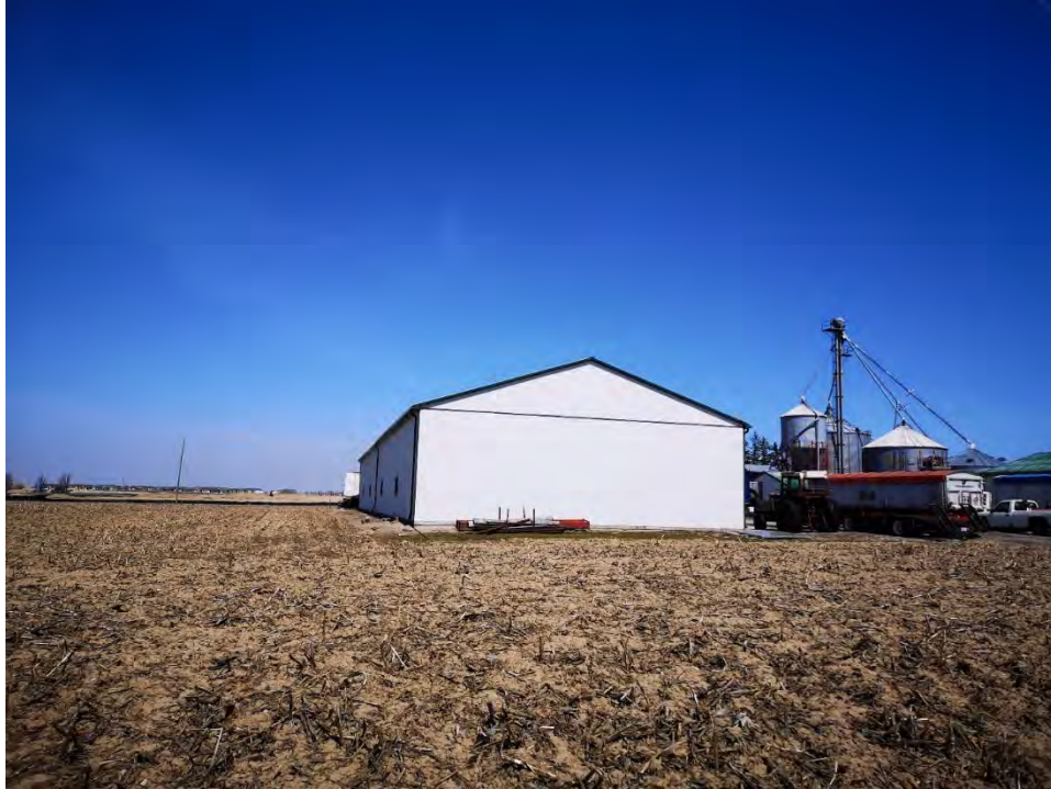
IMAGE 13: 12306 CHINGUACOUSY RD PROPERTY, OUTBUILDING LOCATED WITHIN THE FARMYARD. VIEW FACING NORTH.
