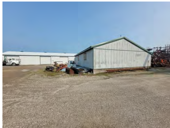
Picture 28: View of Storage Barn 2, facing northwest.
