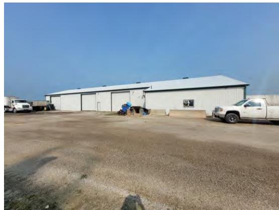
Picture 40: View of the Maintenance Barn, facing west.
