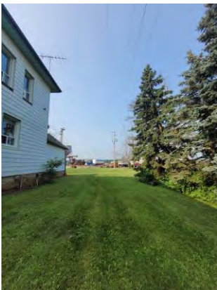
Picture 11: View of the pole mounted transformer and hydro lines, west of the house.
