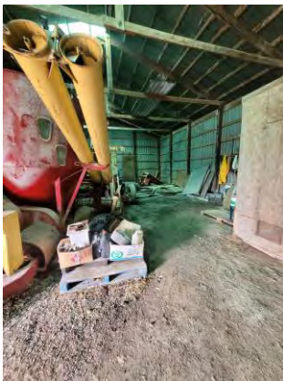
Picture 39: View of the interior of Storage Barn 3, facing south.
