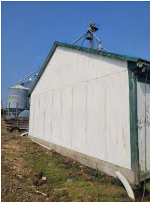
Picture 19: View of Storage Barn 1, facing southwest.
