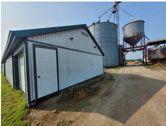
Picture 21: View of Storage Barn 1, facing southeast.
