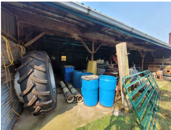
Picture 27: View of the inside of Storage Barn 2, facing southwest.
