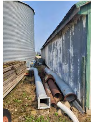
Picture 20: View of Storage Barn 1, facing northwest.
