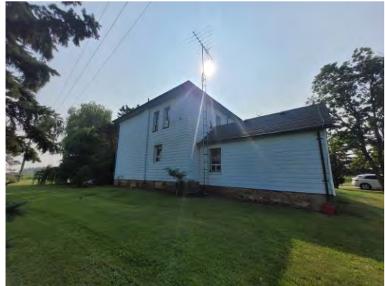
Picture 8: View of the house on Site, facing northeast.
