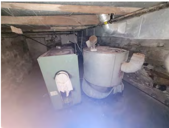
Picture 15: View of the former fuel oil furnace in the basement.
