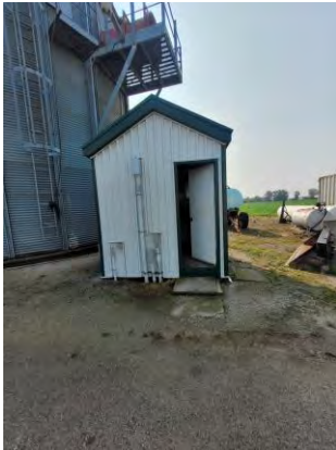
Picture 25: View of the silo control shed, facing east.
