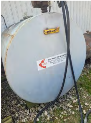
Picture 31: View of the active diesel fuel tank beside Storage Barn 2.
