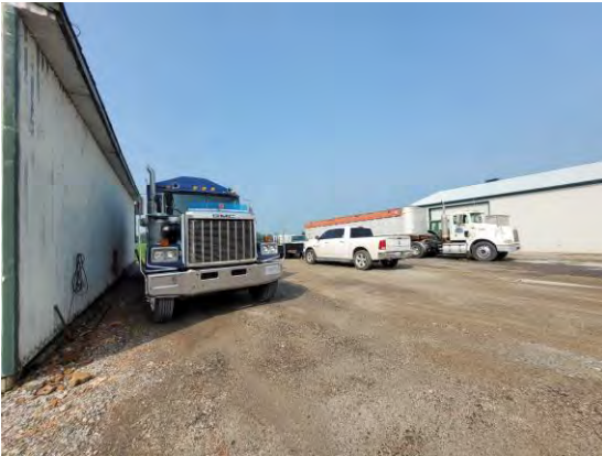
Picture 37: View of the west side of Storage Barn 3, facing southwest.
