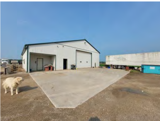
Picture 41: View of the Maintenance Barn, facing southwest.
