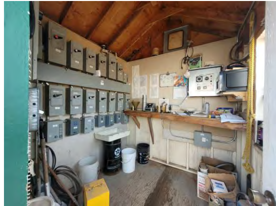
Picture 26: View of the silo control shed, facing northeast.
