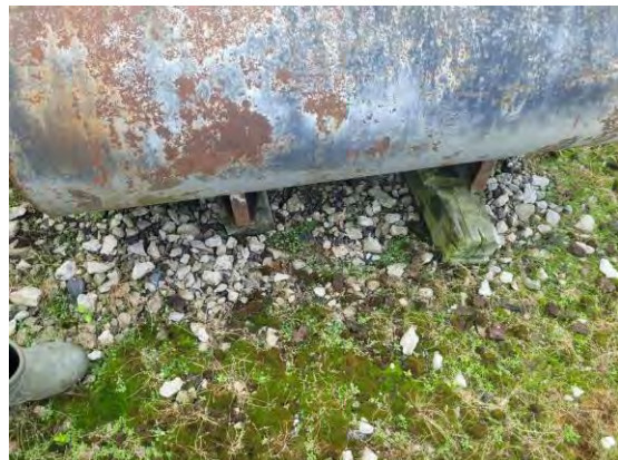
Picture 30: View of the old diesel fuel tank beside Storage Barn 2.
