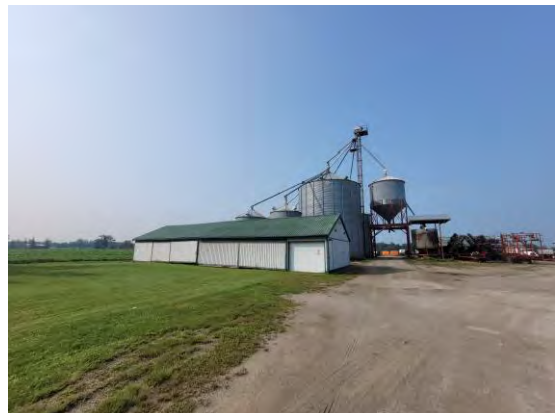
Picture 18: View of Storage Barn 1, facing south.
