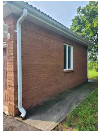
Picture 4: View of the house on Site, facing south.
