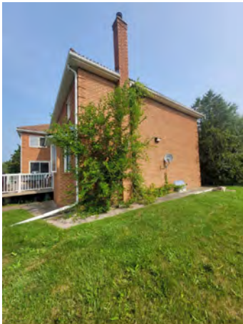
Picture 3: View of the house on Site, facing west.
