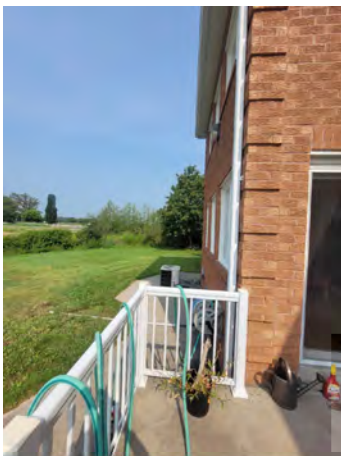
Picture 11: View of the south face of the house with the A/C unit, facing west.
