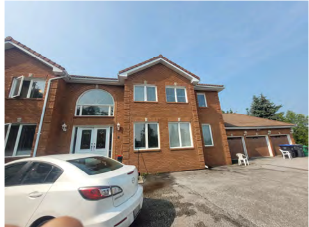
Picture 2: View of the house on Site, facing south.
