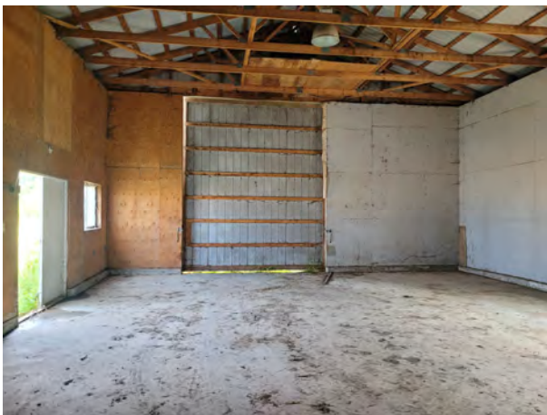
Picture 21: View of the interior of the barn, facing north.
