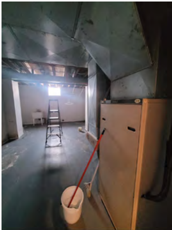
Picture 7: View of the furnace room in the basement.
