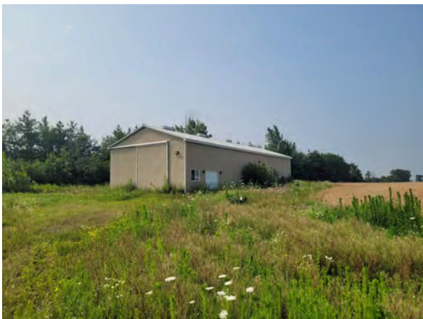
Picture 17: View of the barn on the southeast portion of the Property, facing southeast.
