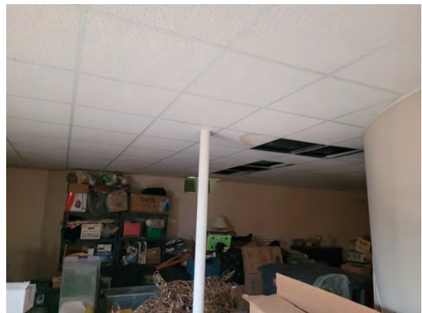
Picture 6: View of the basement of the house.
