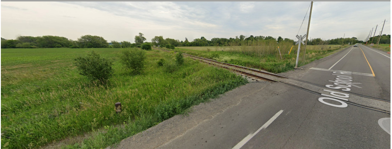
Photo 5: View west along Old School Road at the rail line crossing
