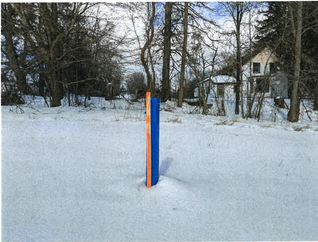
General view of another previously installed groundwater monitoring well on the subject site (looking west)
