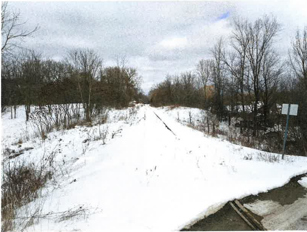
General view of abandoned railway line northeast of subject site (looking north)
