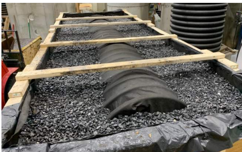
Figure 3: StormTech “Isolator® Row PLUS” Test Set-up at MASWRC
