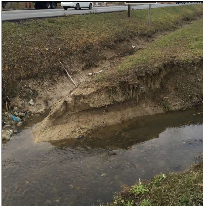
Photograph 3. Tributary as it joins the roadside drainage ditch, showing exposed sands and soil
