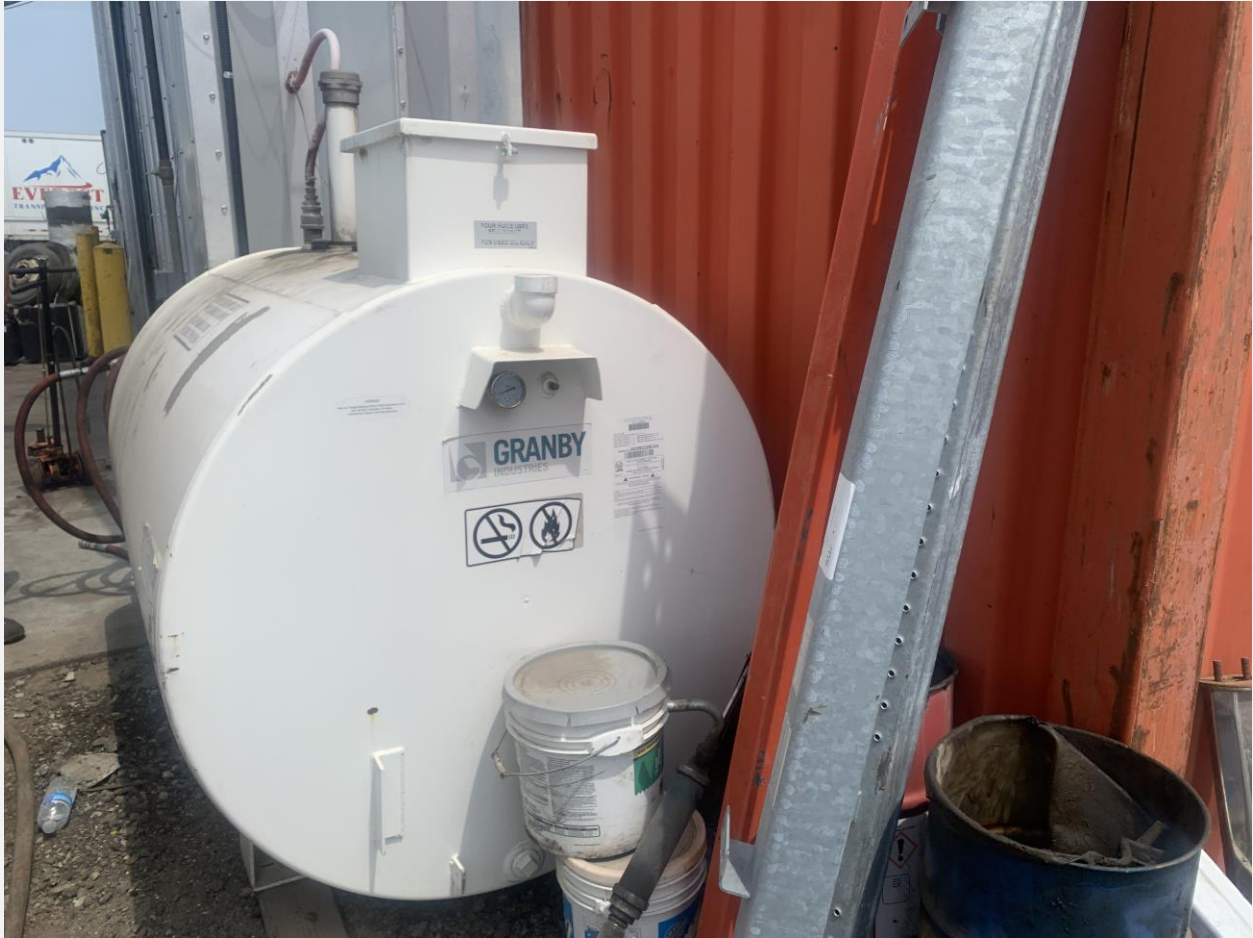
Double-walled Waste oil AST. Noted tag on the right identified volume and other parameters.
