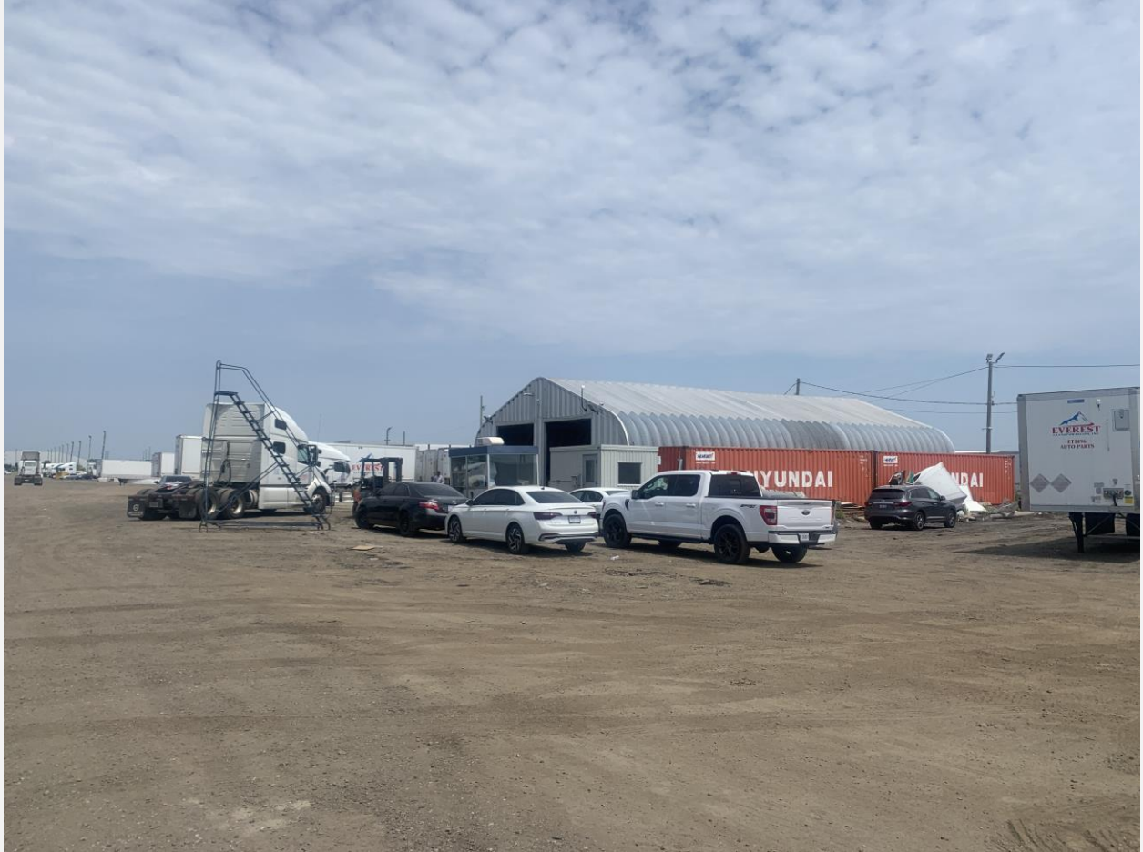
Exterior view of the truck parking terminal and minor repair shop
