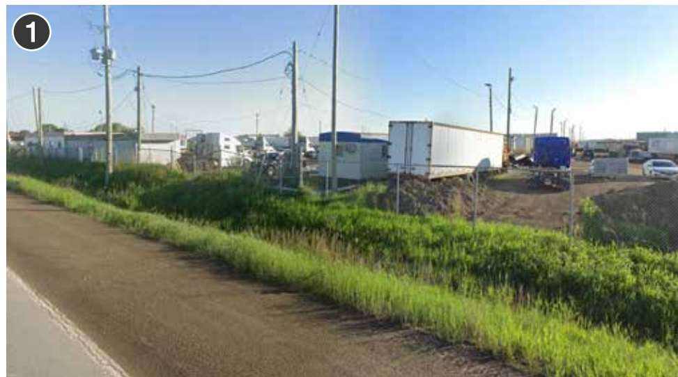
Looking Northeast towards the Subject Property from Coleraine Drive
