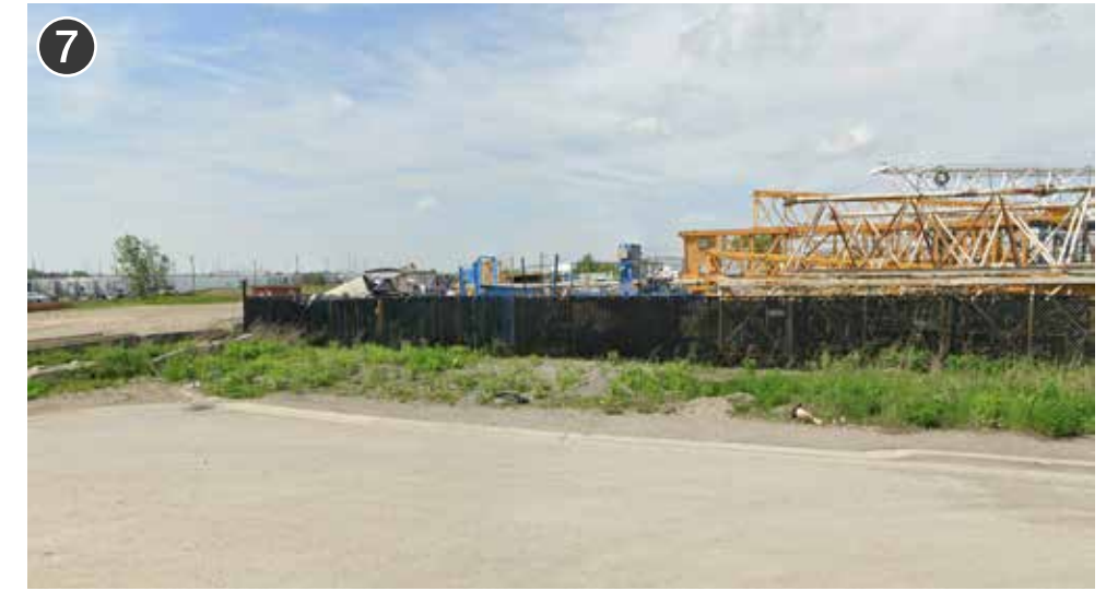
Looking Southwest from Simpson Road and Its Future Extension Adjoining Point
