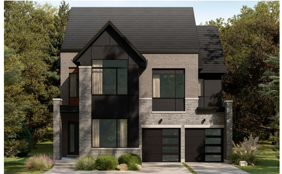
Figure 3.3c - A larger proportion of openings to solid wall should be integrated into elevations with prominent public views, such as corner units (Caivan OpenPlan™ 42' single detached lot)
