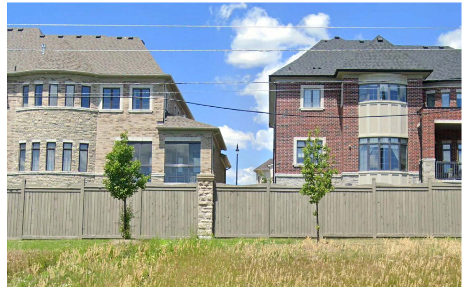
Figure 3.8c - The second storey and roof form may include architectural enhancements such as roof articulation (i.e. gables or raised parapets), upgraded window treatments, frieze board, etc.
