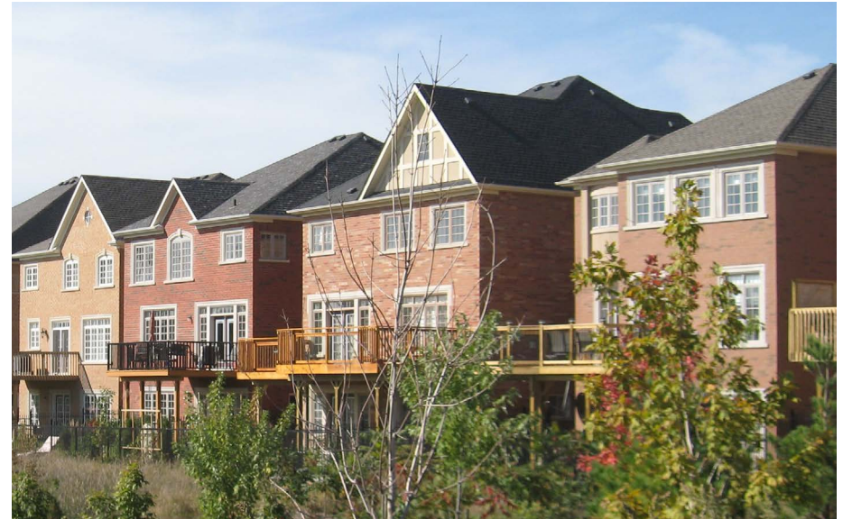
Figure 3.8b - Upgraded rear architecture is required where elevations are exposed to public view
