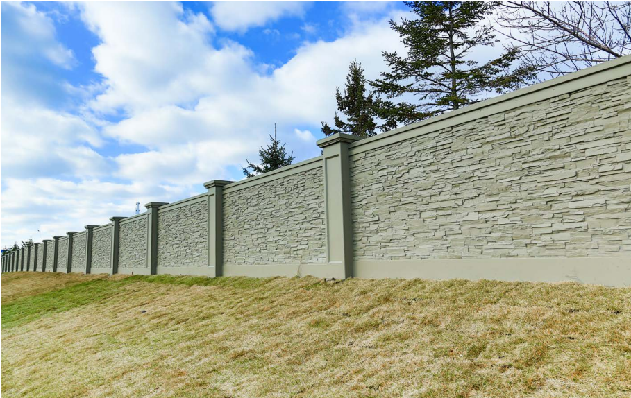
Figure 2.2f - Image example of a precast concrete wall for noise attenuation along a 400 series highway
