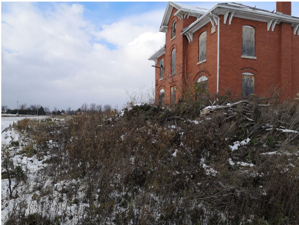
IMAGE 6: FRONT OF HOUSE DEPICTING DISTURBANCE AND BRUSH PILE. VIEW FACING NW
