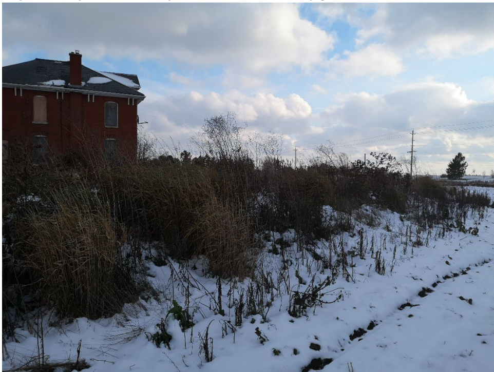
IMAGE 12: W SIDE OF HOUSE AT THE NW CORNER OF THE TEST PIT STUDY AREA. DEPICTS DROP IN ELEVATION FROM THE TEST PIT AREA INTO THE FIELD. VIEW FACING S
