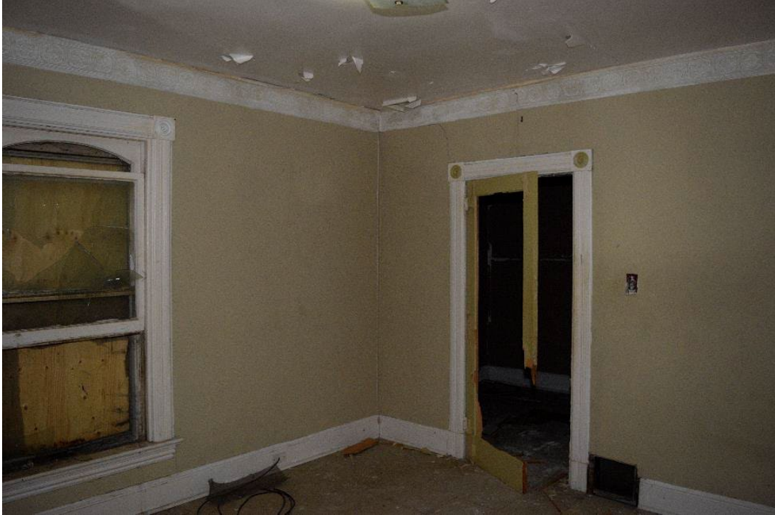
Figure 55: Southeast room second floor, facing southwest
