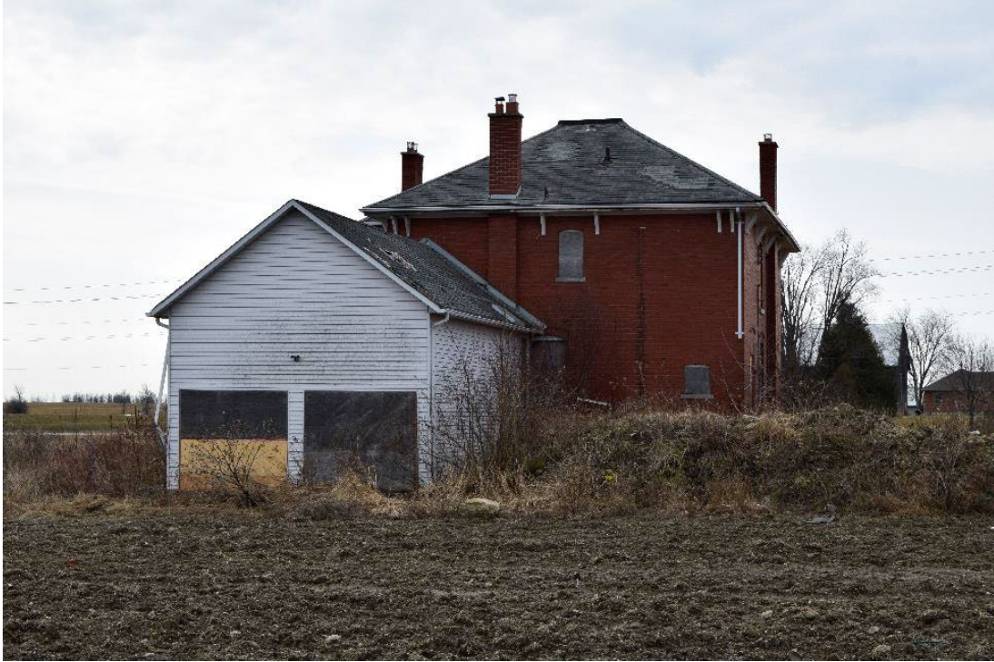
Figure 20: North face of structure, two car garage is a modern addition
