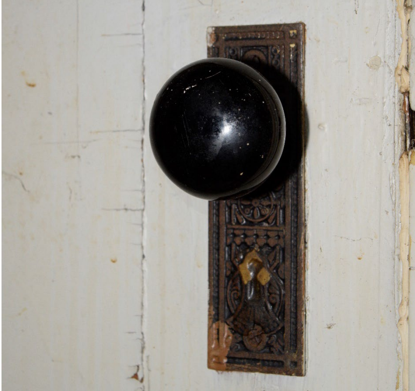
Figure 86: Example of original door hardware, typically referred to as Victorian Style
