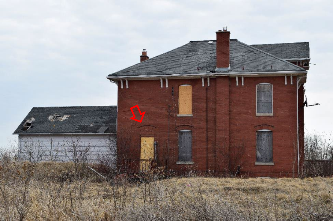
Figure 18: West face of structure, red arrow indicates a window that has been converted to a door
