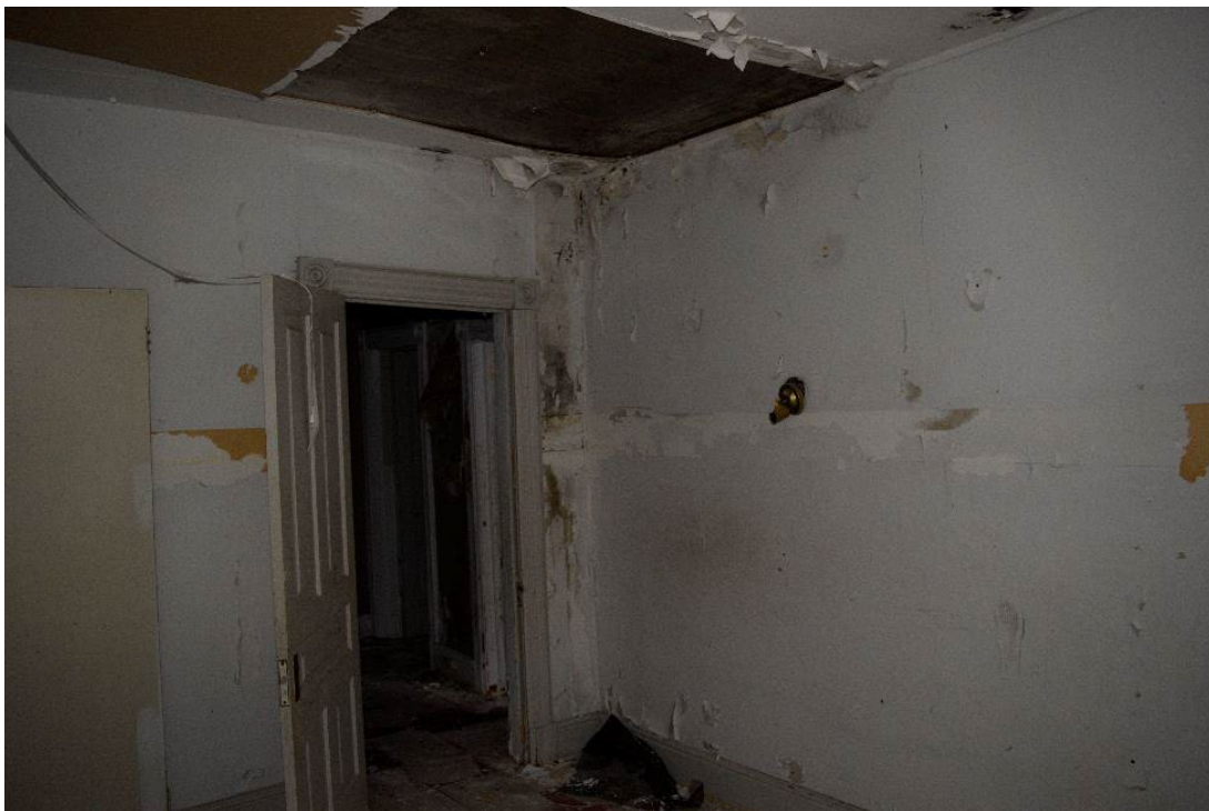
Figure 63: Centre room east side of second floor, facing northwest
