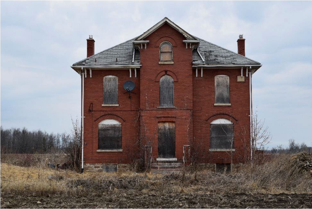
Figure 16: Front façade of structure
