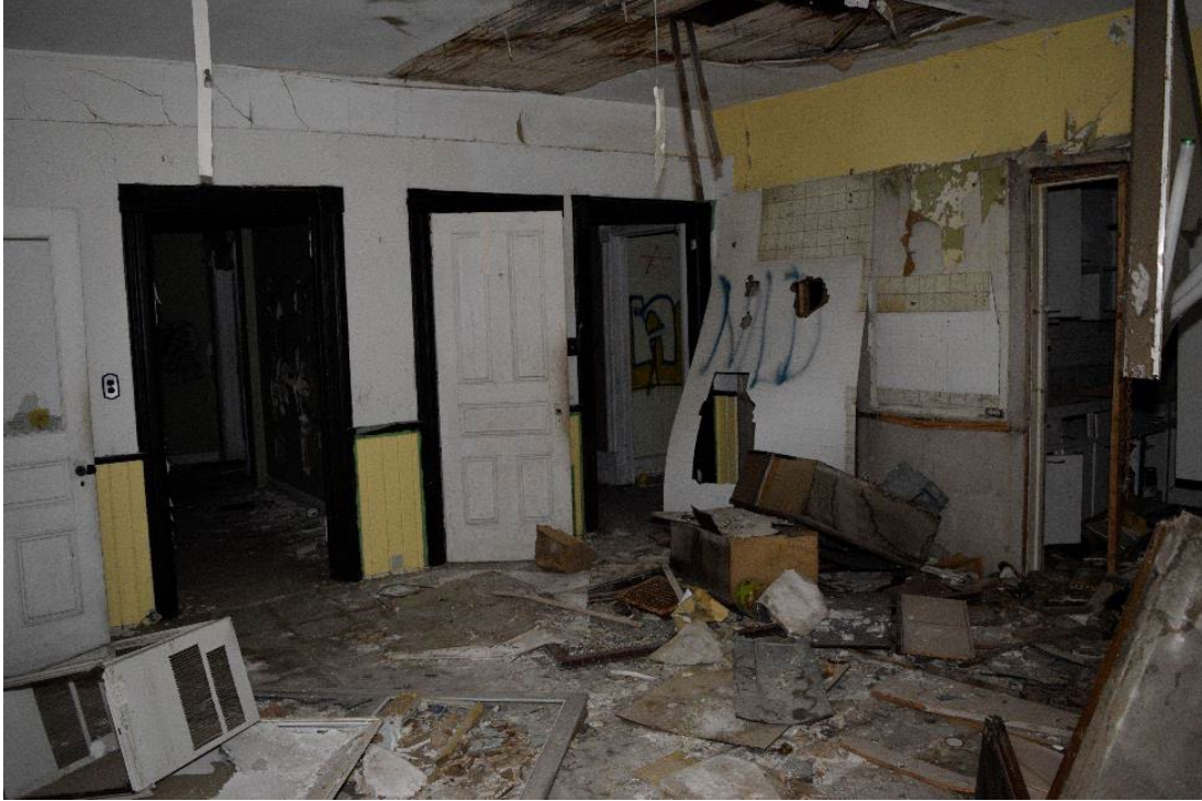
Figure 42: Northeast room, facing southwest
