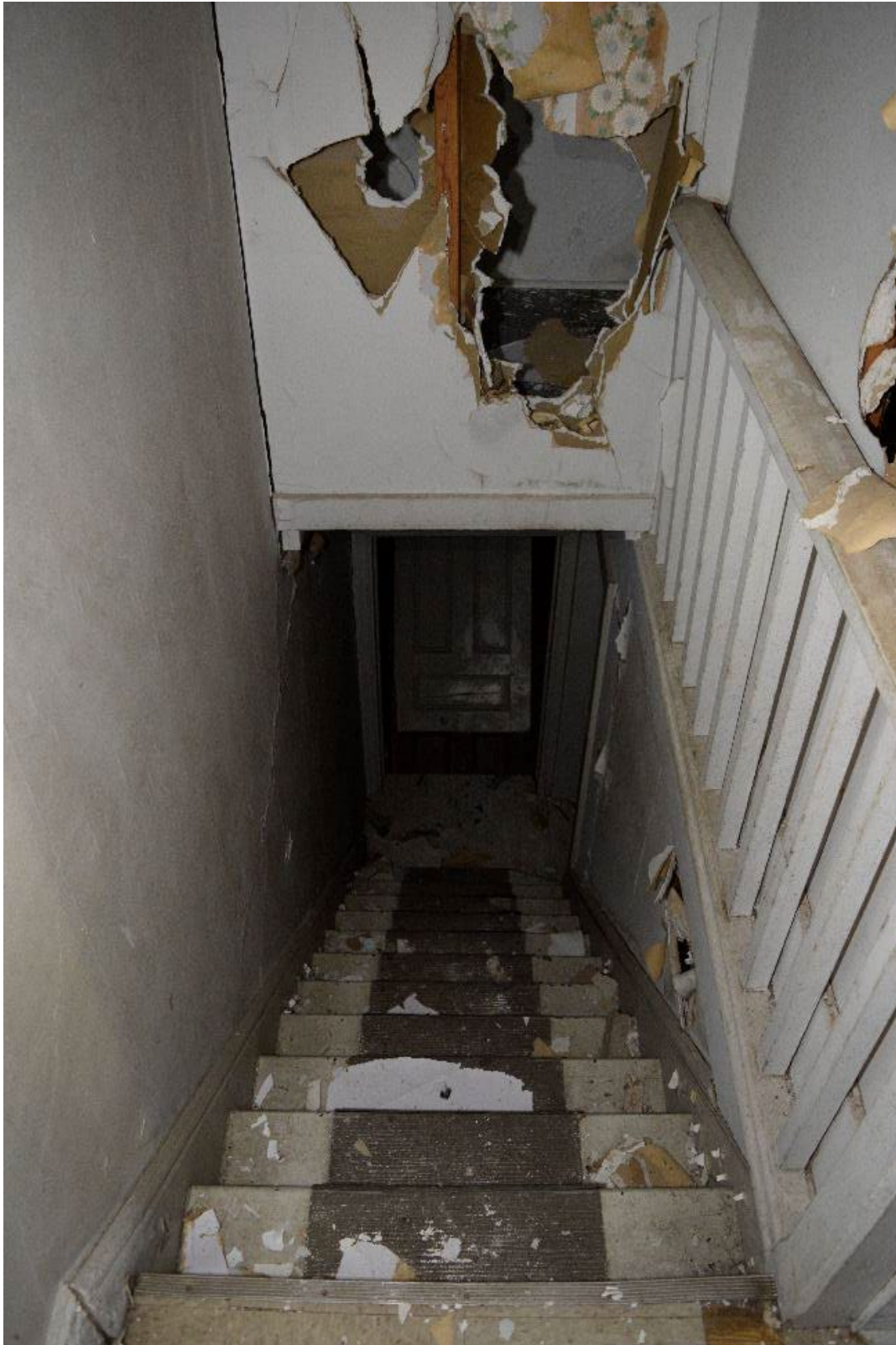
Figure 69: Rear stairs located in northwest corner of structure, facing east
