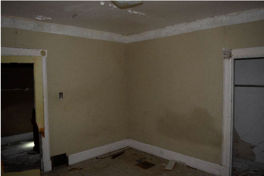
Figure 54: Southeast room second floor, facing northwest
