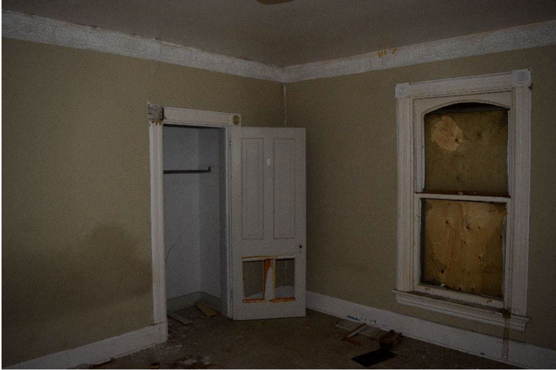
Figure 53: Southeast room second floor, facing northeast
