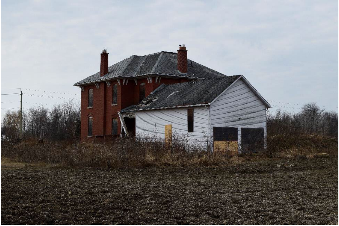
Figure 21: Northeast corner of structure
