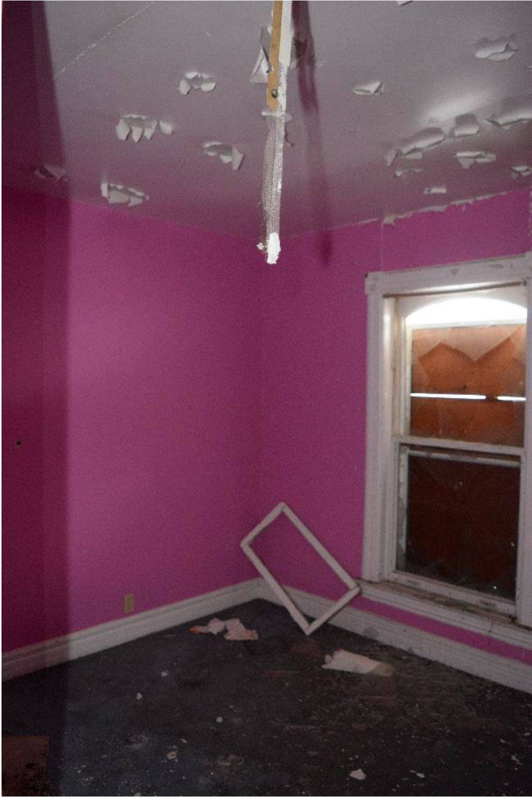
Figure 61: Northeast room second floor, facing northeast
