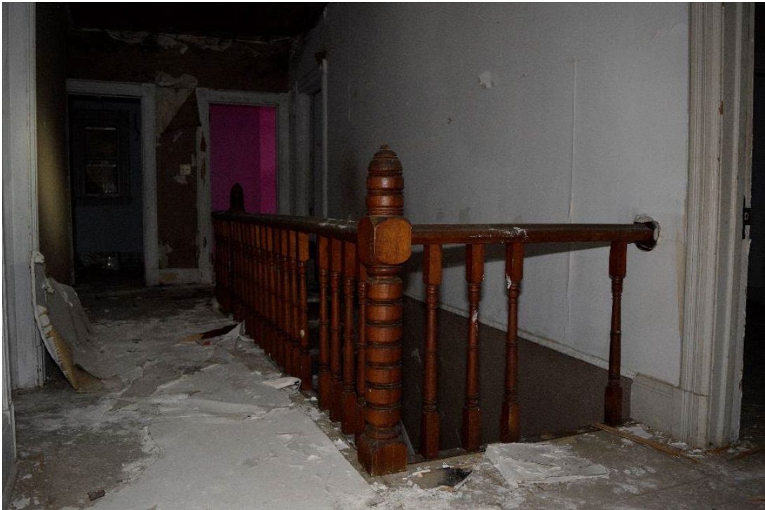
Figure 67: Balustrade second floor, facing north
