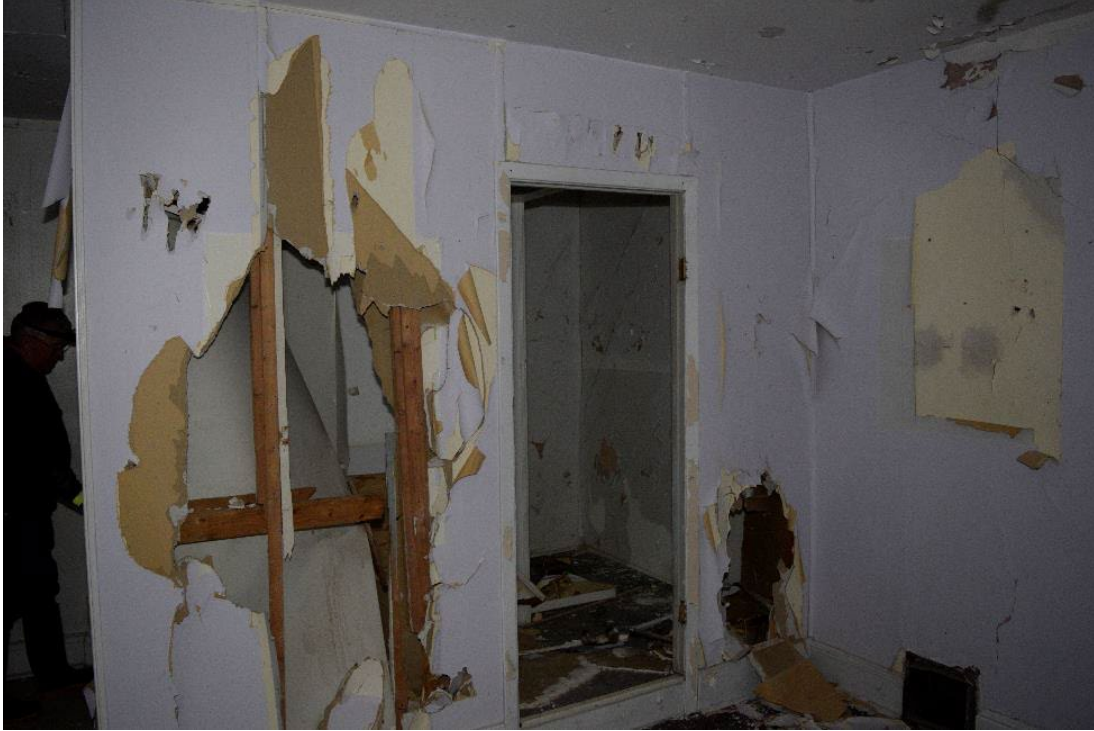
Figure 59: Northwest room second floor, facing northeast
