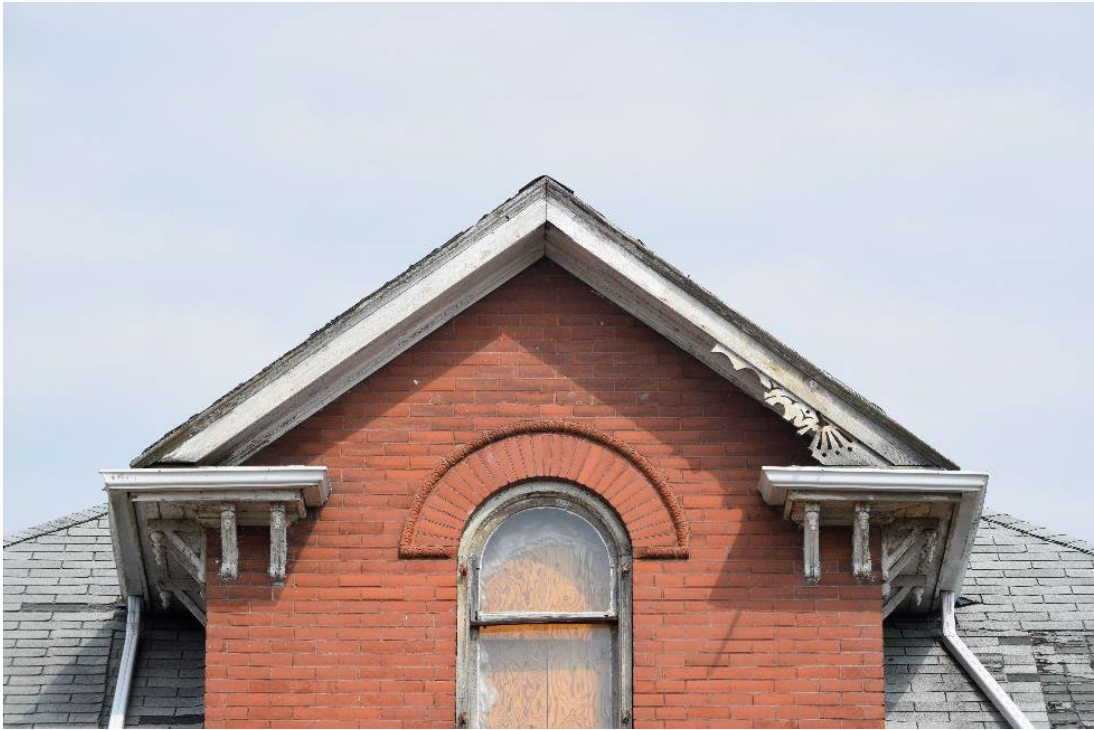
Figure 25: Remnants of decorative millwork associated with centre dormer
