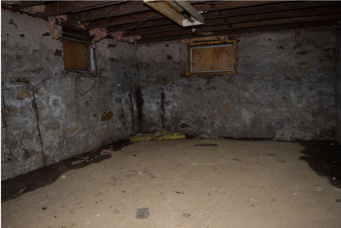
Figure 76: Southeast room of basement, facing southeast
