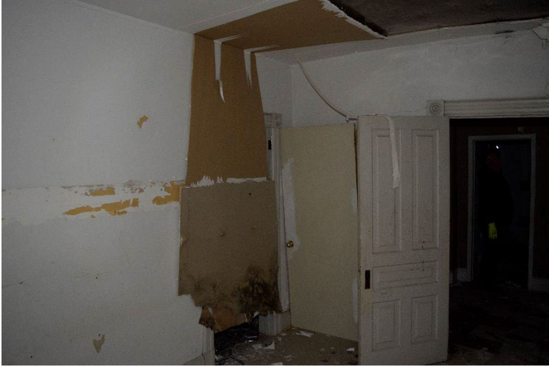
Figure 64: Centre room east side of second floor, facing southwest
