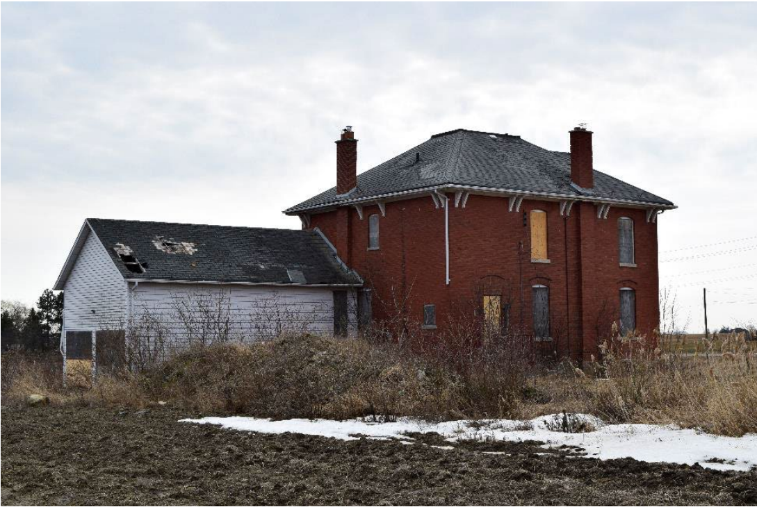
Figure 19: Northwest corner of structure
