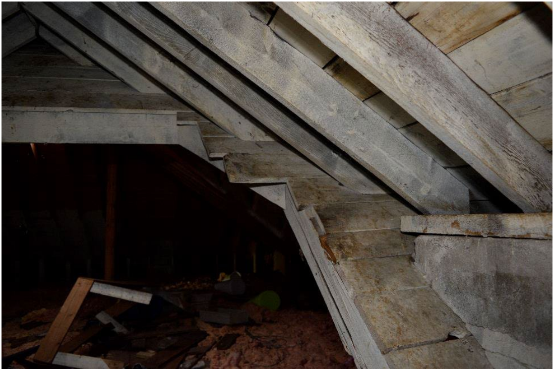
Figure 71: Framing in attic between centre dormer and main roofline, facing north
