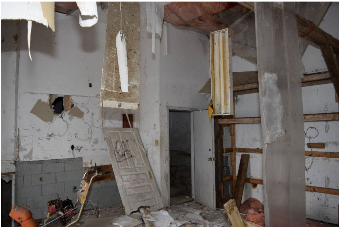
Figure 73: Interior of modern garage, facing southwest
