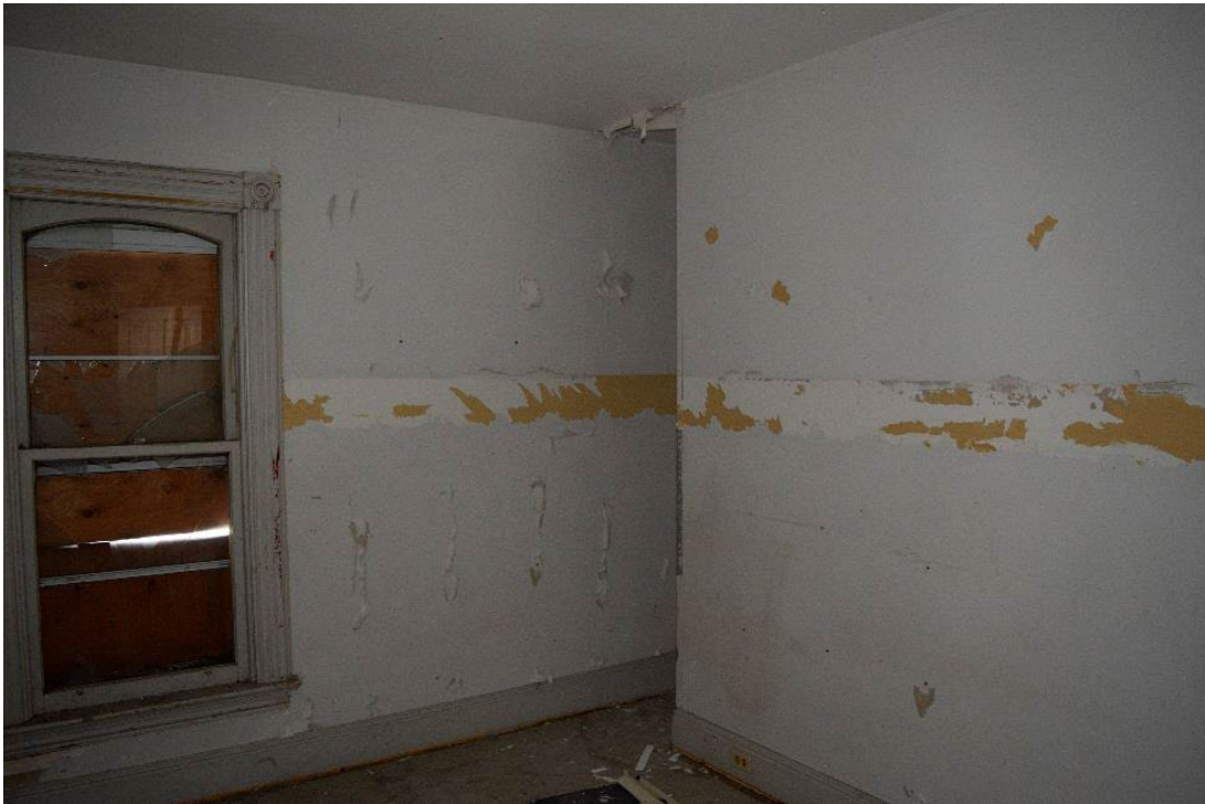
Figure 65: Centre room east side of second floor, facing east
