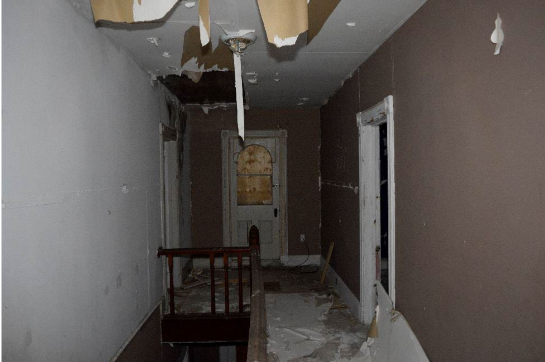
Figure 66: Centre of second floor, facing south
