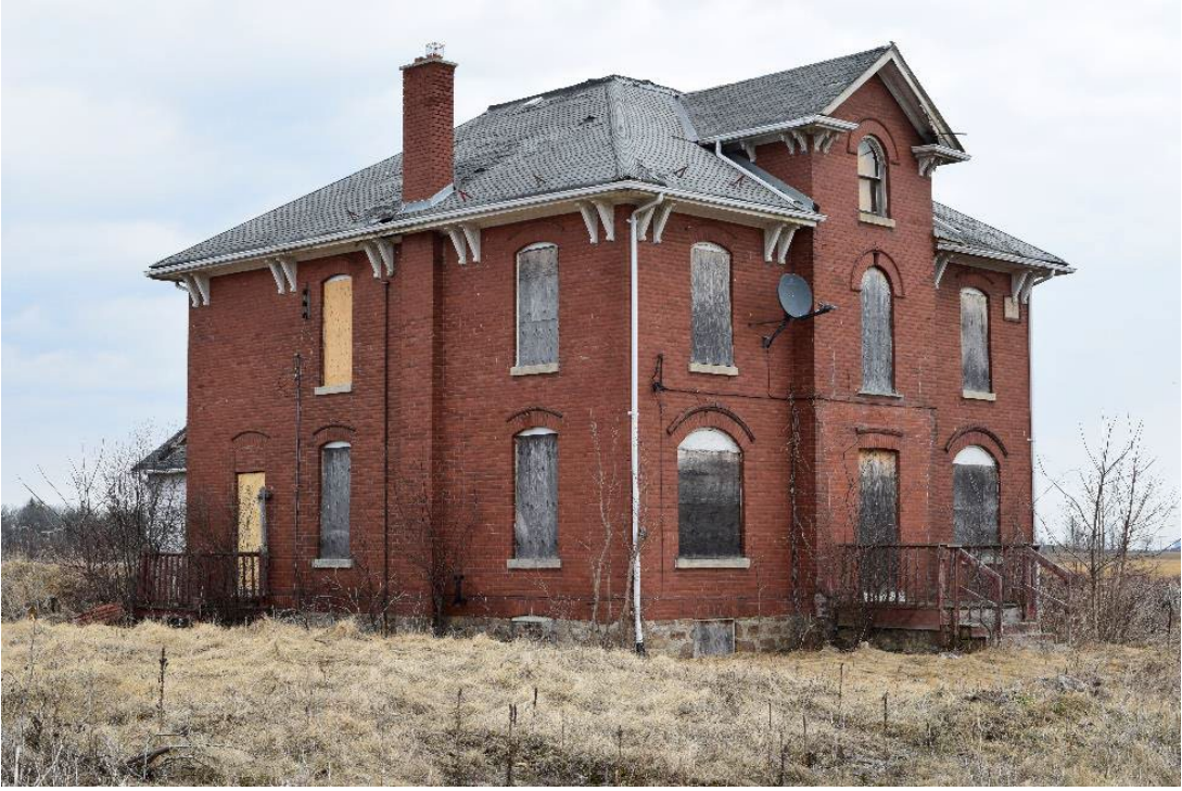
Figure 17: Southeast corner of structure
