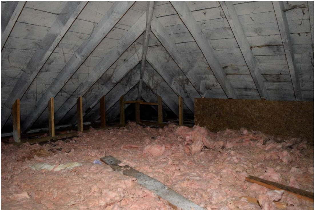
Figure 70: Attic space, facing southeast corner of structure
