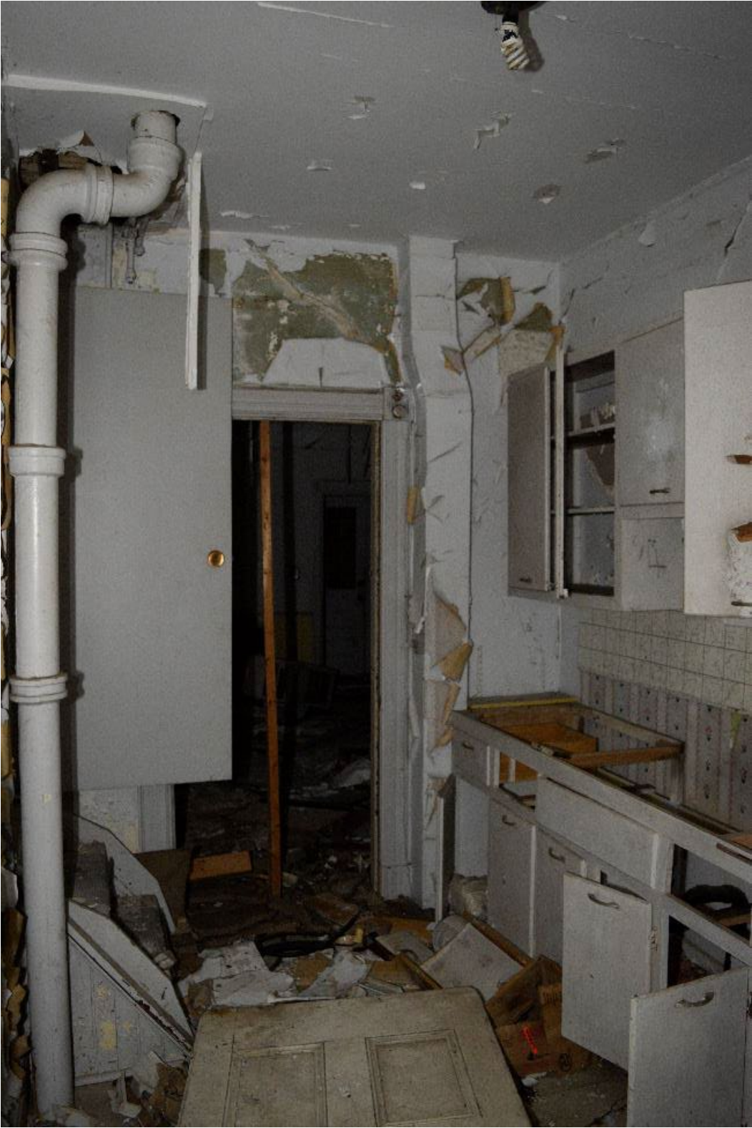
Figure 52: Northwest room first floor, facing east
