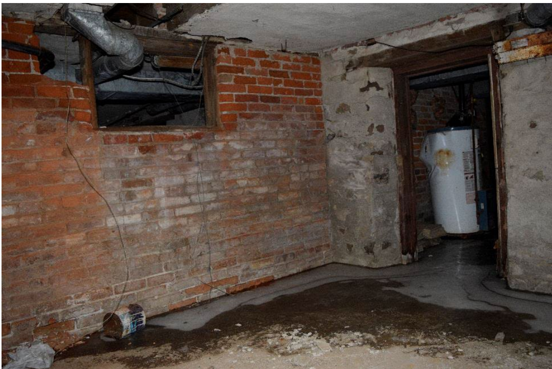
Figure 77: Brick partition in south half of basement, facing northwest
