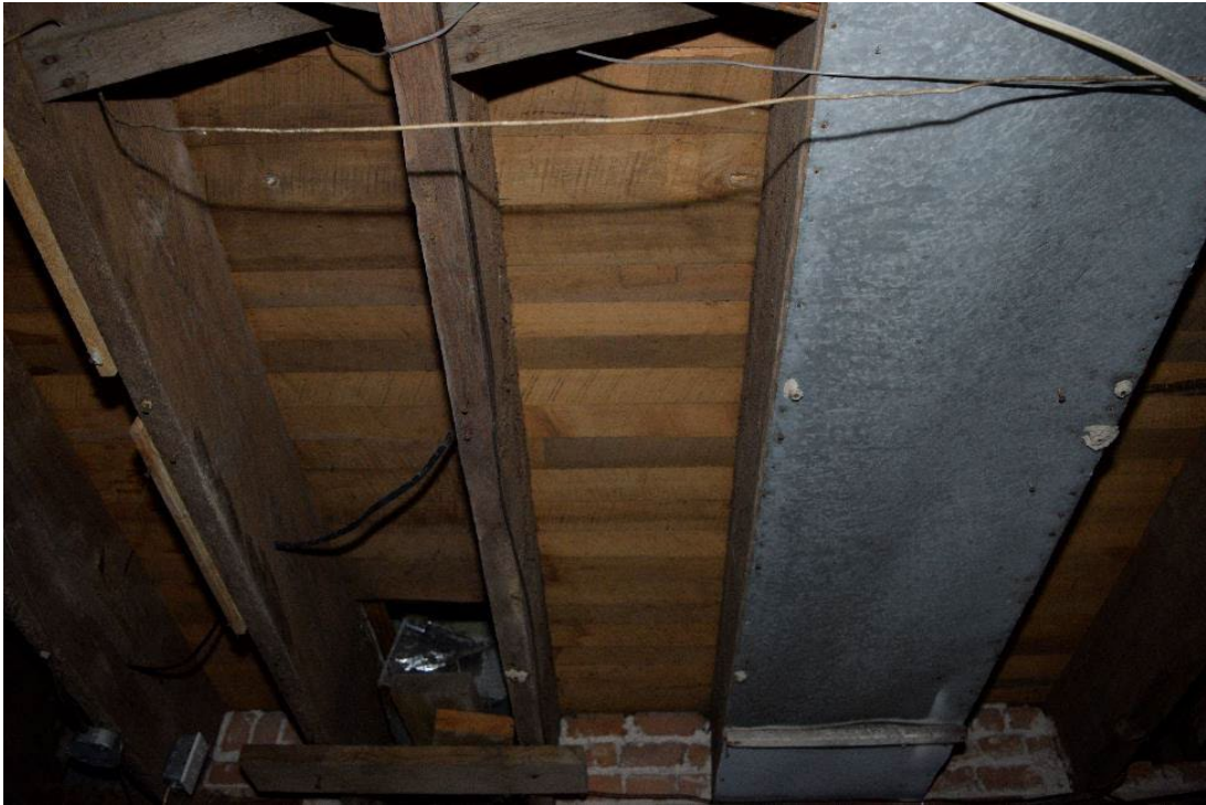
Figure 79: Typical joists with tongue and groove plank flooring
