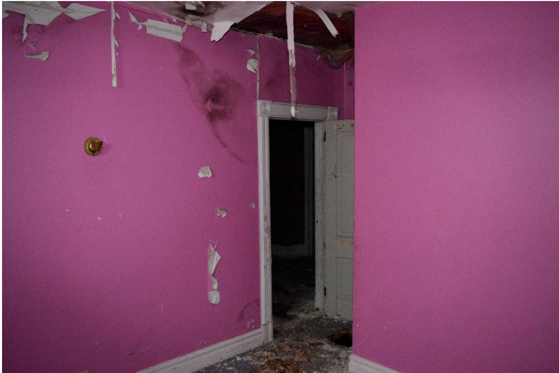
Figure 62: Northeast room second floor, facing southwest
