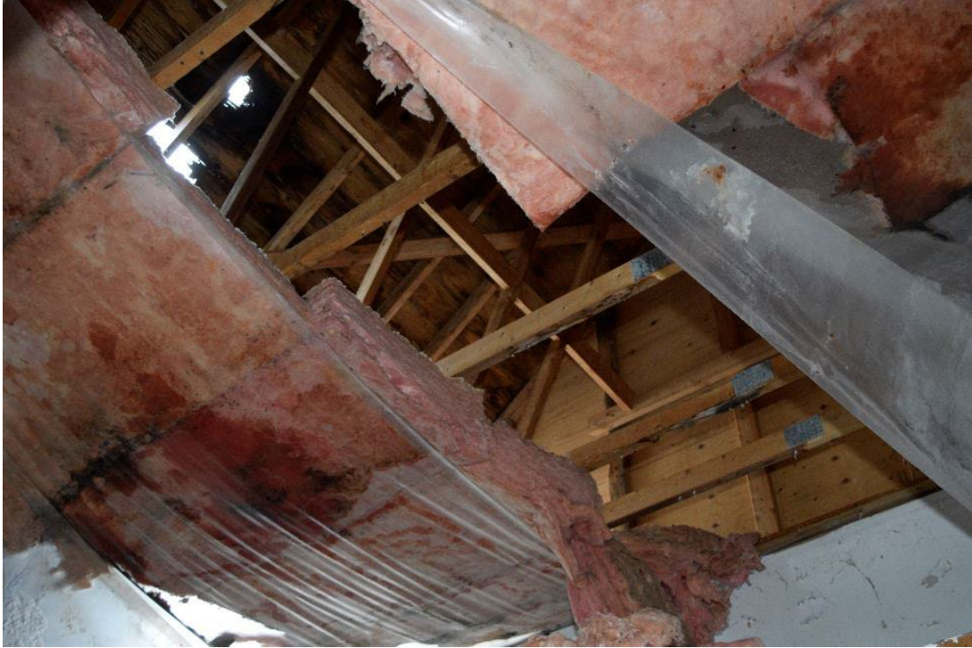
Figure 74: Modern trusses used in rear addition
