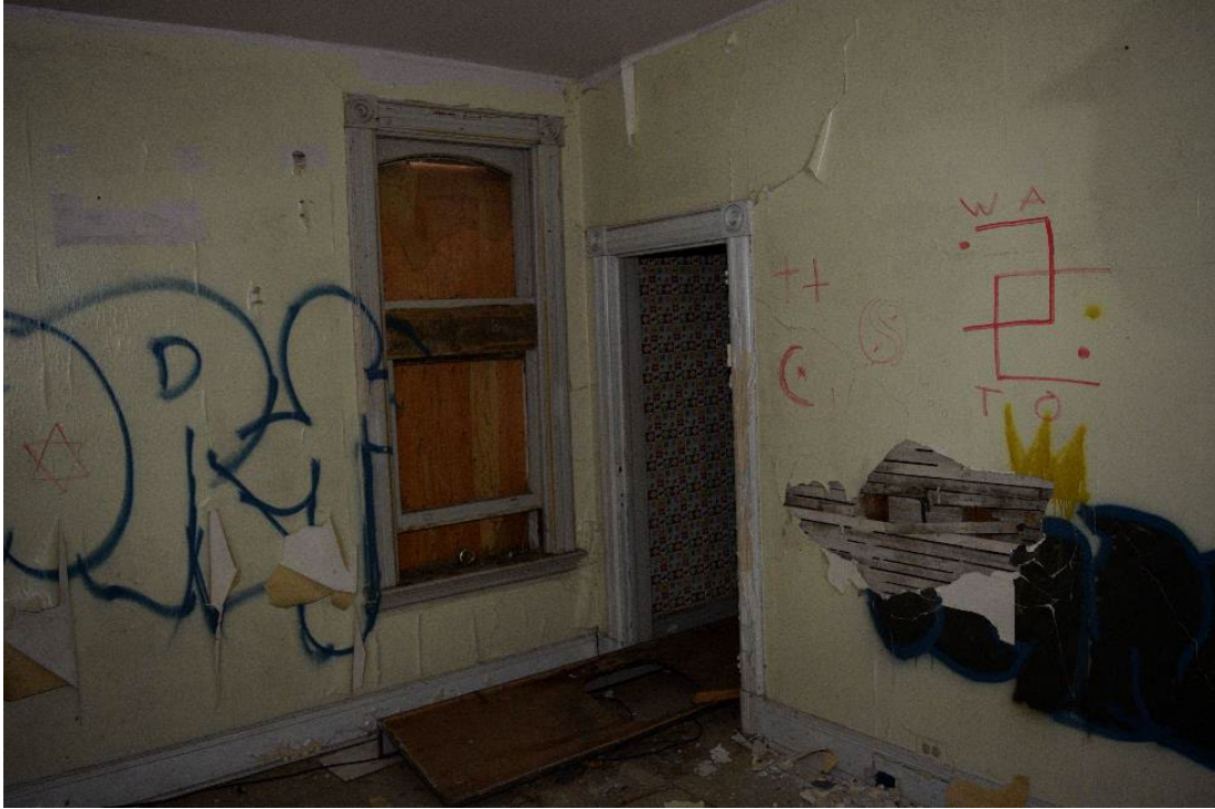
Figure 50: Central room on west side of structure, facing northwest
