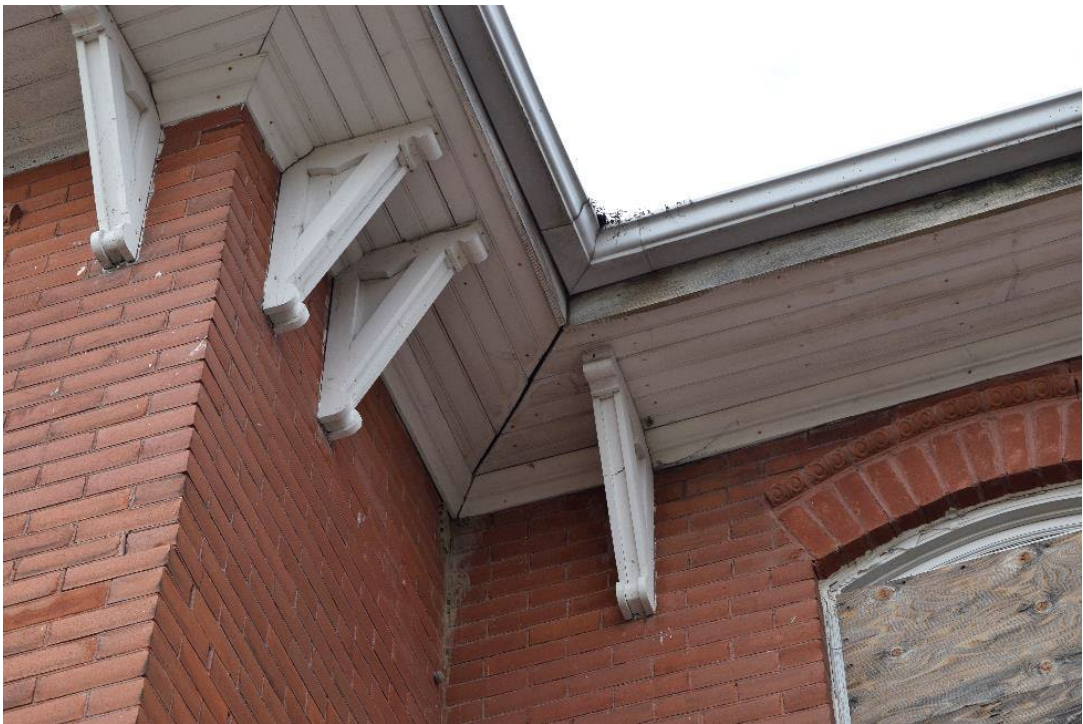
Figure 27: Decorative brackets used elsewhere on the structure, note the paired installation
