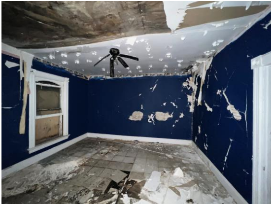
Picture 38: View of room on the second level, facing southeast.
