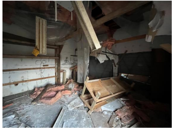
Picture 26: View of the inside of the garage, facing north.
