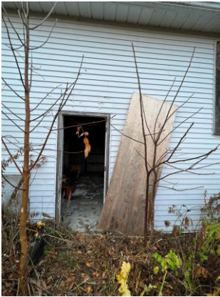
Picture 25: View of the garage door entrance, facing north.
