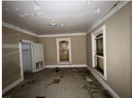
Picture 39: View of room on the second level, facing west
