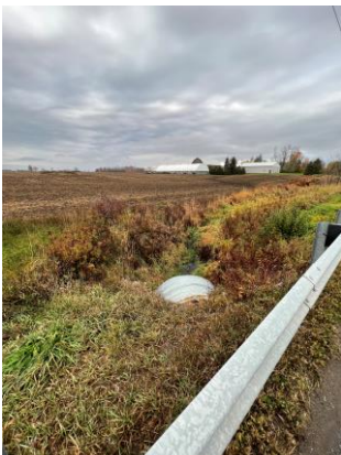
Picture 5: View of the culvert on the west adjacent property connecting it to the east side under the bridge for the tributary, facing northwest.
