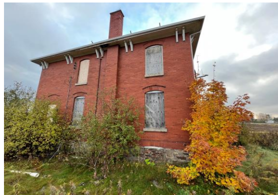
Picture 22: View of the old heritage situated on the central east portion of Phase One Property, facing south.
