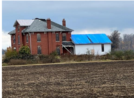
Picture 2: View of the Old Heritage home and the extended garage on the Phase One Property 12455 Creditview road), facing northeast.
