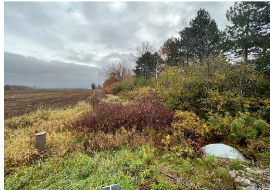
Picture 4: View of the culvert opening up in to the stream/creek on the southeast of the Site facing east.
