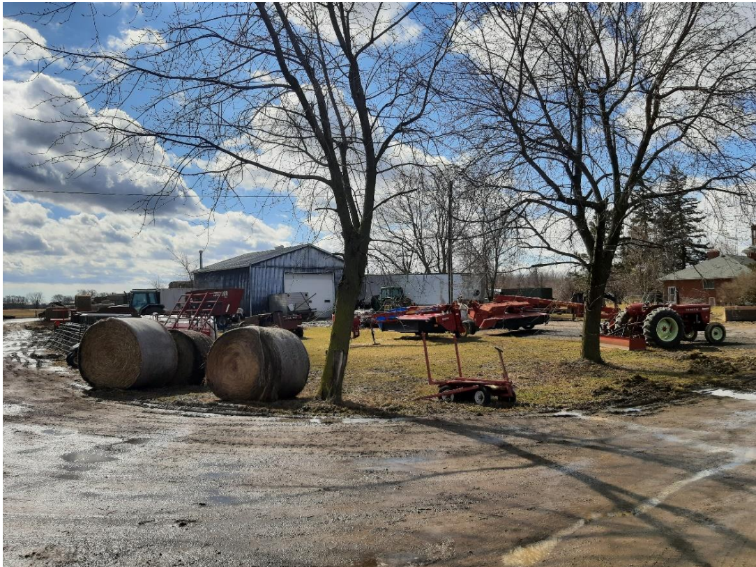
Photograph No. 6 – View of the farm equipment storage and the workshop building facing south.
