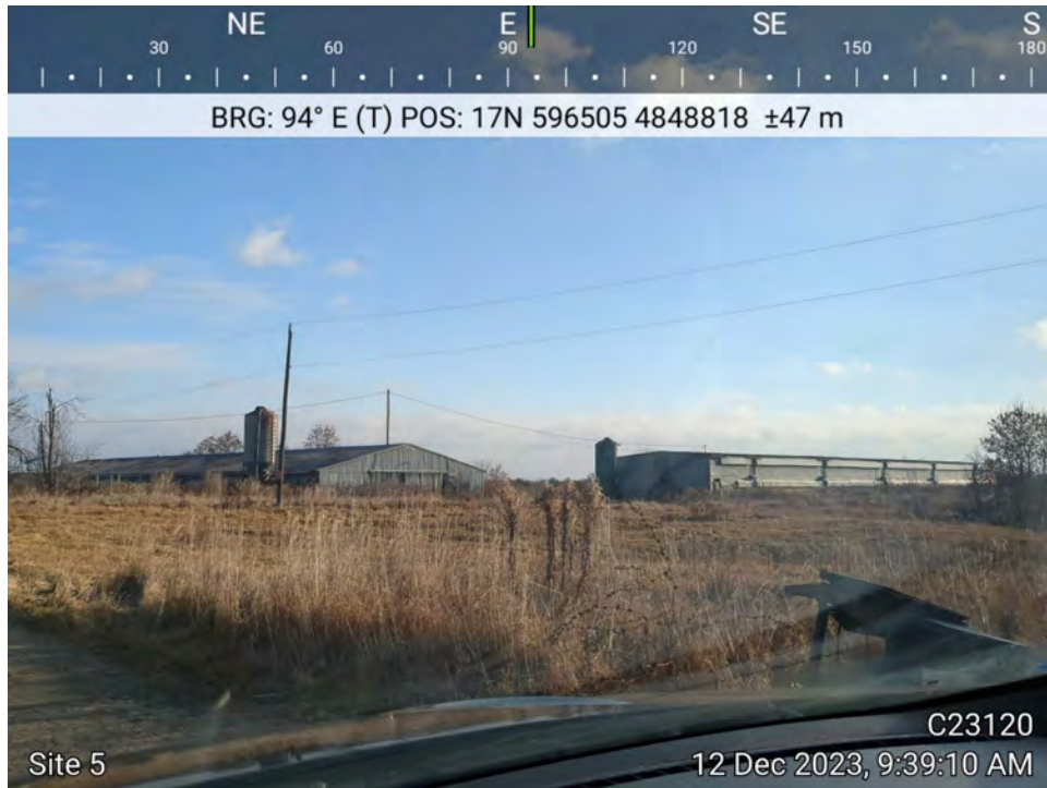
Photo 5: View of livestock housing at site #5, retired livestock operation.
