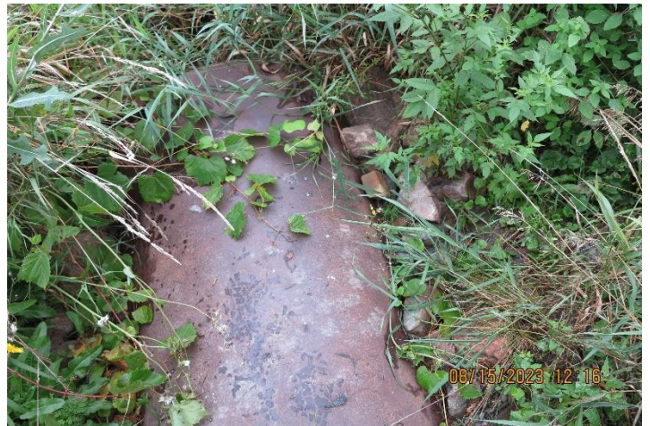
Photo 18: Steel pipe culvert in Kilamanagh Creek on 12861 Dixie Road. Date: August 15 2023
