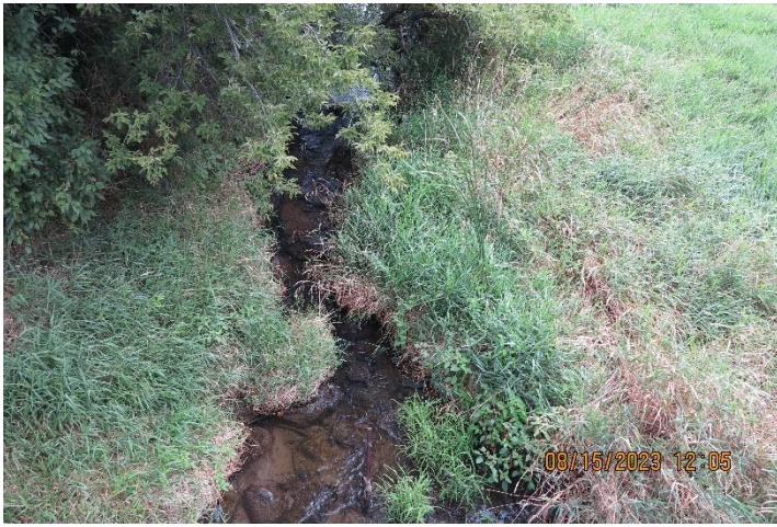
Photo 13: Conditions in Kilamanagh Creek on 12861 Dixie Road. Date: August 15 2023
