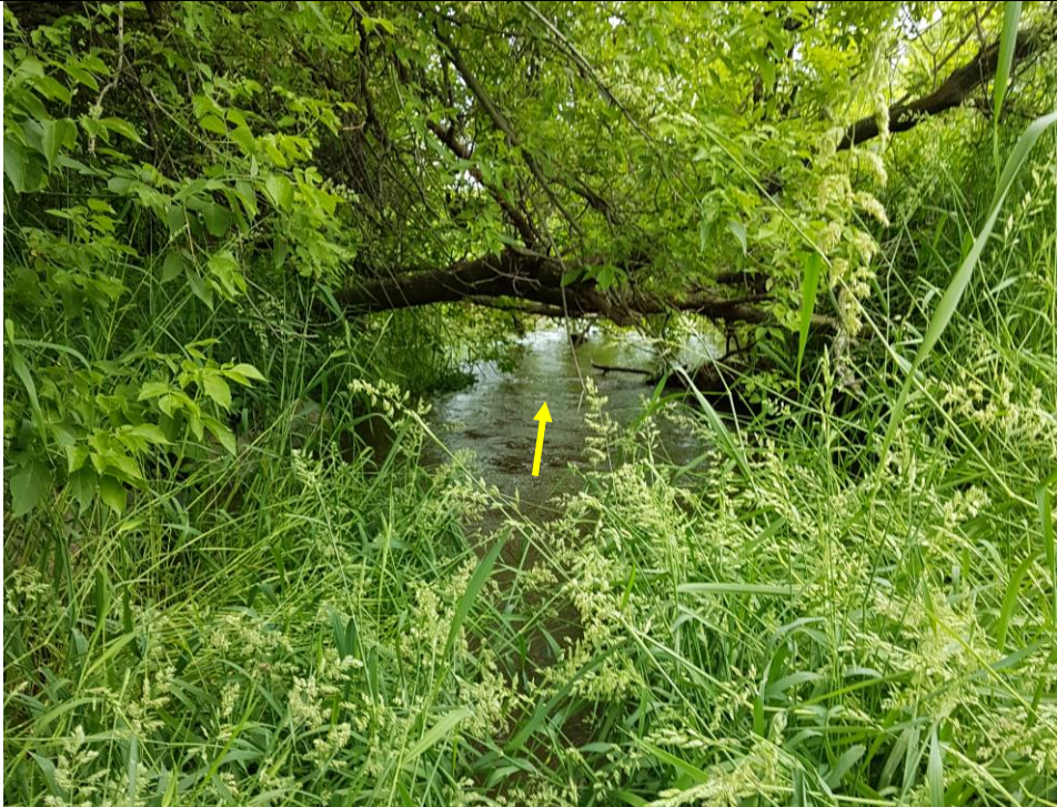
Photograph taken at the upstream extent of Reach 4b . The reach enters the subject property through a culvert along Dixie Road (yellow arrow indicates flow direction).
