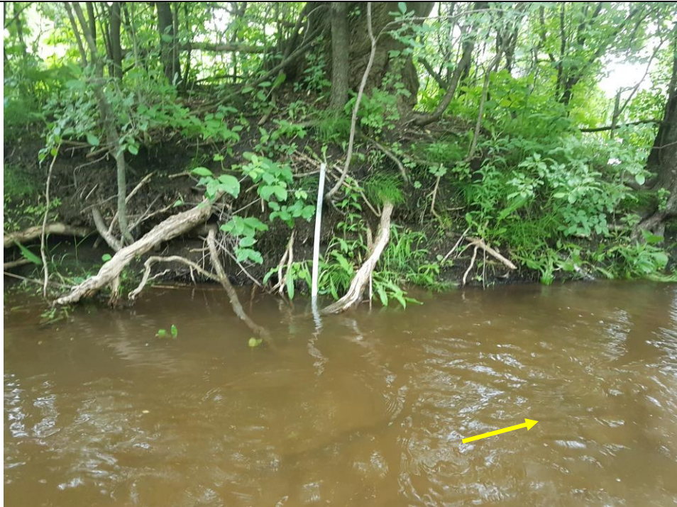
Bank erosion was observed throughout the channel as undercuts, basal scour, exposed tree roots, and fallen or leaning trees.
