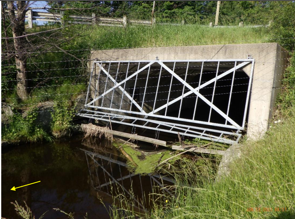
Photograph taken at the upstream extent of Reach 8a . The reach enters the subject property through a culvert along Dixie Road (yellow arrow indicates flow direction).
