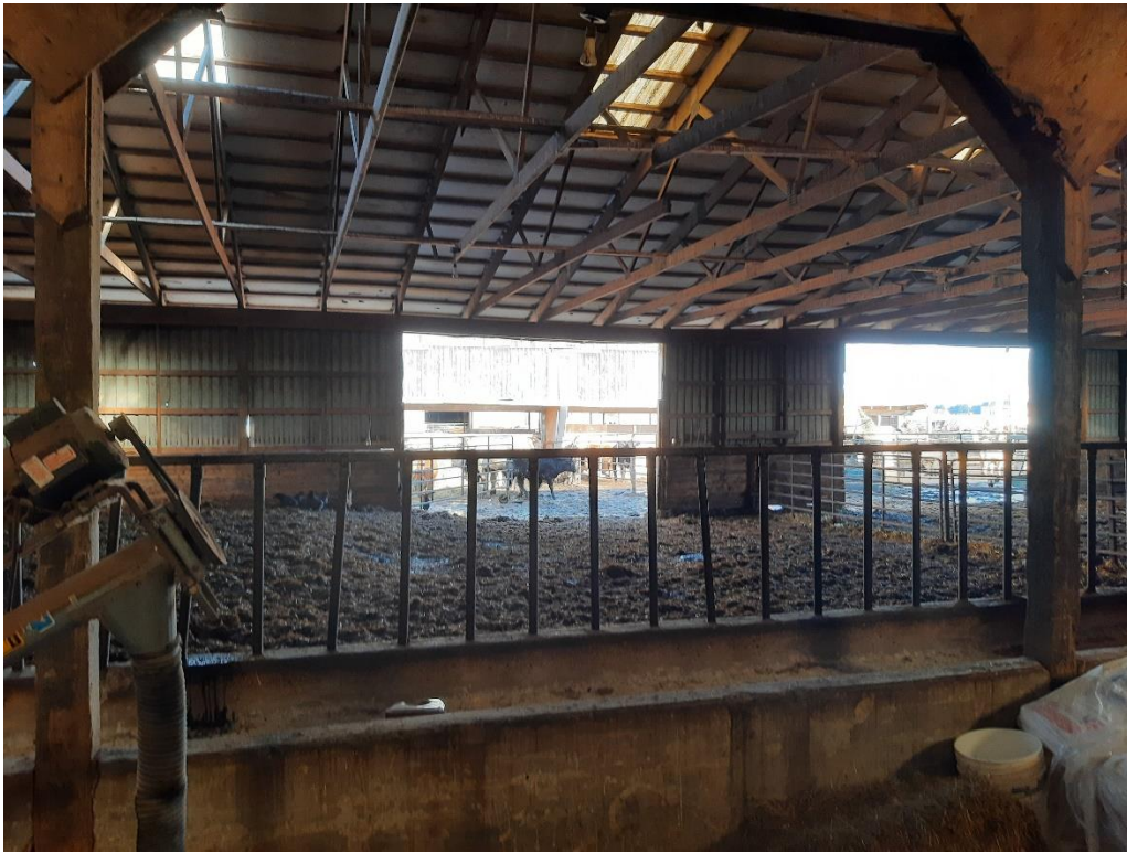
Photograph No. 9 – Interior view of the one-storey barn.
