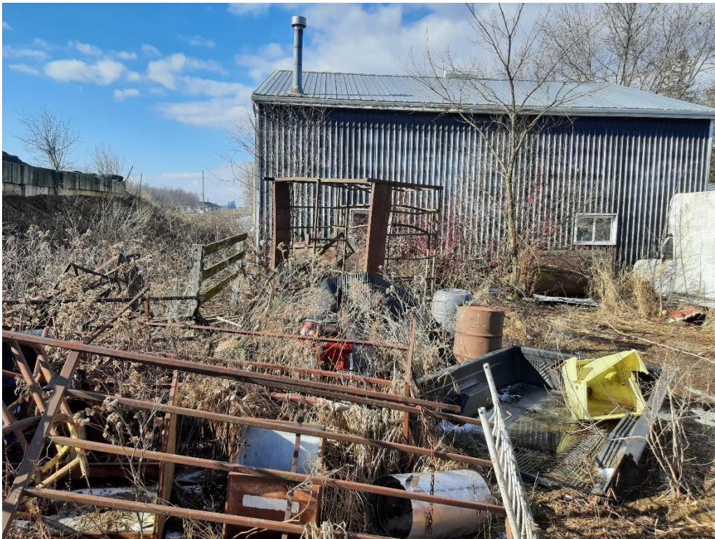
Photograph No. 6 – View of the workshop building facing west.
