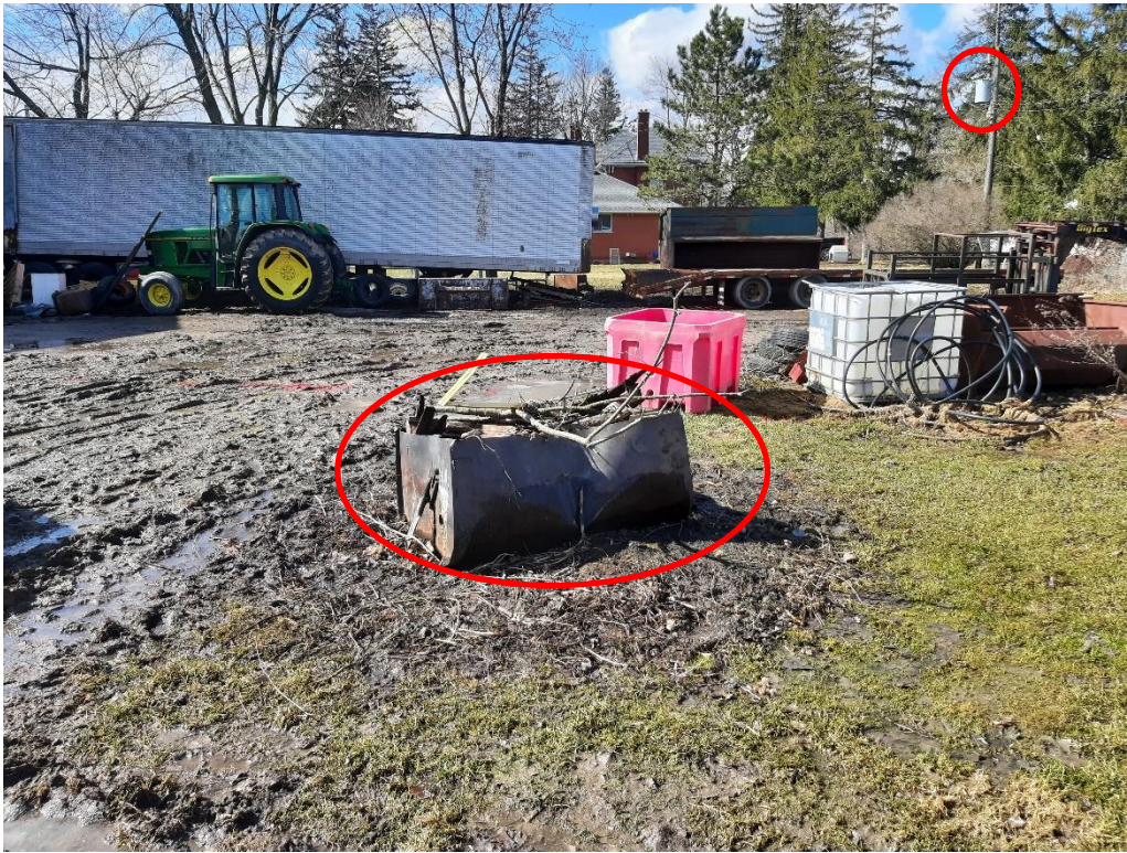
Photograph No. 15 – View of the fire pit in a half cut out steel barrel at the central portion of the Site and the pole mounted transformer, facing west.
