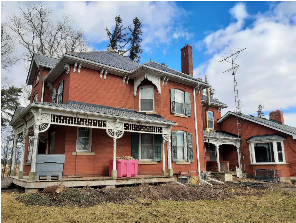
Photograph No. 2 – View of the farmhouse facing north.
