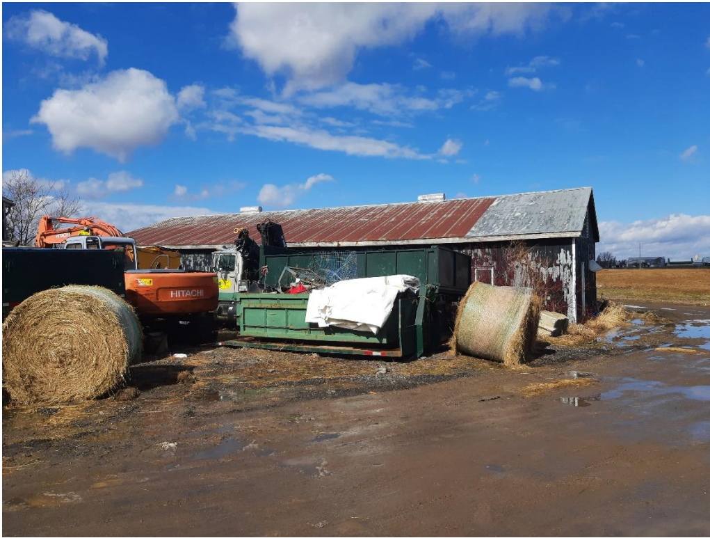
Photograph No. 13 – View of the miscellaneous scrap metal bin stored to the south of the north storage barn, facing north.
