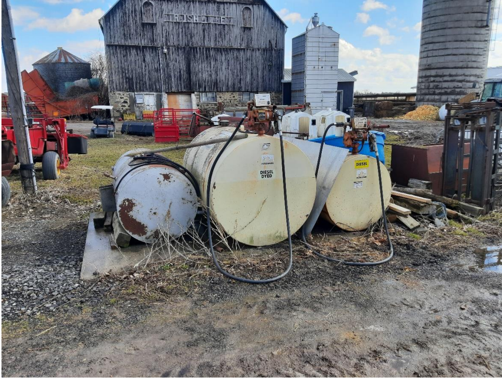
Photograph No. 17 – View of the 2,200L dyed diesel AST in use and two 1,360L dye diesel ASTs facing east from the gravel driveway.
