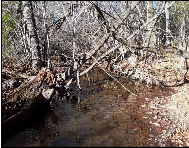
Photograph 21. Location 18. Reach WHT-2 North-South Tributary Downstream view of channel bank erosion. Note leaning trees and exposed tree roots on left bank. View: DS Date Taken: November 8, 2022 Site: 12522 & 12306 Torbram Rd, Caledon ON
