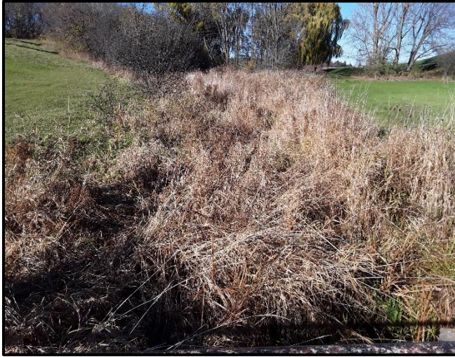
Photograph 29. Location 26. Reach WHT-3 North-South Tributary Upstream view of channel conditions from golf cart crossing. Note riparian grasses and vegetation encroachment. View: US Date Taken: November 8, 2022 Site: 12522 & 12306 Torbram Rd, Caledon ON
