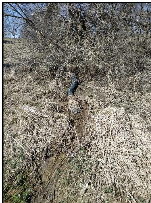
Photograph 11. HDF 3B – Upstream View of Tile Drain Outfall (April 12, 2023).
