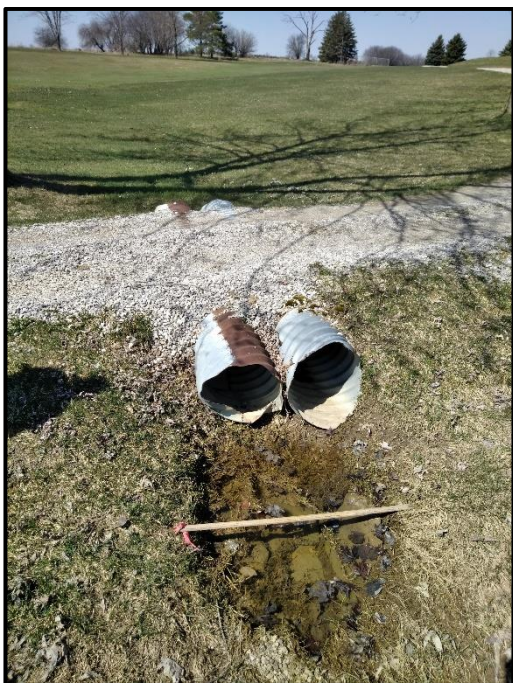
Photograph 14. HDF 4B – Upstream View (April 12, 2023).
