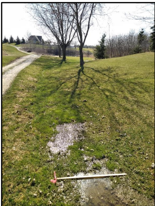
Photograph 8. HDF 1 – Downstream View (April 12, 2023).
