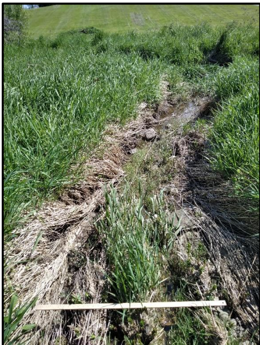
Photograph 12. HDF 3C – Downstream View (May 17, 2023).
