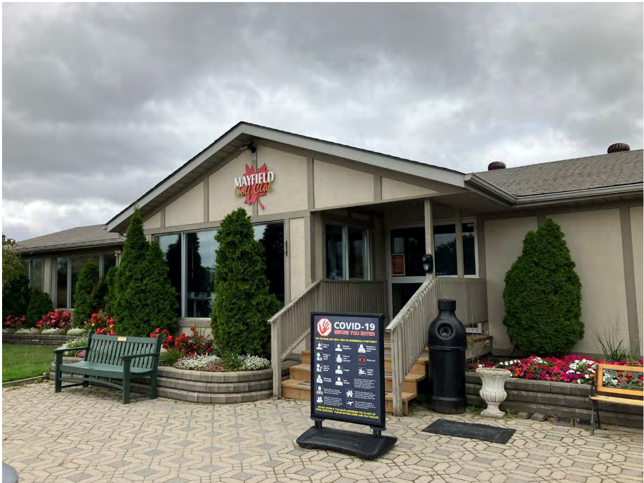
Photo H5 (South): Clubhouse entrance
