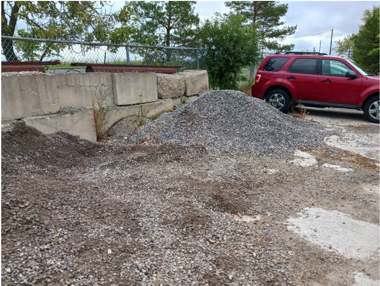
Photo H9 (North): Gravel stockpile
