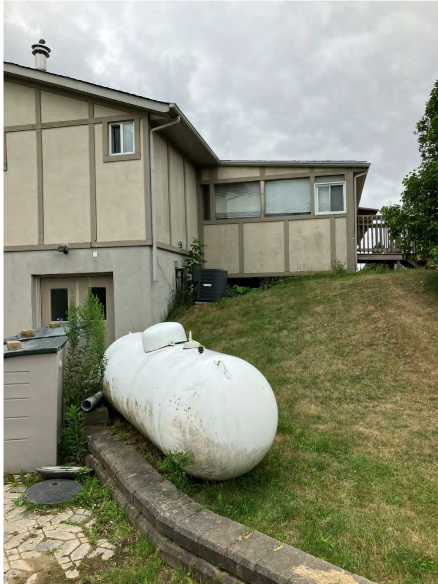
Photo H8 (East): 500-gallon propane AST at clubhouse
