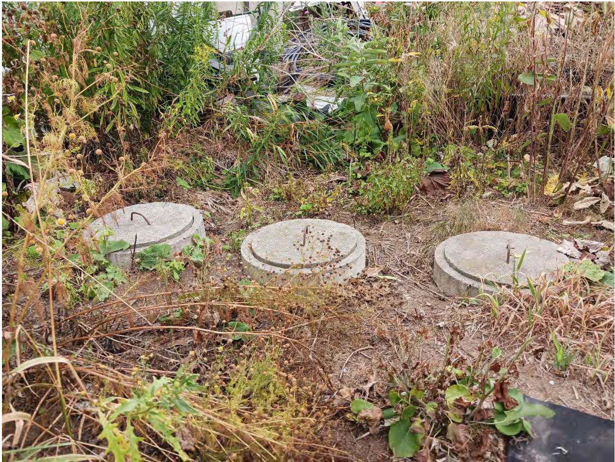
Photo H14 (West exterior of maintenance yard): Oil-water separator
