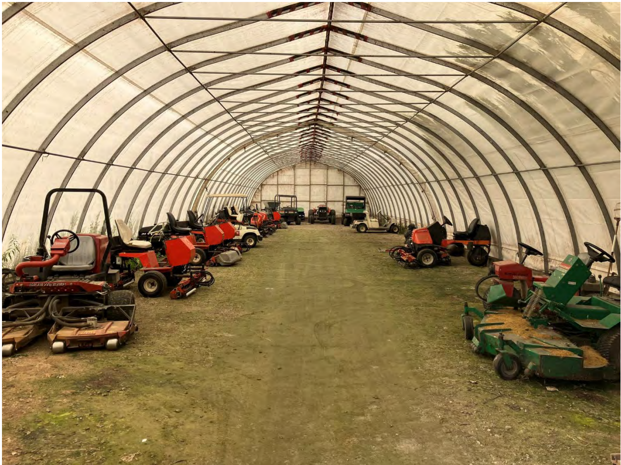
Photo H12 (Inside the vehicle storage shed): Carport structure used to store landscaping equipment
