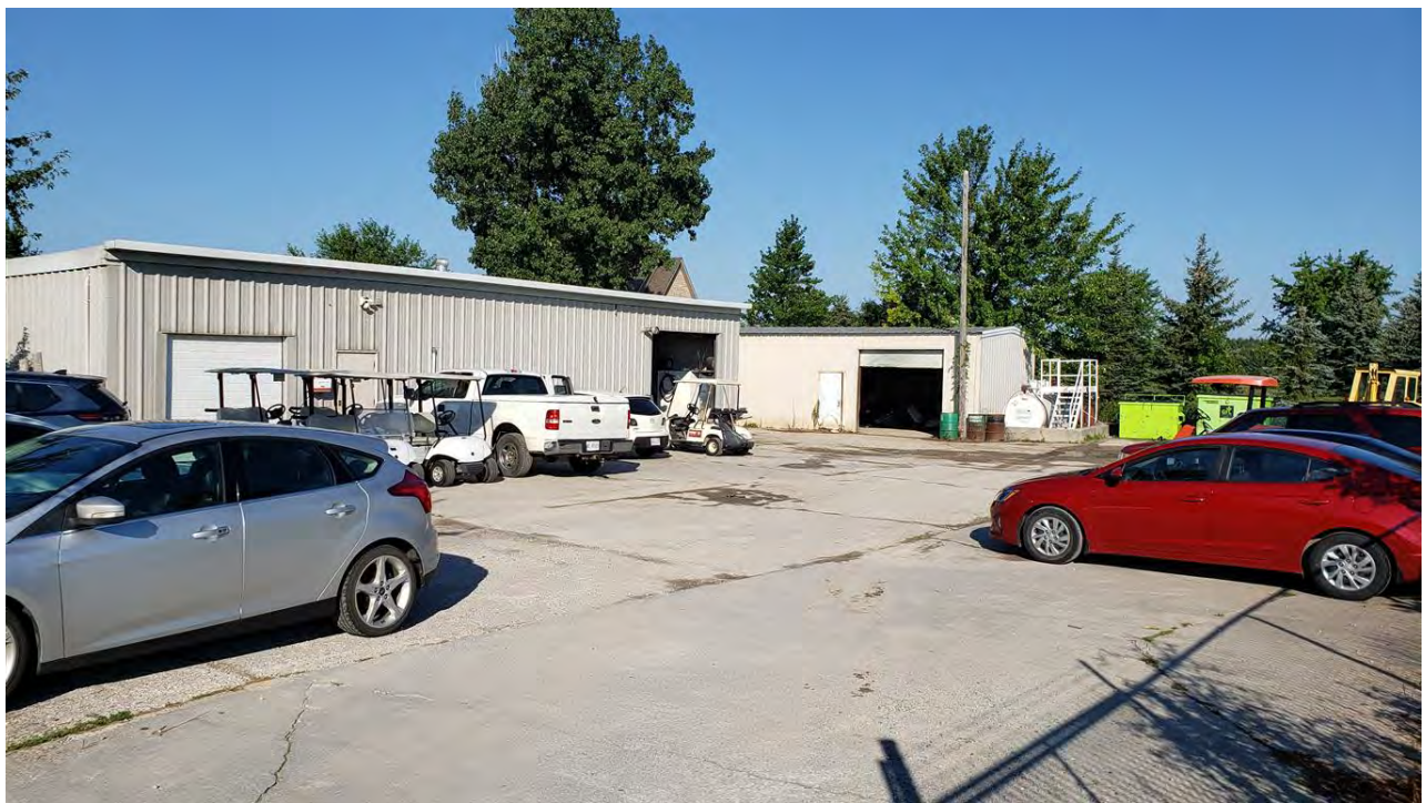
Image 16: Mayfield Golf Club maintenance facilities and their parking area; facing west, August 24, 2022.
