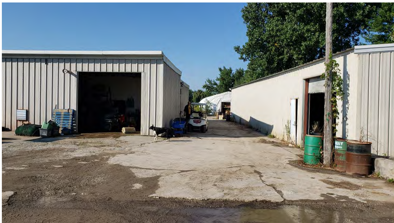
Image 17: Mayfield Golf Club maintenance facilities and their parking area; facing southwest, August 24, 2022.
