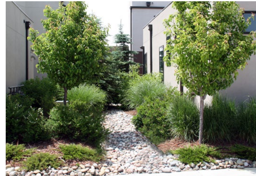
Roof downspouts help direct excess water into soakaway pits. Paired with xeriscape planting, the combination performs well in urban environments due to low-maintenance requirements
