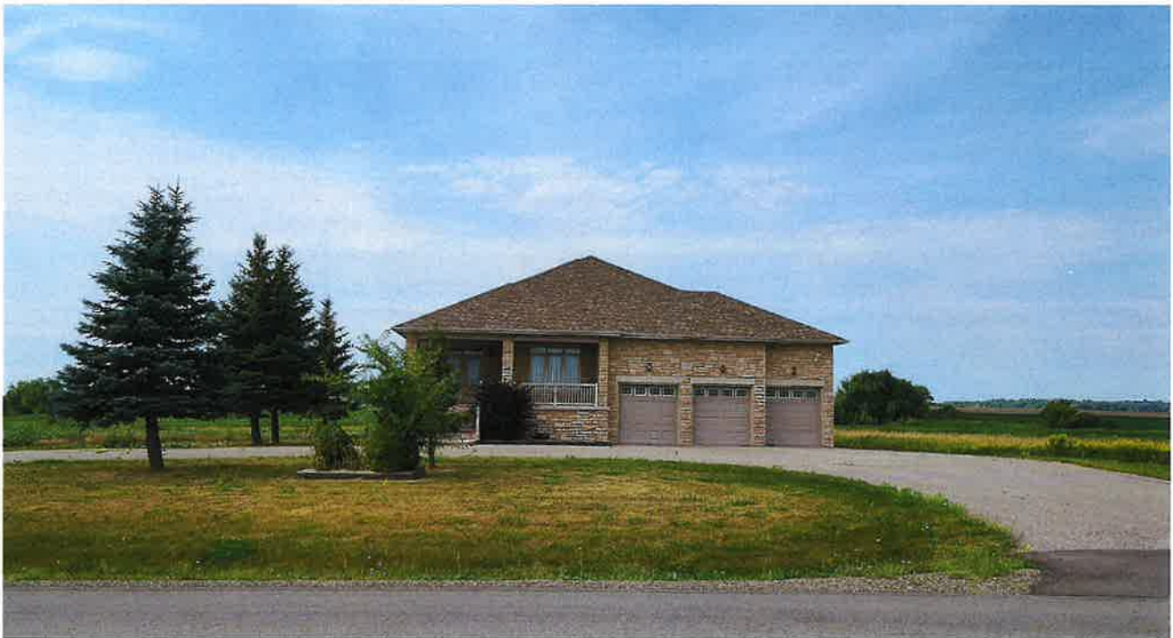
Neighboring property to the southwest of the subject site (looking west)
