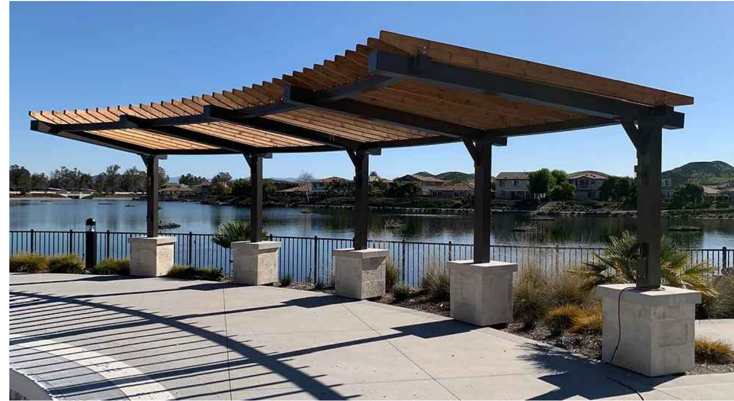
2 PARK LOOKOUT SHADE STRUCTURE
