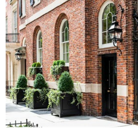
Windows should reflect the architectural style of the building
