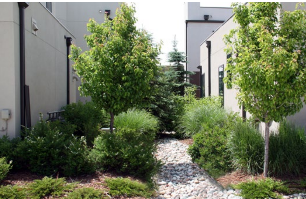
Roof downspouts help direct excess water into soakaway pits. Paired with xeriscape planting, the combination performs well in urban environments due to low-maintenance requirements.
