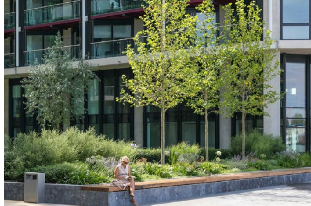
Rain gardens designed to capture water and allow it to infiltrate into the ground.
