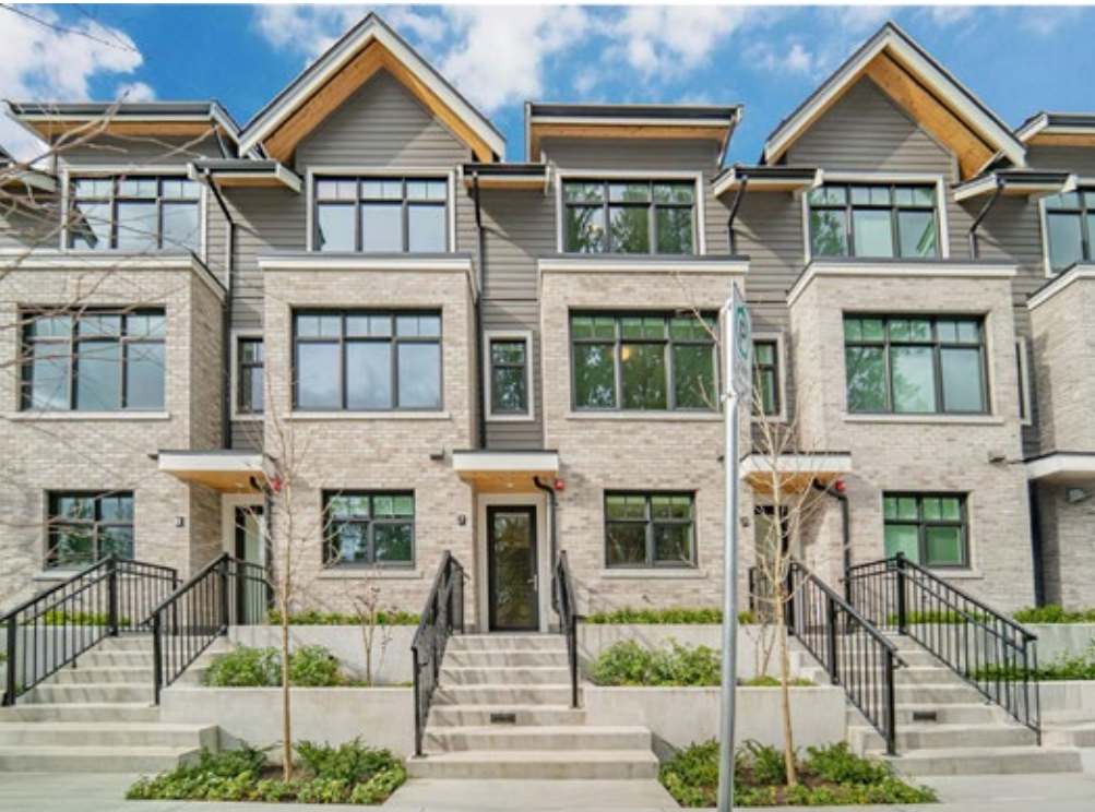
Building design should adapt to suit the site, especially when there are grading conditions to consider.
