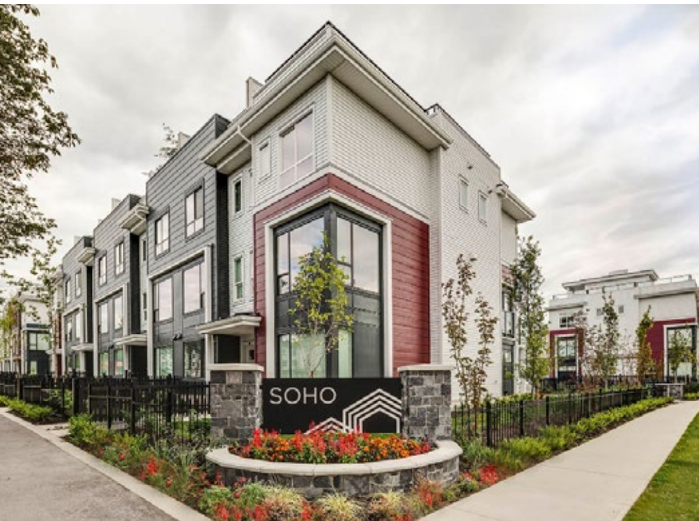
Associated hardscape and softscape landscape features may be integrated with built form massing to emphasize the gateway function.
