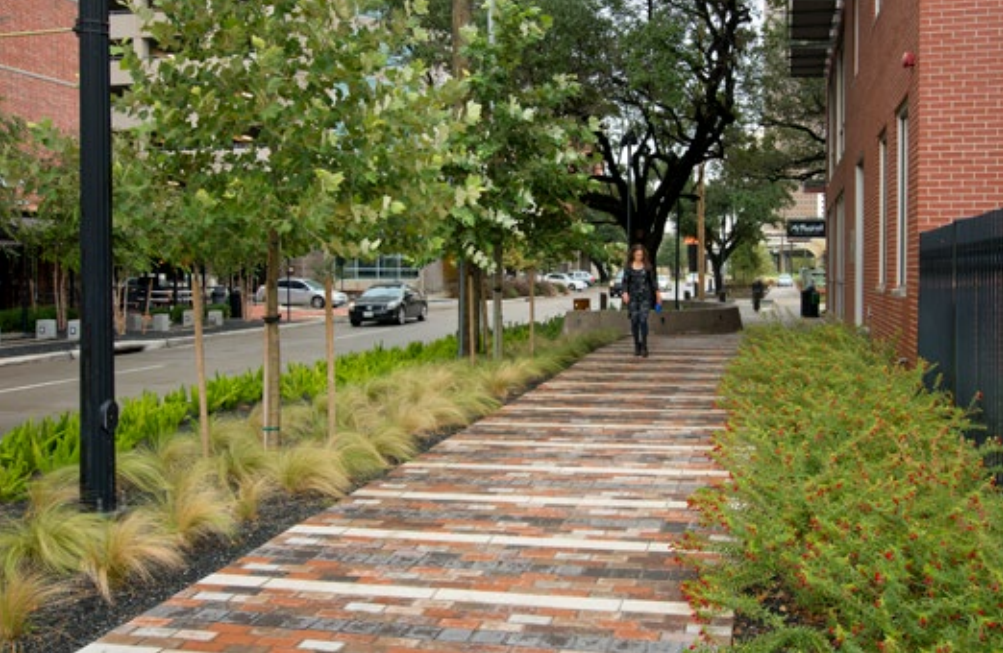
Drought tolerant planting species coupled with permeable paving help with rainfall and drainage.
