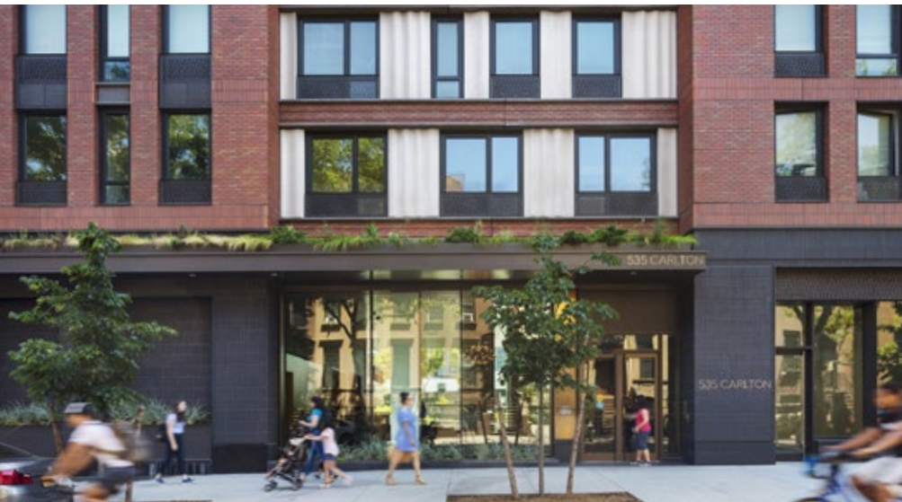
Transparent areas shall be maximized on the ground floor to allow views into the structure or into display windows.
