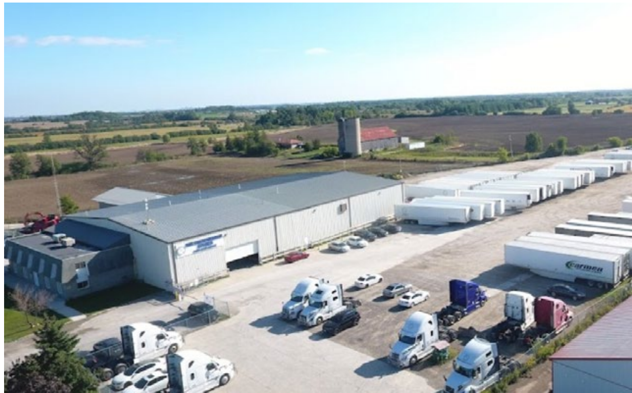
4 Sun Transportation Systems south of site along King Street
