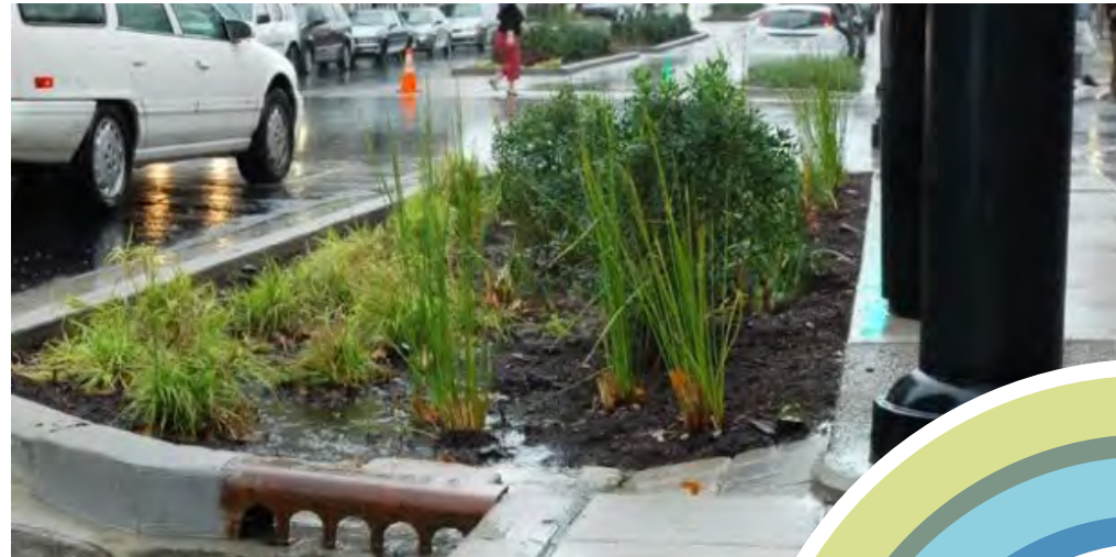
Street Level Stormwater Retention
