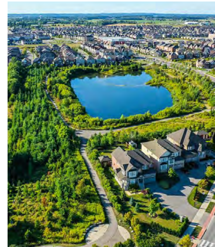
SWM ponds are a compatible use with the greenway system and have been situated along the edges of the community.
