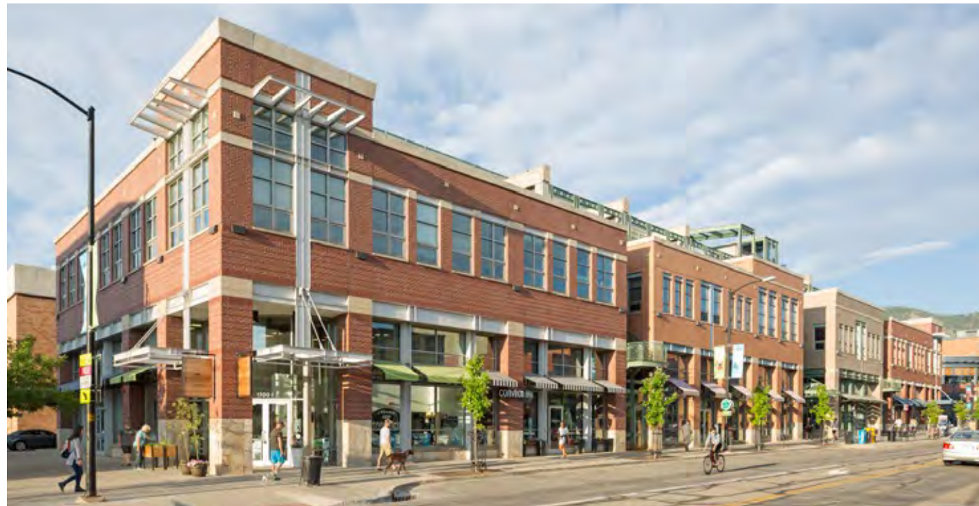
Example of parking facilities which have been architecturally designed to blend harmoniously with the surrounding buildings, enhancing the visual appeal along the streetscape.
