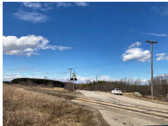
Plate 6: Humber Station Road facing northwest towards the Canadian Pacific Railway
