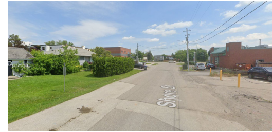
Figure 5: Existing Condition of Shore Street
