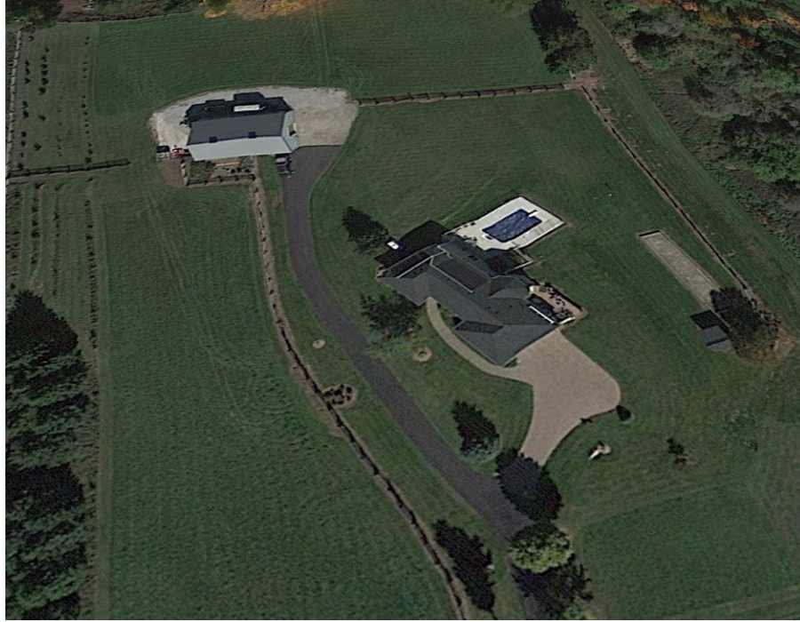
17673 Shaws Creek Road (Source: Google Earth)
