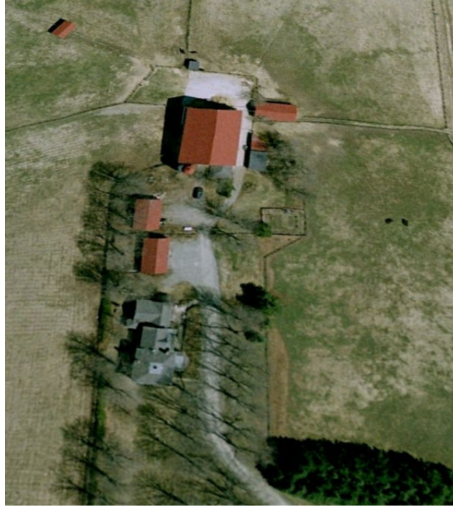
18101 Shaws Creek Road (Source: Google Earth)
