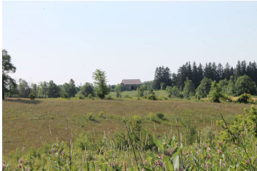
Bank barn, located at #17757, Shaws Creek Road (Photo taken from Elora Cataract Trail)
