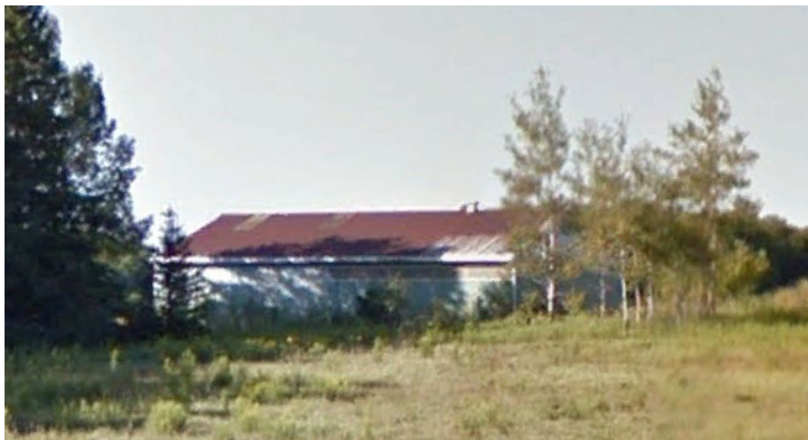
18147 Mississauga Road (Source: Google Earth)
