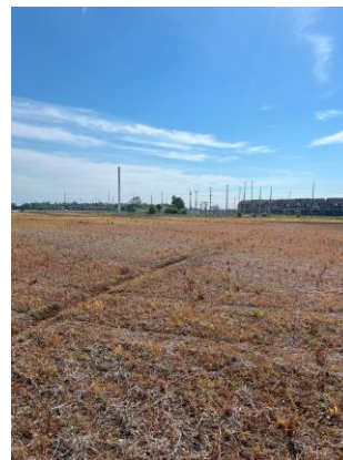
Picture 12: View of electrical transformers (east neighbouring property), facing west.
