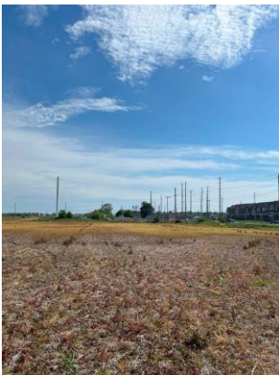
Picture 15: A closer view of electrical transformers on the east neighbouring property, facing west.
