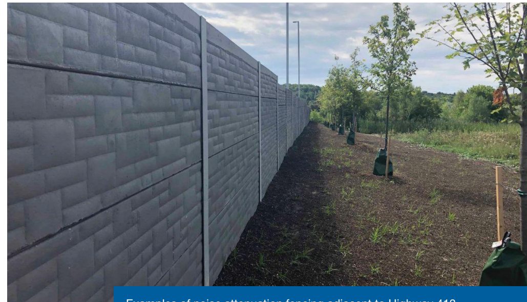
Examples of noise attenuation fencing adjacent to Highway 413
