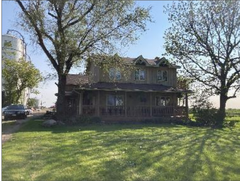
Photo 1 – Site Building A (southwest side).
