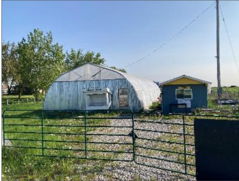
Photo 9 – Site Building K and L (southwest side).
