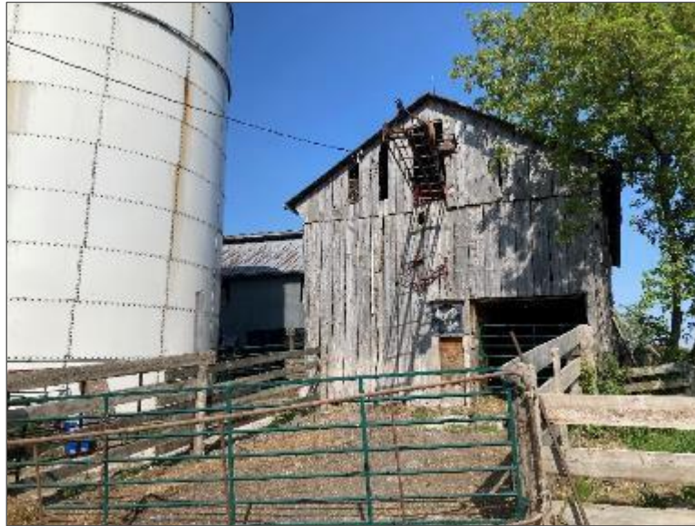
Photo 5 – Site Building E and F (southeast side).
