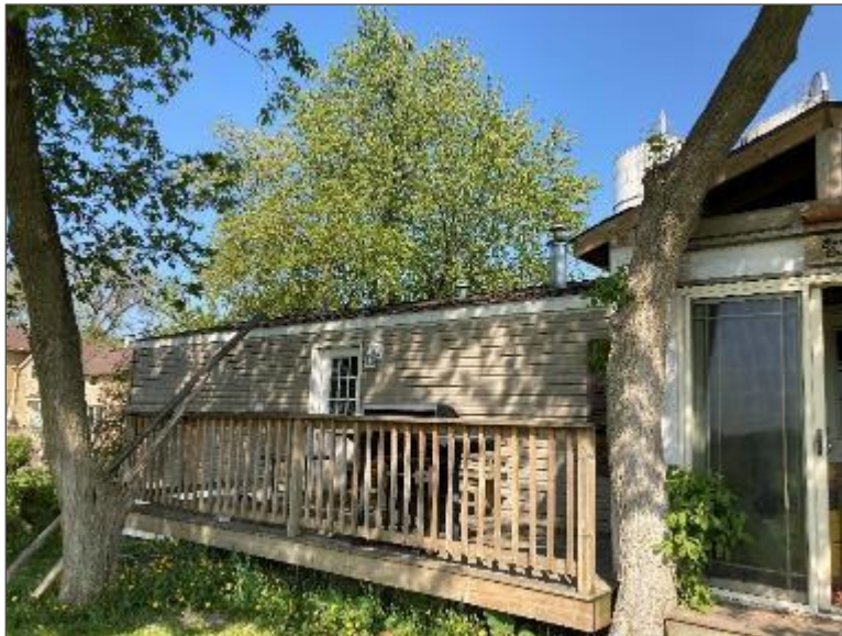
Photo 2 – Site Building B (southeast side).
