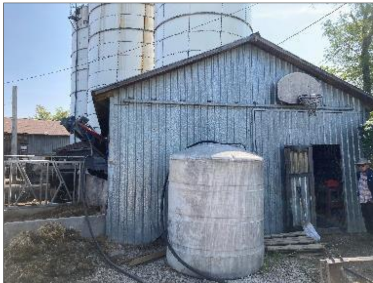
Photo 6 – Site Building G (southwest side).
