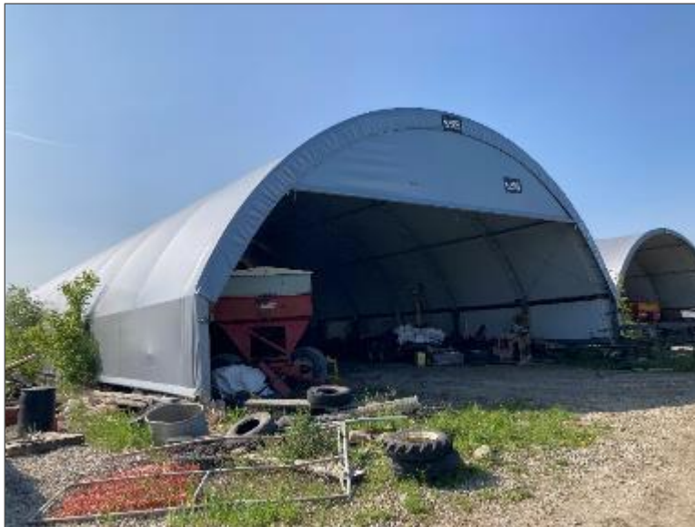
Photo 8 – Site Buildings I and J (northwest side).
