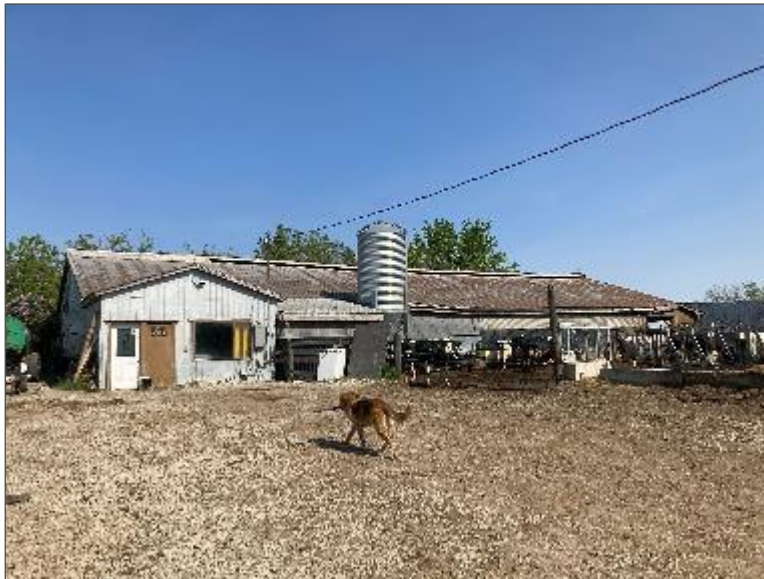
Photo 4 – Site Building (southeast side).
