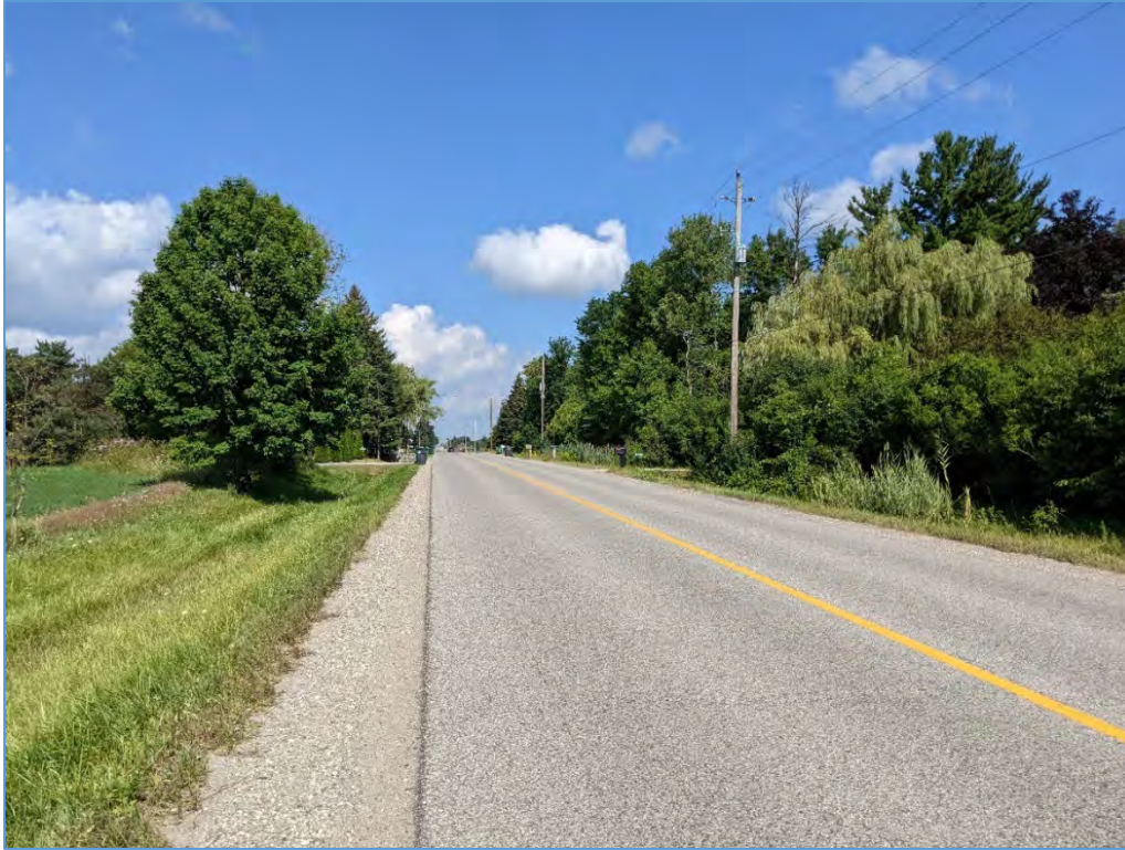
Figure 29: View north on Innis Lake Road
