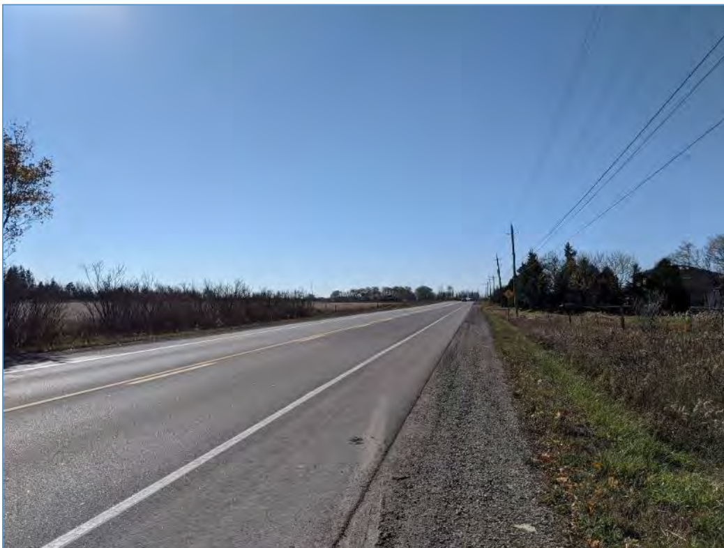
Figure 16: View west on King Street
