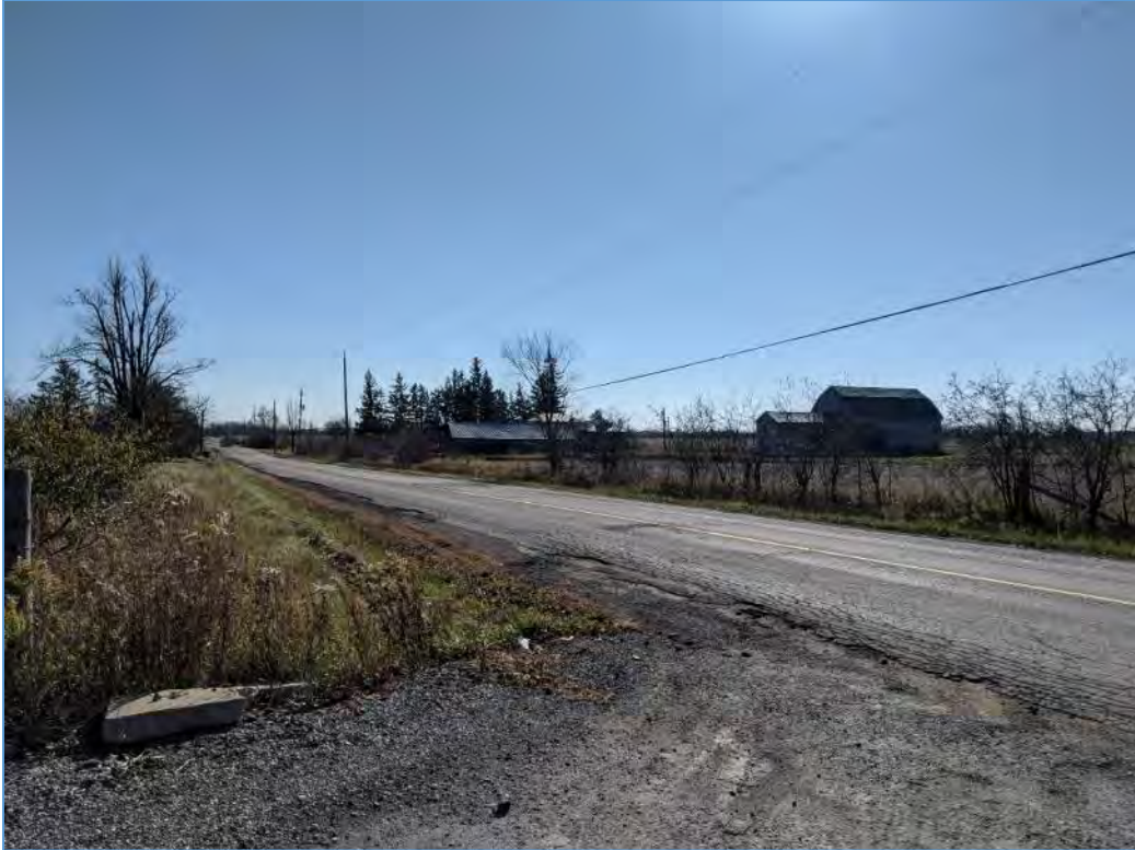
Figure 19: View south of 14166 Centreville Creek Road
