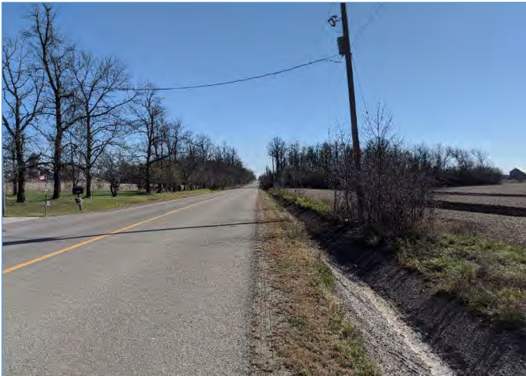
Figure 12: View south on Centreville Creek Road
