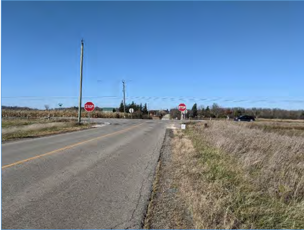
Figure 17: View north, intersection of King Street and Centreville Creek Road
