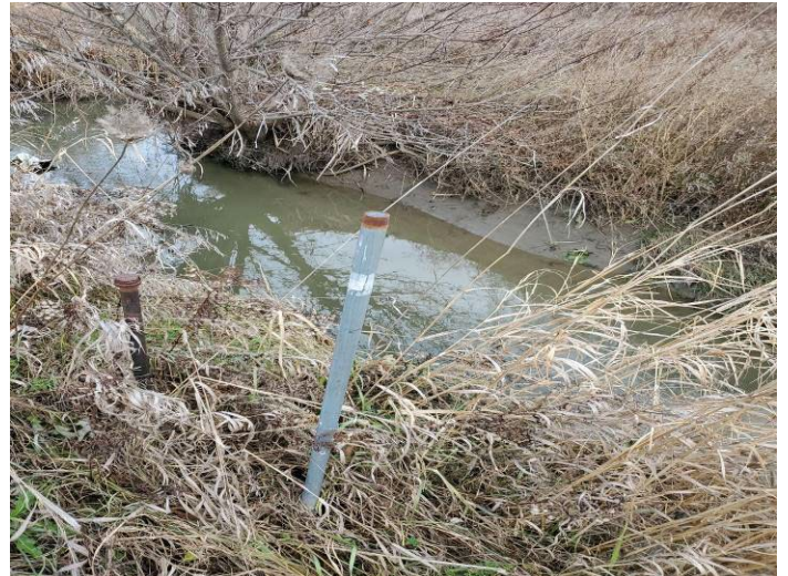
Photo 16: A view of the piezometers at SF6-17 taken on December 9, 2022. A missing cap was observed on one of them, but remaining conditions were noted to be in good condition.
