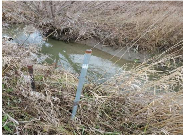
Photo 16: A view of the piezometers at SF6-17 taken on December 9, 2022. A missing cap was observed on one of them, but remaining conditions were noted to be in good condition.
