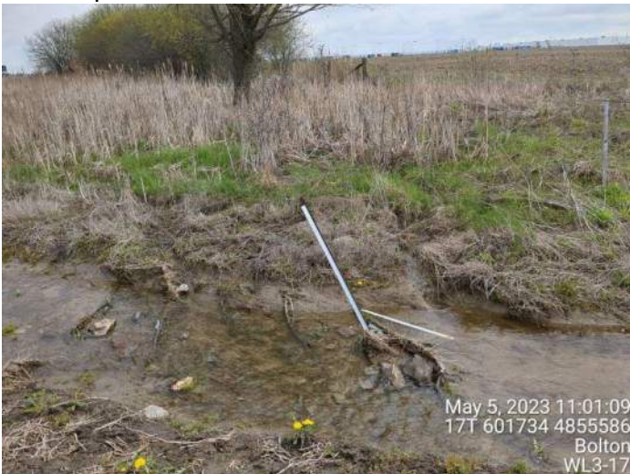
Photo 41: A view of the wetland station at WL3-17 taken on May 5, 2023. No piezometers were observed in the vicinity. Staff gauge is observed to be in poor condition. Stream flow was observed from slow to intermediate.
