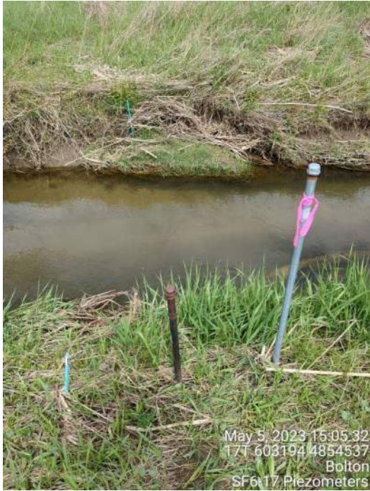
Photo 17: A view of the piezometers at streamflow station SF6-17 taken on May 5, 2023. A replacement cap was provided. Piezometer conditions were noted to be in good condition.
