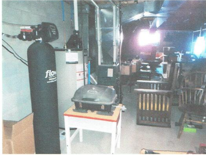
Photo No. 7: Basement
