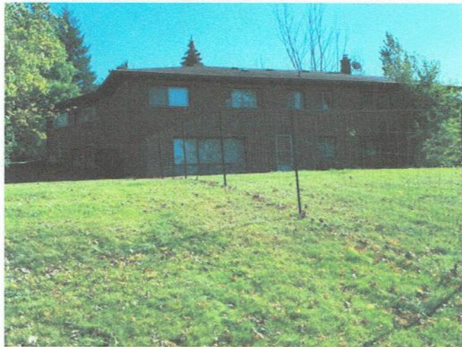
Photo No. 3: Backyard (probable Septic Tile Bed)
