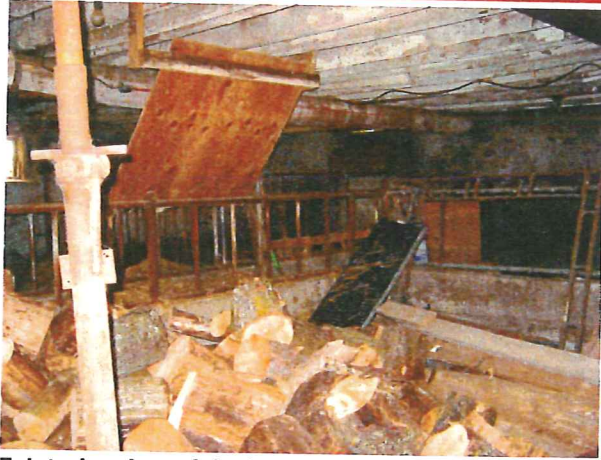
7. Interior view of the barn facing northwest.
