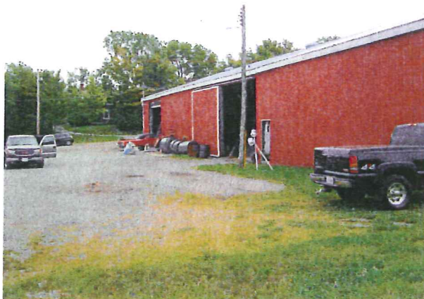
5. View of the diesel ASTs located on the phase one property (facing south).
