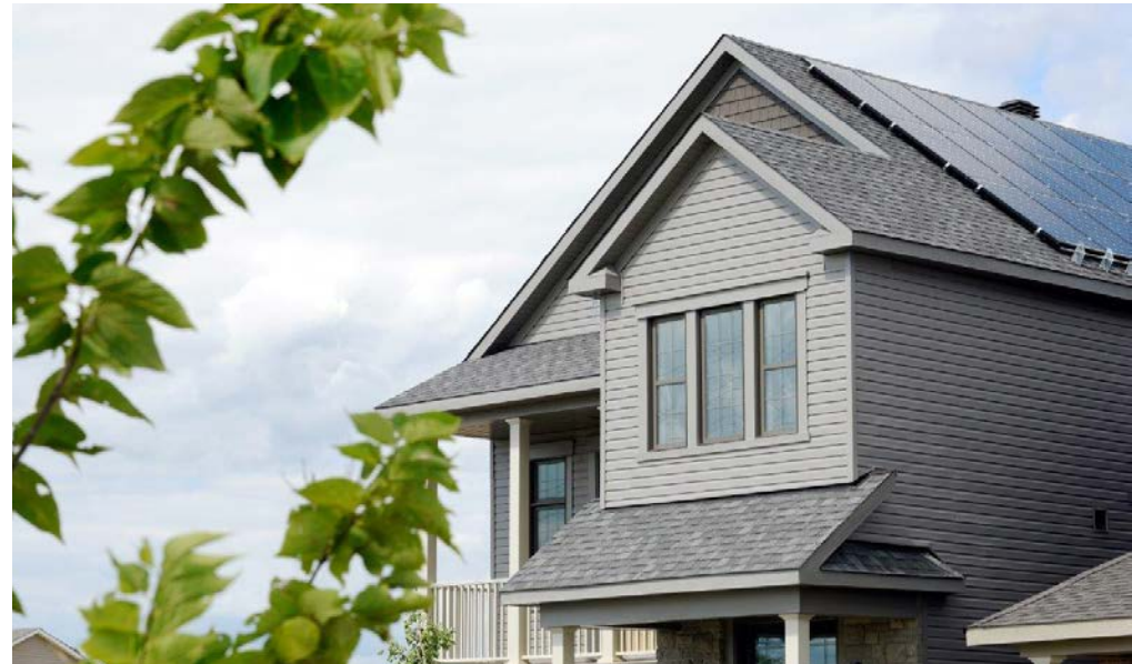
Solar paneling located on residential roofs can provide an alternative and sustainable energy source
