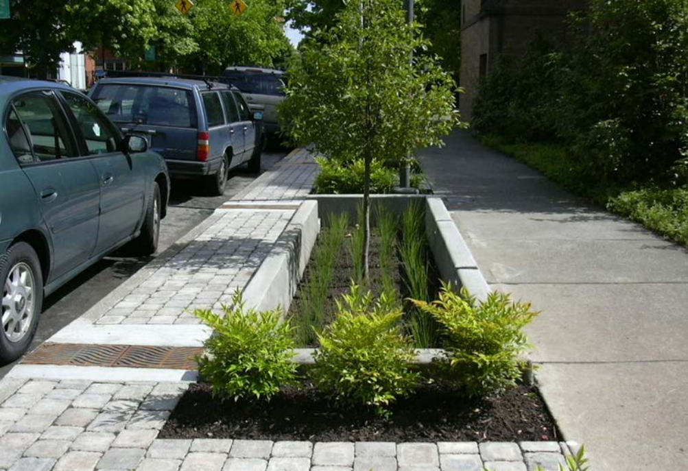
Street level stormwater retention
